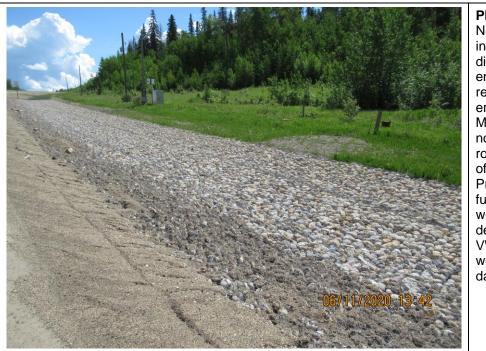
Photo 42-05. New gabion mattress installed in the south ditch across the entire site extents to repair previous erosion damage. Minor rill erosion was noted between the road edge and edge of the gabion. Previous non-functioning pumping wells were decommissioned and VW piezometers were added with a datalogger.
