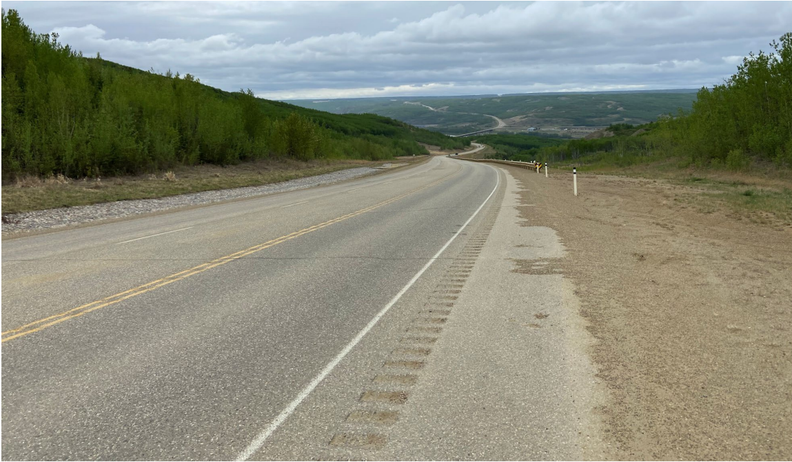
Photo 42-03.: Looking west at the replaced highway segment that previously had cracking and settlement across the roadway due to landslide movement (33+300). Road surface was in a good condition at time of inspection and had no observable change from the 2023 condition.
