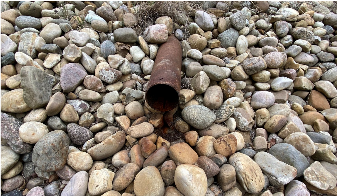
Photo 42-04.: Looking at subdrain pipe outlet that was slowly dripping within the end of the armoured drainage swale from the west side of the wall.
