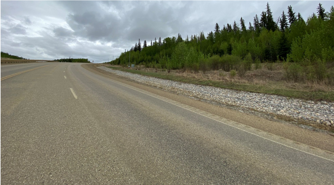
Photo 42-05.: View looking east at the gabion mattress installed in the south ditch across the entire site extents to repair previous erosion damage. Minor rill erosion was noted between the road edge and edge of the gabion. No major visible changes within the area east of 33+175 since 2023.
