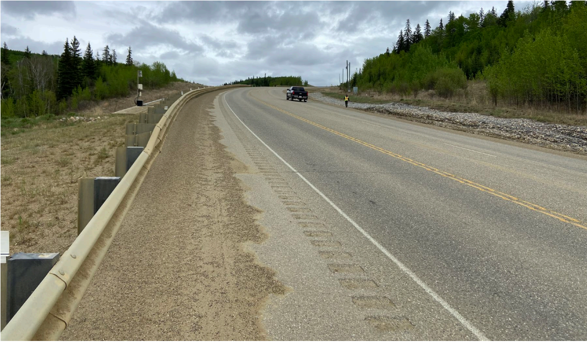
Photo 42-01.: Looking east across the repaired slide area. Guardrail and pavement surface in good condition with no major change since previous inspection.
