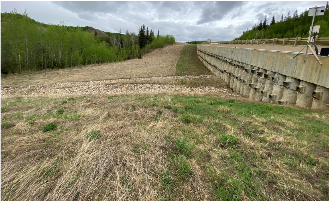
Photo 42-02.: Looking east at the pile wall and regraded slope below. Wall appears in a good condition and there has been no observable changes in the slope below since 2023.
