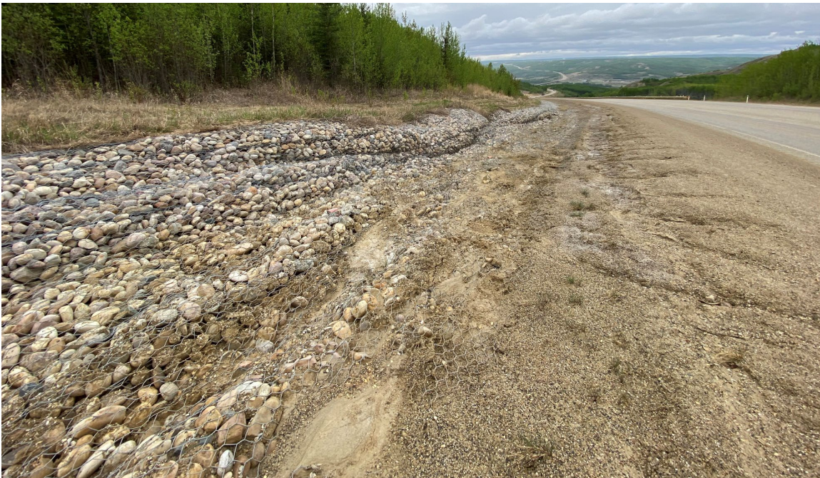
Photo 42-06.: Looking west at the gabion mattress installed in the south ditch near 33+125 deformed by the toe roll of an upslope landslide that occurred in 2020. Gabion was slightly more heaved but had no significant change since previous inspection. Some increased erosion in ditch sideslope due to restricted flow from gabion heave.
