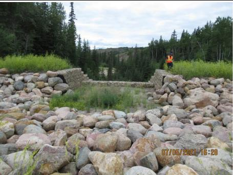
Photo 43-18. View of the riprap berm located near the top of the gabion drop structure (33+650)
