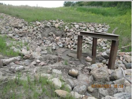
Photo 43-14. Site B culvert inlet with riprap protection and steel H-beam debris deflector. Inlet become severely damaged and blocked with fallen riprap during a high flow event in 2019/2020 (33+800). Repairs required in this area.
