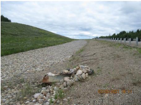
Photo 43-10. Looking east towards the north ditch gabion mattress installation at Site B (34+00).
