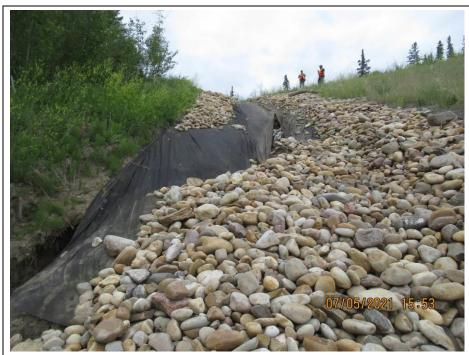
Photo 43-13. Looking south, upslope towards washed out riprap and extensive erosion damage within the riprap swale at the east side of Site A (33+500), likely the result of a high-flow event.
