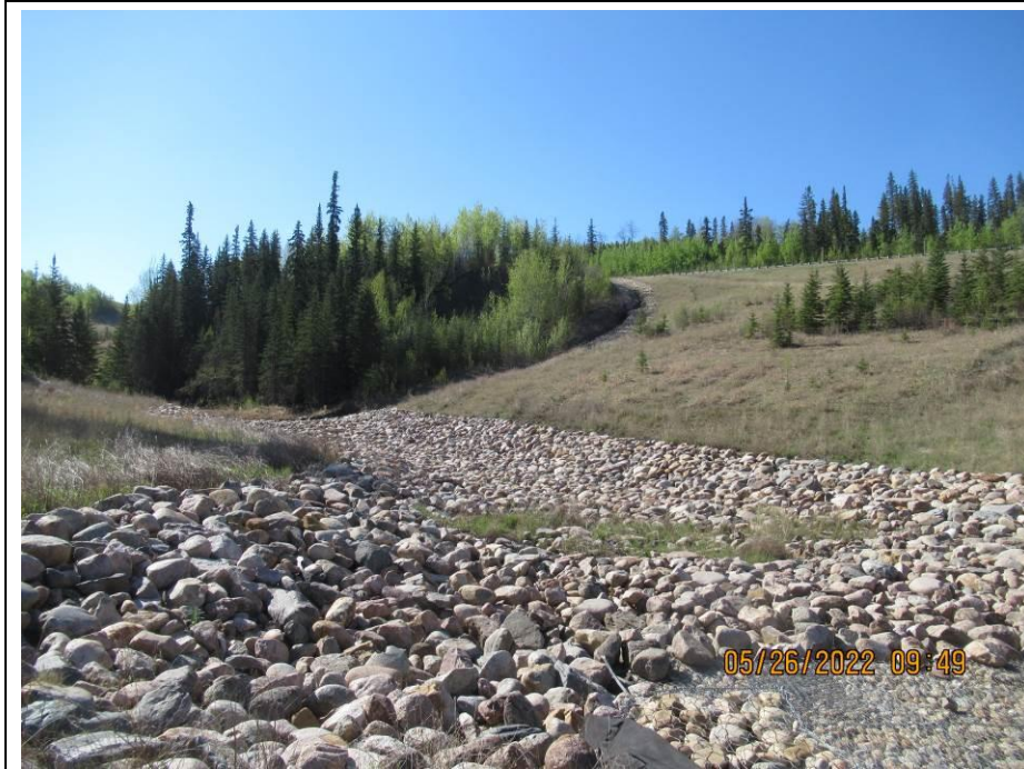
Photo 43-05. Standing at the top of the gabion drop structure looking east towards the overflow channel riprap (33+450). Vegetation has re-established.
