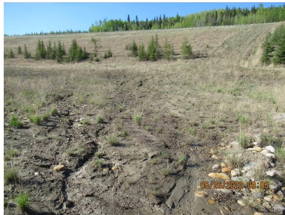
Photo 43-07. Looking south towards the Site B highway embankment and overland flow area. Minor rill erosion is visible on the right top corner of the photo along the slope.
