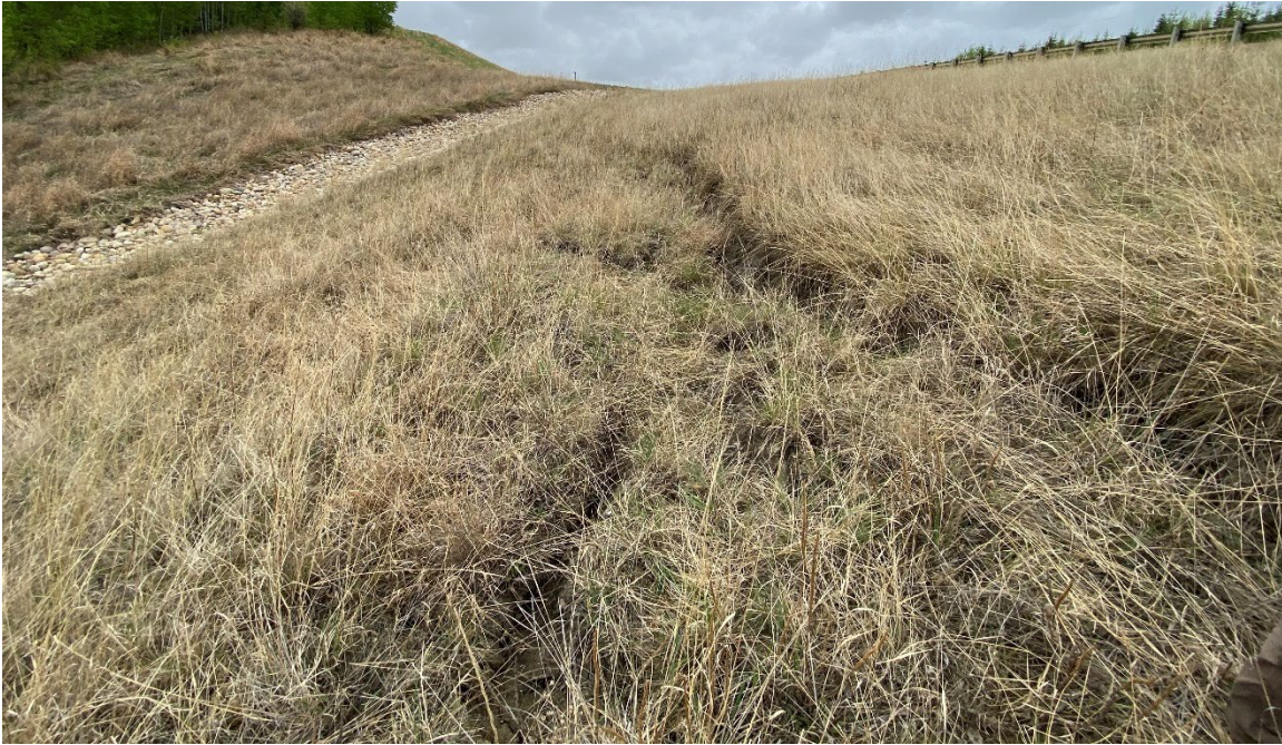
Photo 43-17.: Site B - Looking east towards the scarp of a shallow slide developing above the armoured swale that was identified in 2024 (33+850). Slide was more pronounced with a 0.4 m high main scarp and visible toe roll that extended to the edge of the swale.
