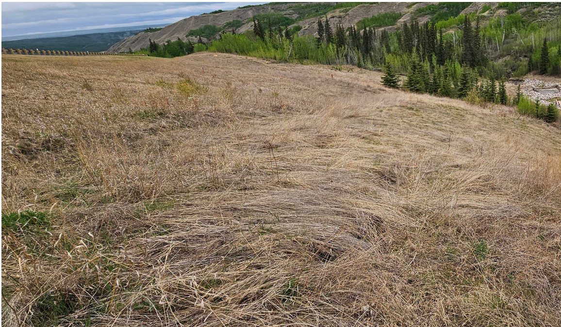
Photo 43-08.: View west along the sideslope above the armoured swale at the east side of Site A (33+530). Tension cracks have formed from shallow slide movement towards the erosion gully.
