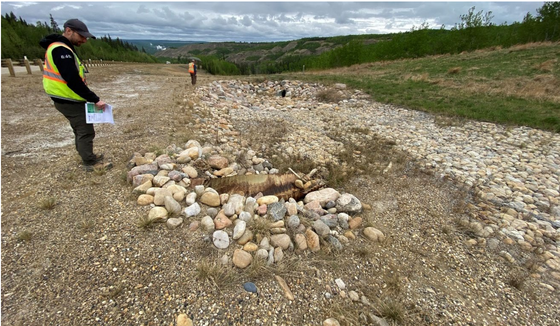
Photo 43-18.: Site B - View west towards centreline culvert outlet, CPP downpipe inlet and riprap protection near 33+900 on north side of road. No visible changes from the 2024 condition.
