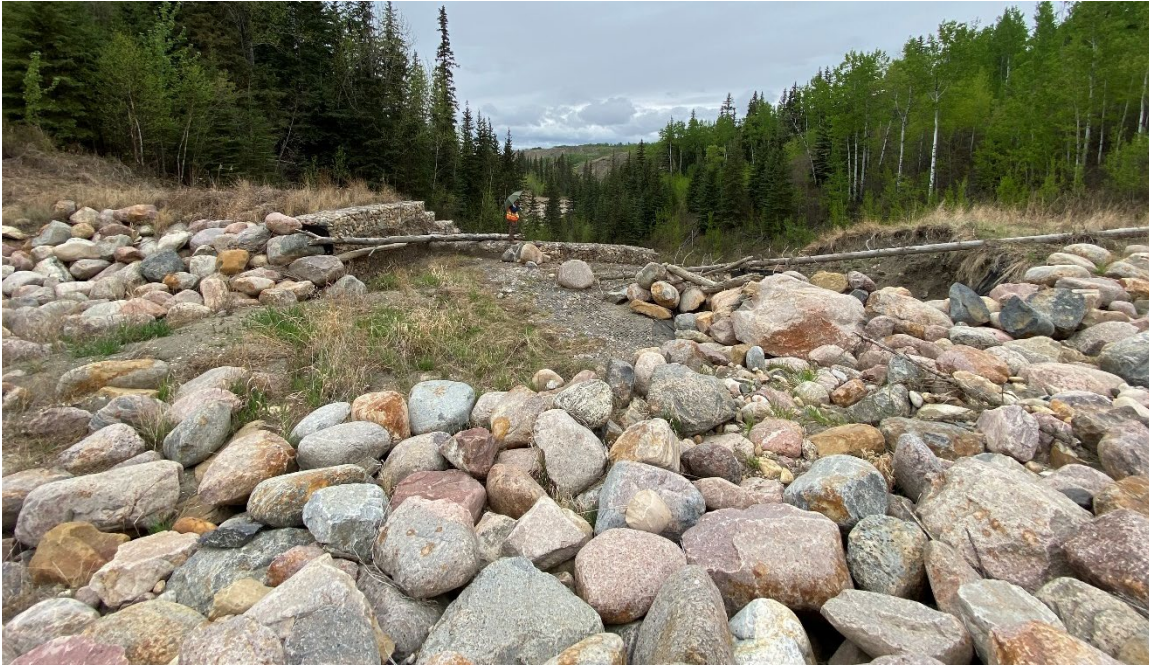
Photo 43-13.: Site B- view east at upstream end/inlet of the gabion drop structure with riprap berm near west end of the overland flow toe berm (33+625). Increased erosion and riprap displacement near the head of the erosion gully at the north side of the drop structure.
