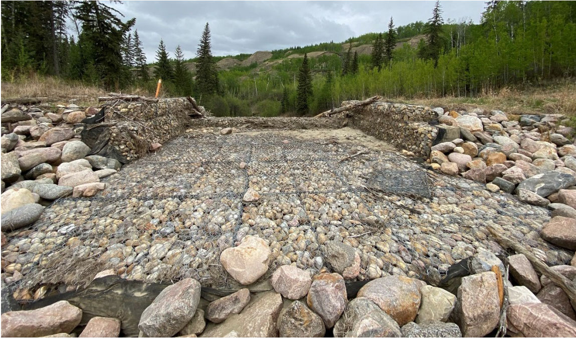
Photo 43-03.: View towards the northwest (downstream) at from the top of the Site A gabion drop structure (33+400). Debris and sediment buildup visible at the top of the structure from the 2024 high flow event. No major changes.
