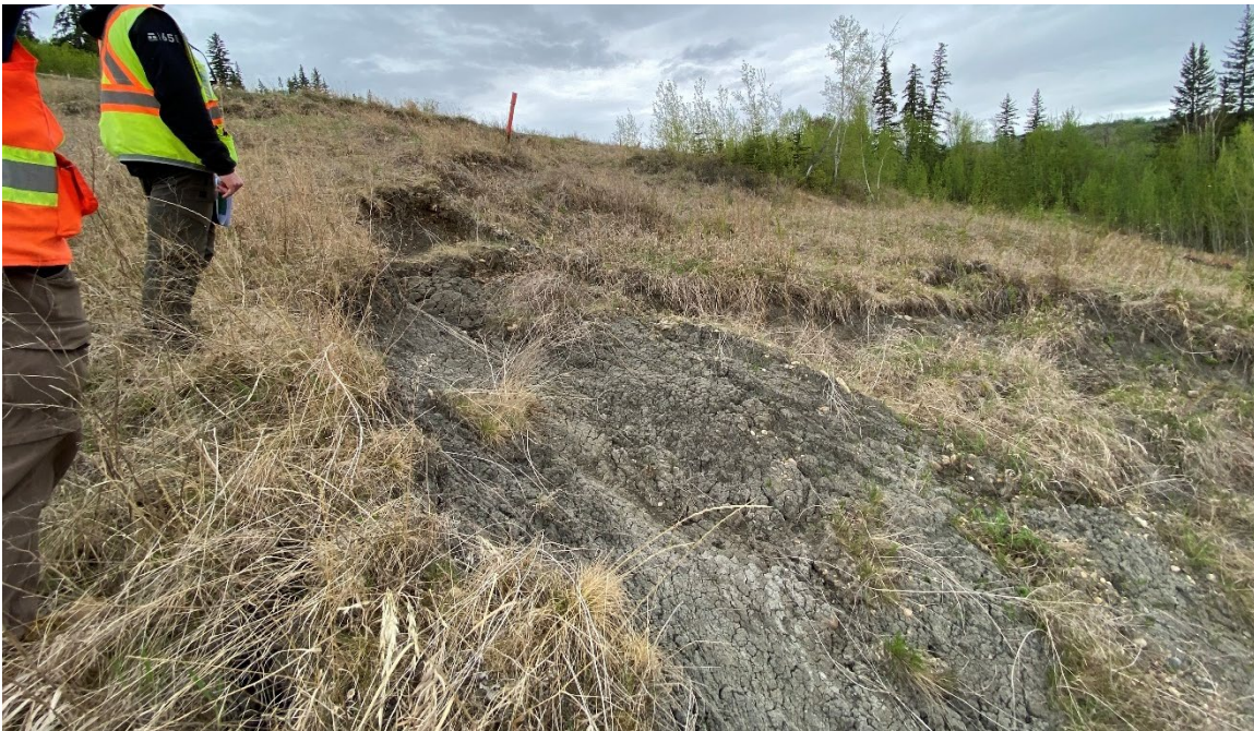
Photo 43-02.: Main slide scarp of active shallow failure downslope of the buried pile wall (33+325) first observed in 2017. Fresh scarps were observed in 2024 and had additional movement and minor retorgression.
