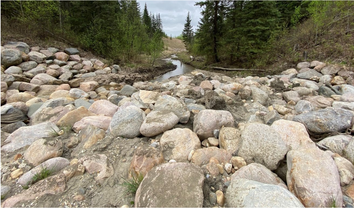
Photo 43-09.: Site B - View west (downstream) along the channel downstream of the gabion drop structure with displaced riprap and sediment buildup (33+600).
