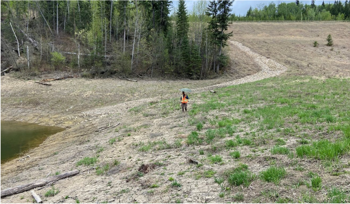
Photo 43-15.: Site B- view south of overland flow area above the culvert inlet near 33+800. Log and sediment debris buildup were visible from the 2024 high flow event.
