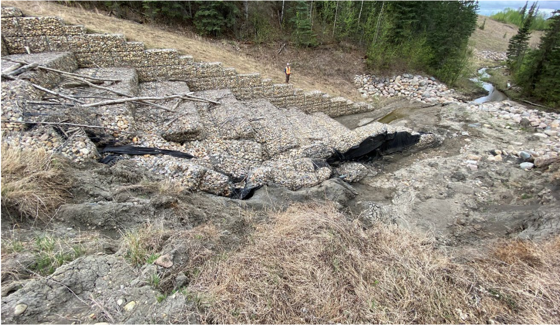
Photo 43-11.: Site B- view south towards the expanded damage and erosion gully along the north side of the gabion drop structure (33+610). Increased sediment buildup in dissipation bowl. Culvert outlet was open and flowing.
