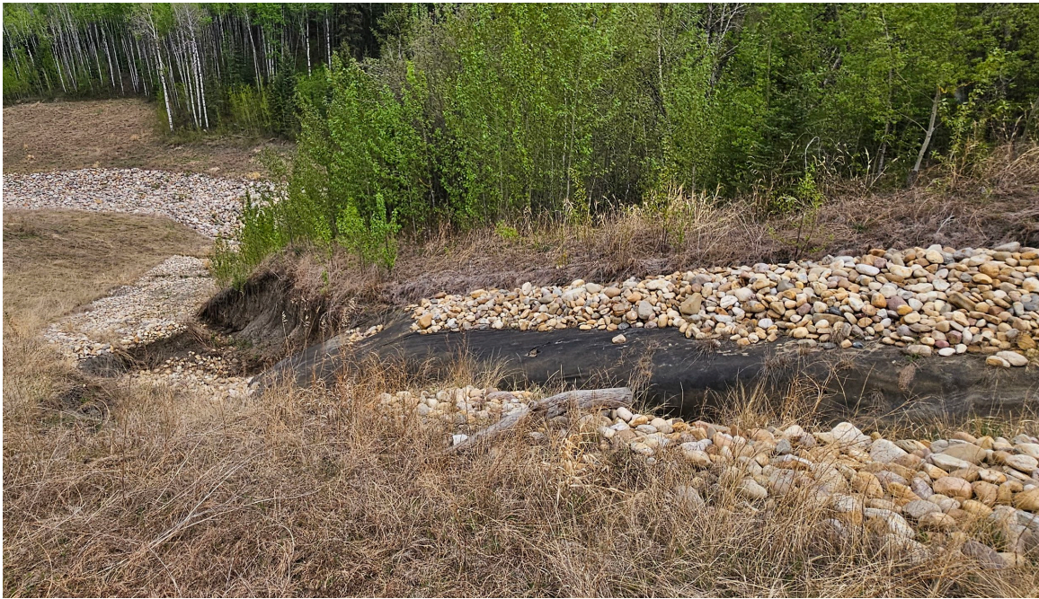
Photo 43-07.: Downslope view towards the north at the washed out riprap and extensive erosion gully damage within the armoured swale at the east side of Site A (33+500) first observed in 2020. Deeper and expanded erosion damage since 2024.
