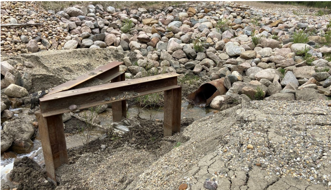
Photo 43-06.: Site A - View southwest towards the culvert inlet and debris deflector (33+500). Large buildup of sand and gravel from upstream washout during 2024 high flow event. Inlet was open and flowing. No significant change from 2024 condition.
