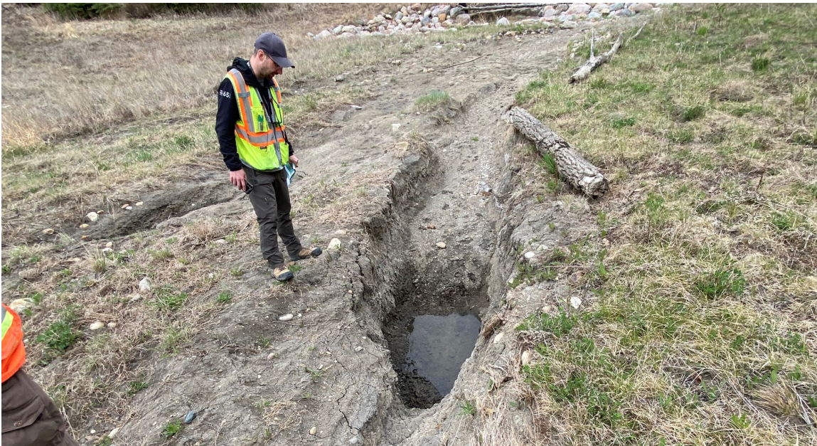
Photo 43-14.: Site B- view east towards a 1.5 m deep scour hole the formed during the 2024 high flow event within the overland flow area upstream from the drop structure near 33+675.
