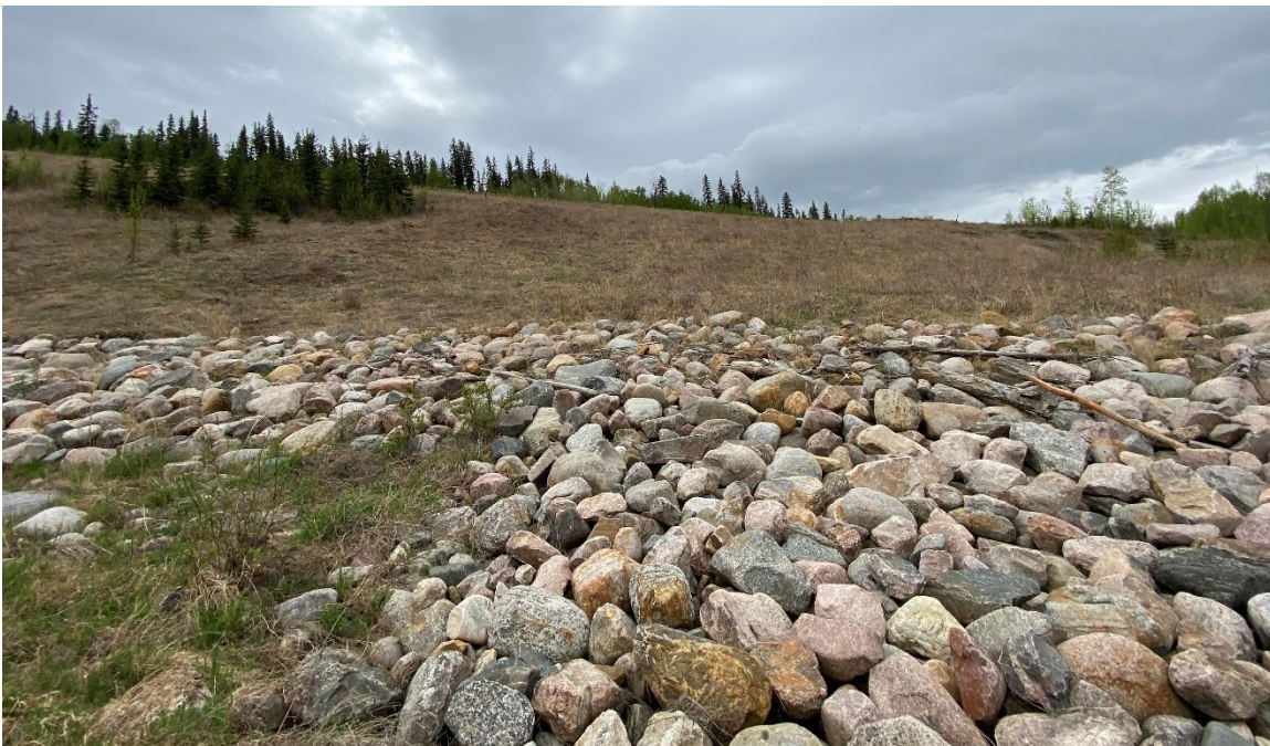
Photo 43-04.: Looking south at the area of previous slumping associated with culvert erosion below pile wall and regraded slide during construction in 2017 (33+430). No visible changes from 2024 condition.
