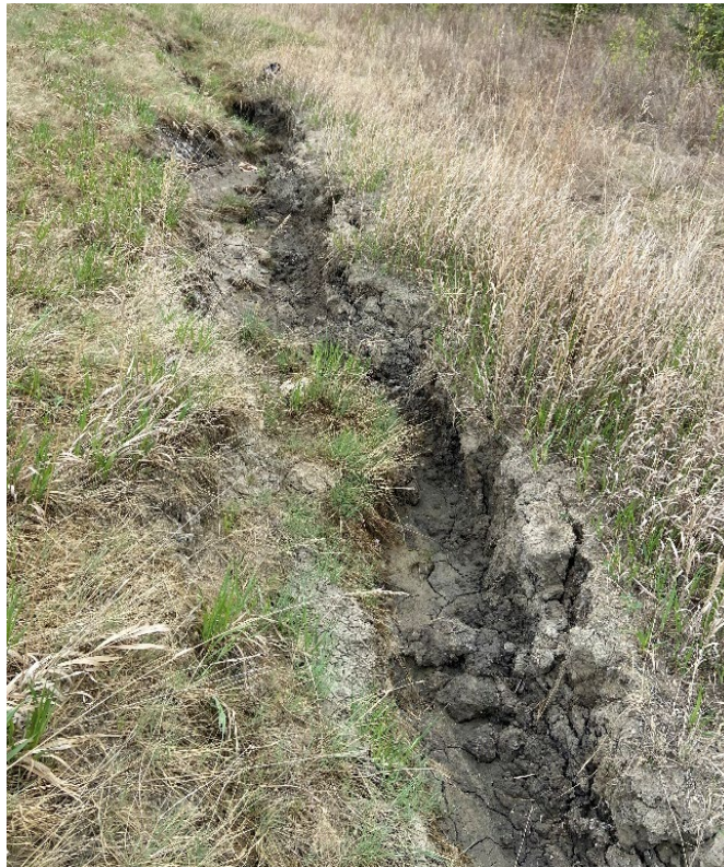
Photo 43-19.: Site B – Increased erosion within gully that has formed upstream of the culvert inlet within the south ditch between approximately 33+900 to 34+010.
