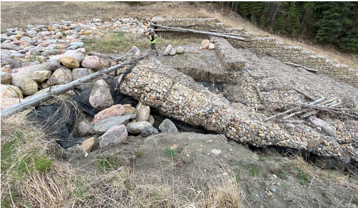
Photo 43-12.: Site B- view south towards the top of the gabion drop structure where high flow outflanked the structure along the outside of the north sidewall during the 2024 high flow event causing subsequent collapse from undermining. Logs and wood debris buildup visible.
