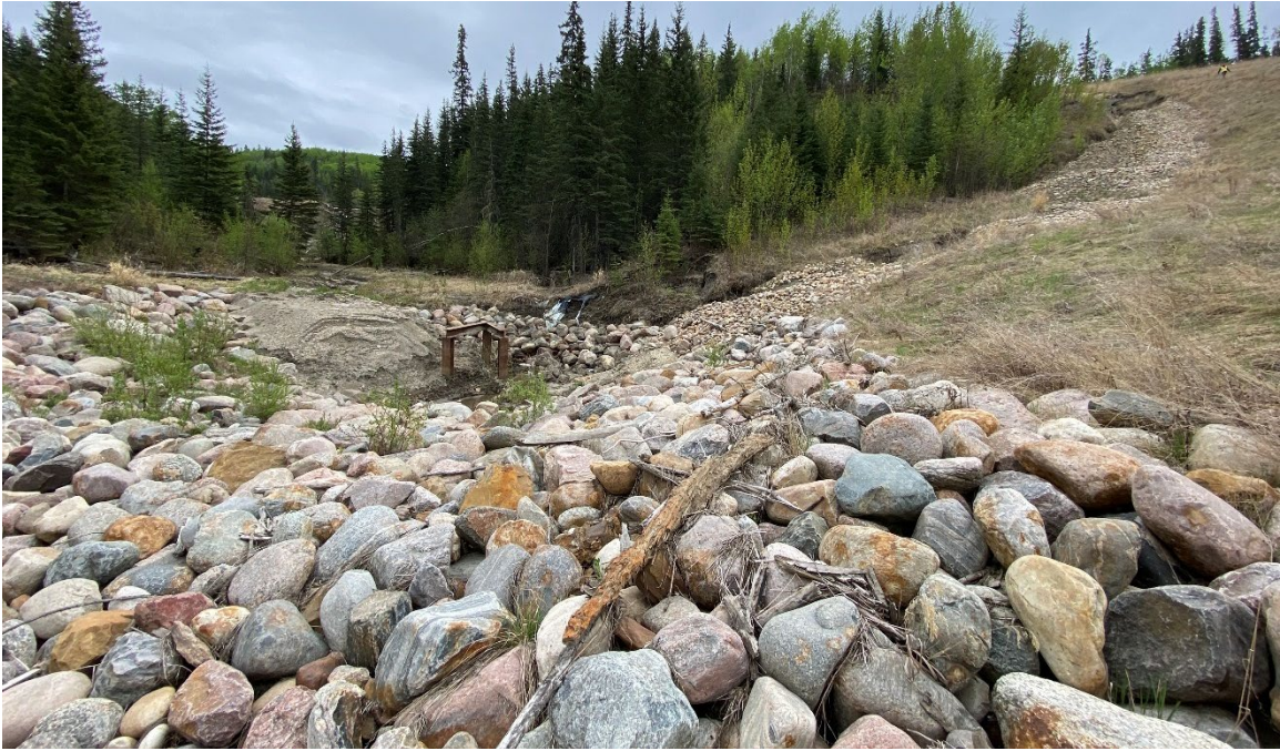
Photo 43-05.: Site A - Standing atop the armoured overflow channel looking towards the southeast (upstream) near 33+525. Buildup of woody debris and sediment visible from the 2024 high flow event. Increased gully erosion along the armoured swale and slumping of the south channel banks.
