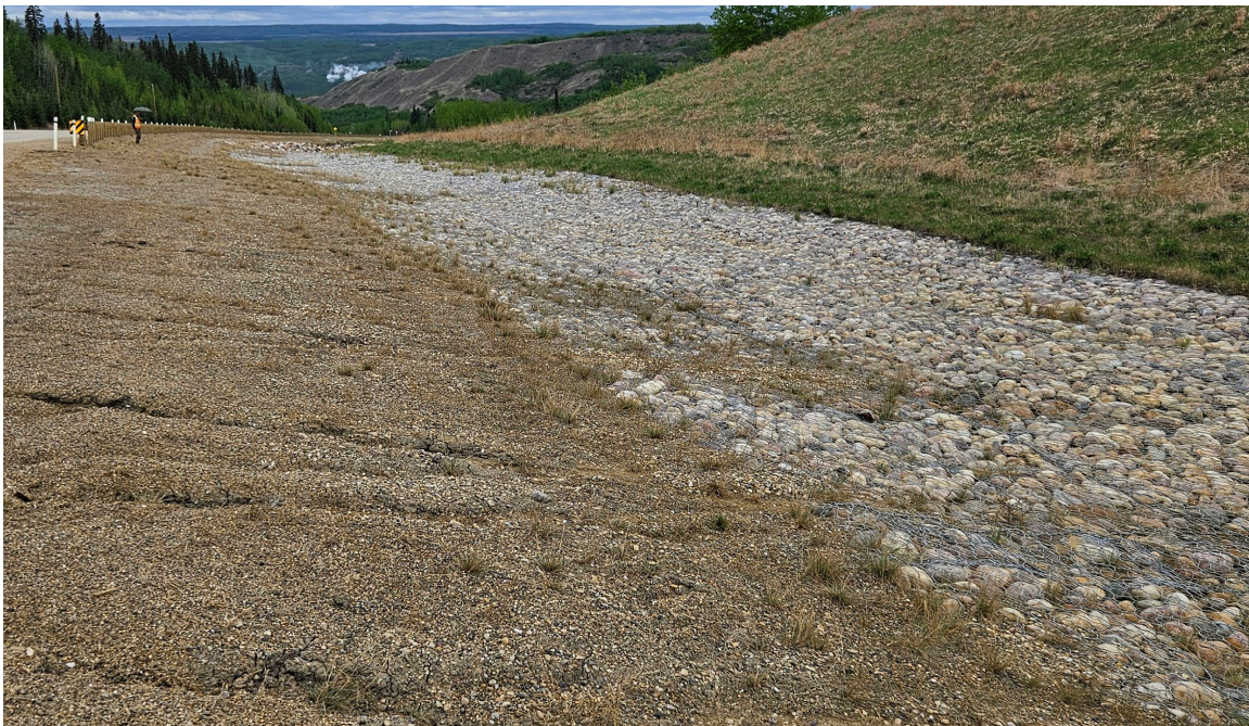
Photo 43-20.: Site B – Shallow rill erosion between the road sideslope and north ditch gabion armour had no major change compared to the 2024 condition (34+000).
