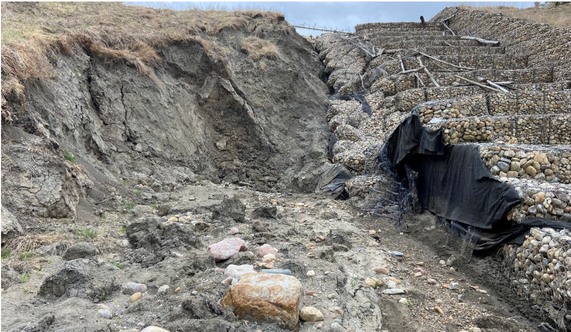
Photo 43-10.: Site B- view east (upstream) from the base of the gabion drop structure and riprap dissipation bowl at the culvert outlet (33+600). Additional erosion expansion and complete gabion collapse along the north sidewall of the drop structure from the erosion gully that formed when high flow outflanked the structure in 2024. Lower area previously compromised from culvert joint leak and piping.
