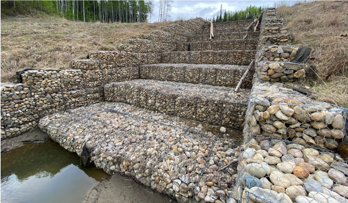
Photo 43-01.: View towards the southeast (upstream) from the base of the Site A gabion drop structure. No major change from 2024 condition. Debris visible from high flow event and there was sediment buildup within the dissipation bowl at the base of the drop structure.
