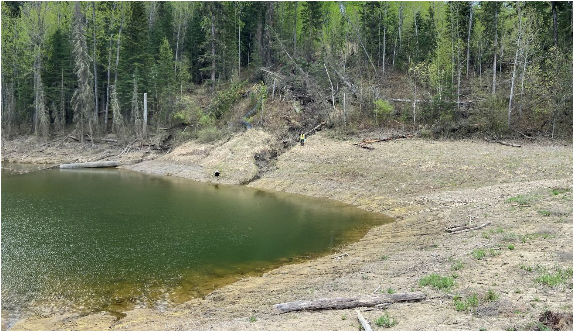
Photo 43-16.: Site B - Looking south towards the outlet of the CPP down pipe near the culvert inlet (33+850). Increased gully erosion and sliding since 2024 due to a leaking joint that requires repair. Water is ponded above the damaged culvert inlet (pinched) that has significantly restricted flow capacity.
