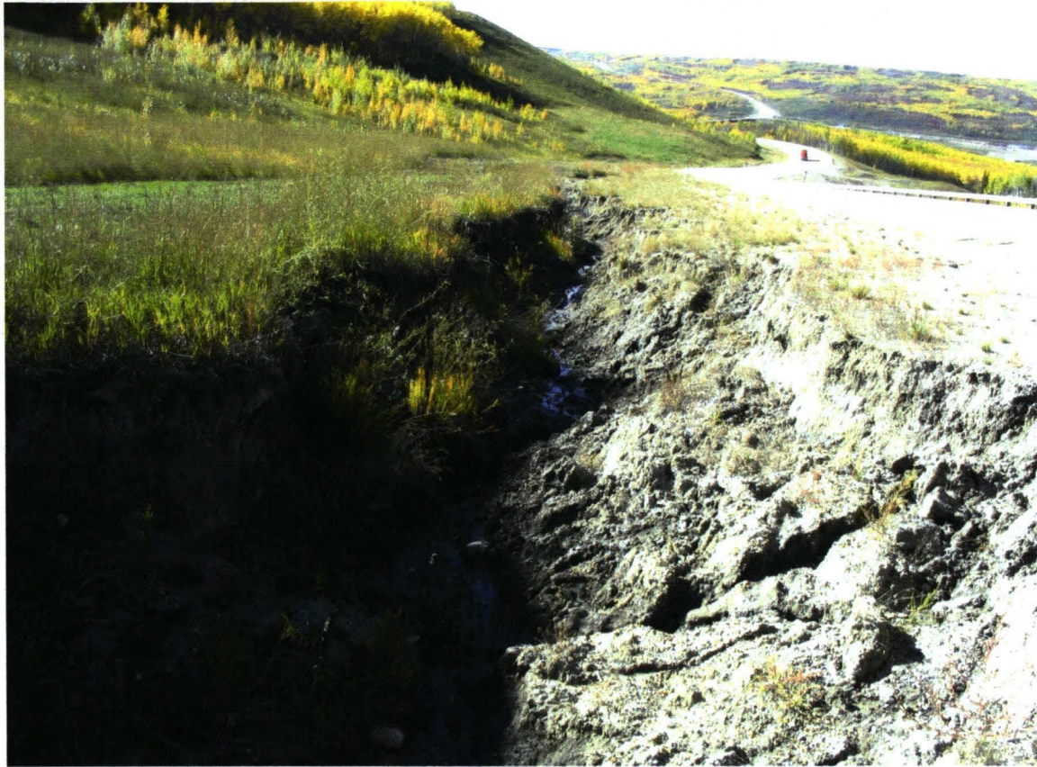
PHOTO 7 LOOKING DOWNSTREAM FROM ABOUT STA. 12+520
