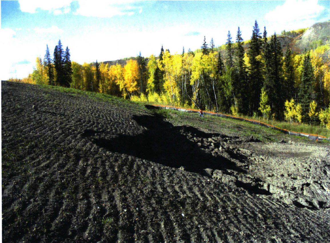
PHOTO 12 LOOKING WEST AT SLIDE AREA
