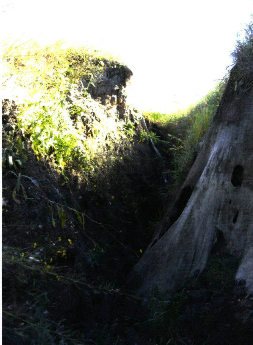
PHOTO 3 DEEPEST PART OF EROSION CHANNEL IS ABOUT 3m DEEP
