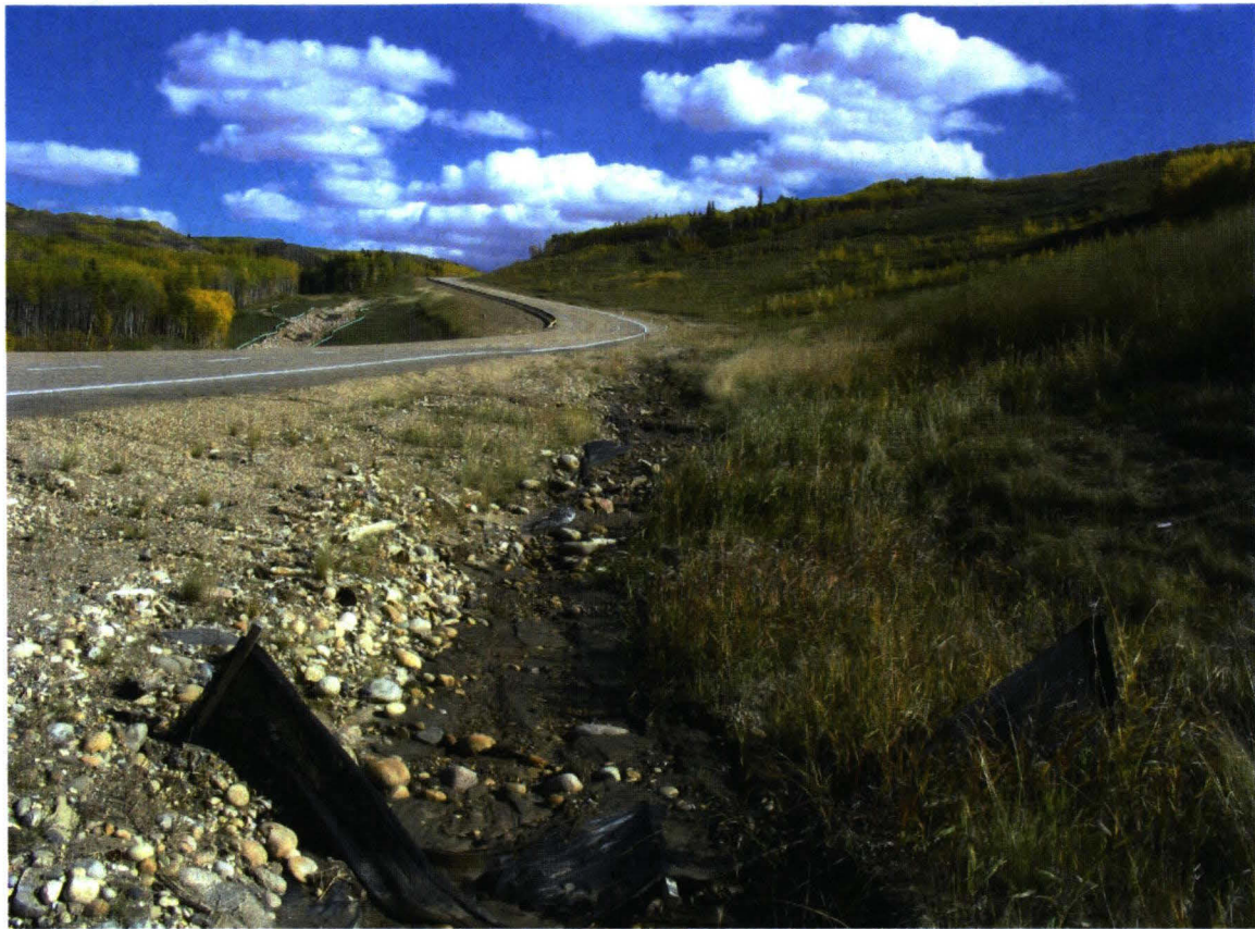
PHOTO 5 LOOKING UPSTREAM (EAST) FROM INLET OF CULVERT AT ABOUT STA. 12+120
