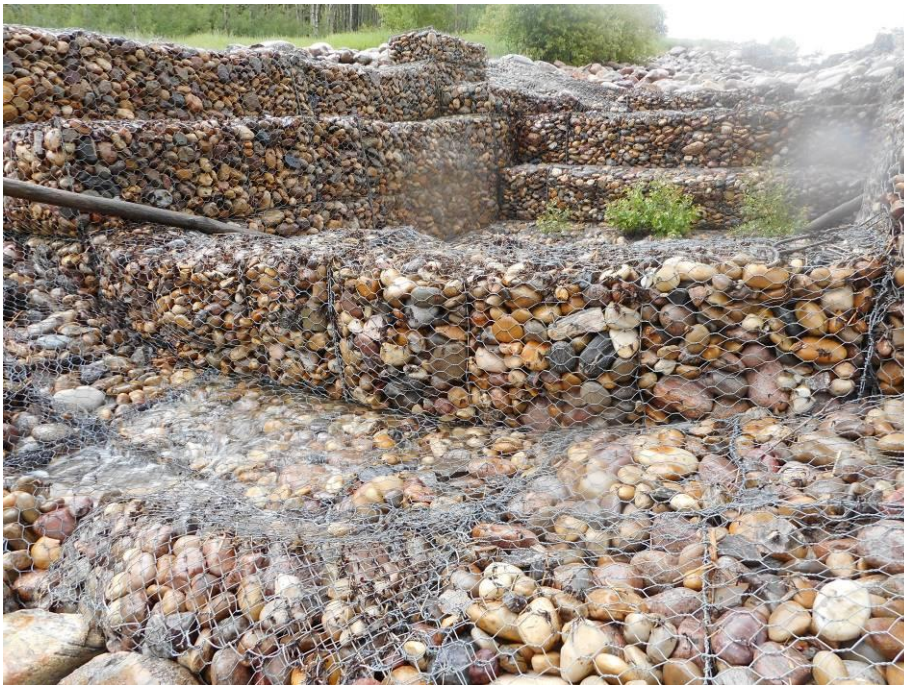
Photo 7-02. Looking upstream from lower gabion drop structure (32+495).
