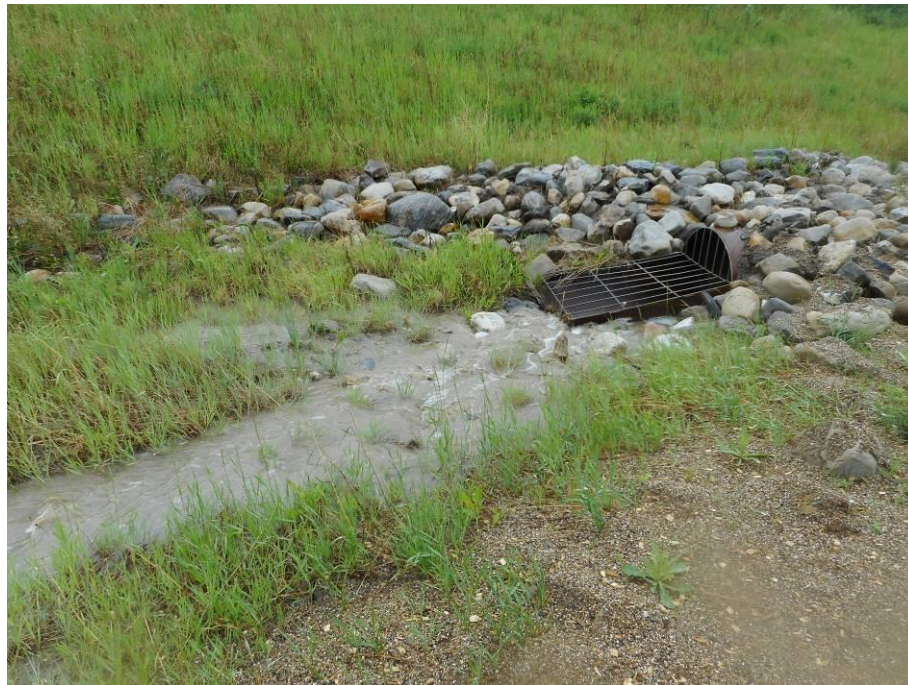
Photo 7-18. Culvert inlet at west end of erosion control section (32+050).
