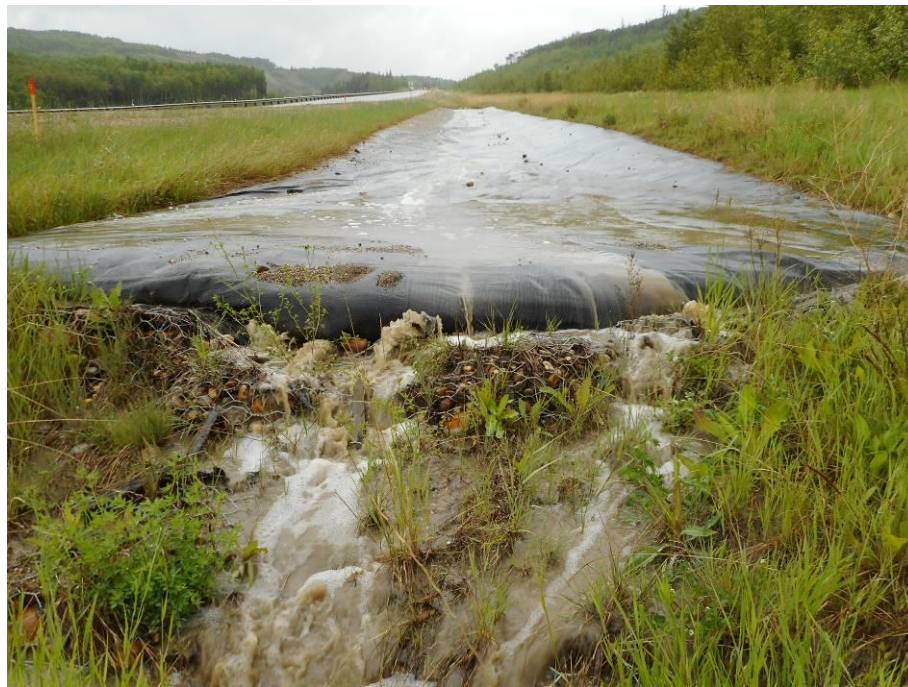
Photo 7-15. Looking upslope (east) at the Coletanche geomembrane erosion control section (32+250).
