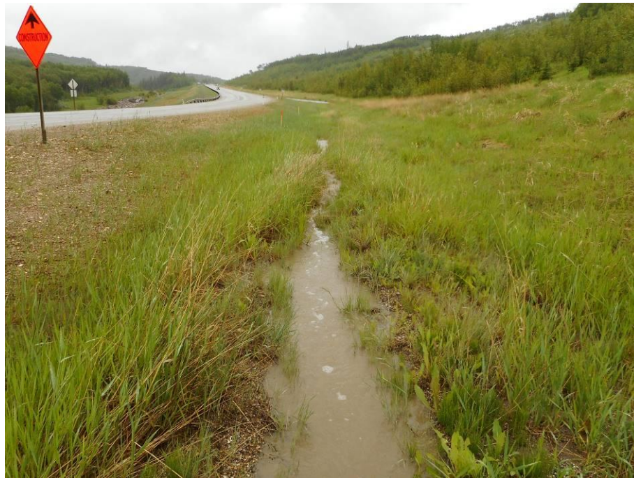
Photo 7-16. Looking east towards 300 m diameter channel sock erosion control section (32+150). Section had good vegetation growth.
