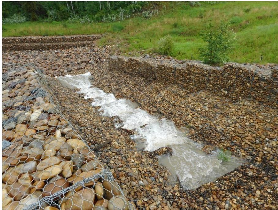
Photo 7-08. Lower segment of the gabion channel bend and drop structure (31+800).
