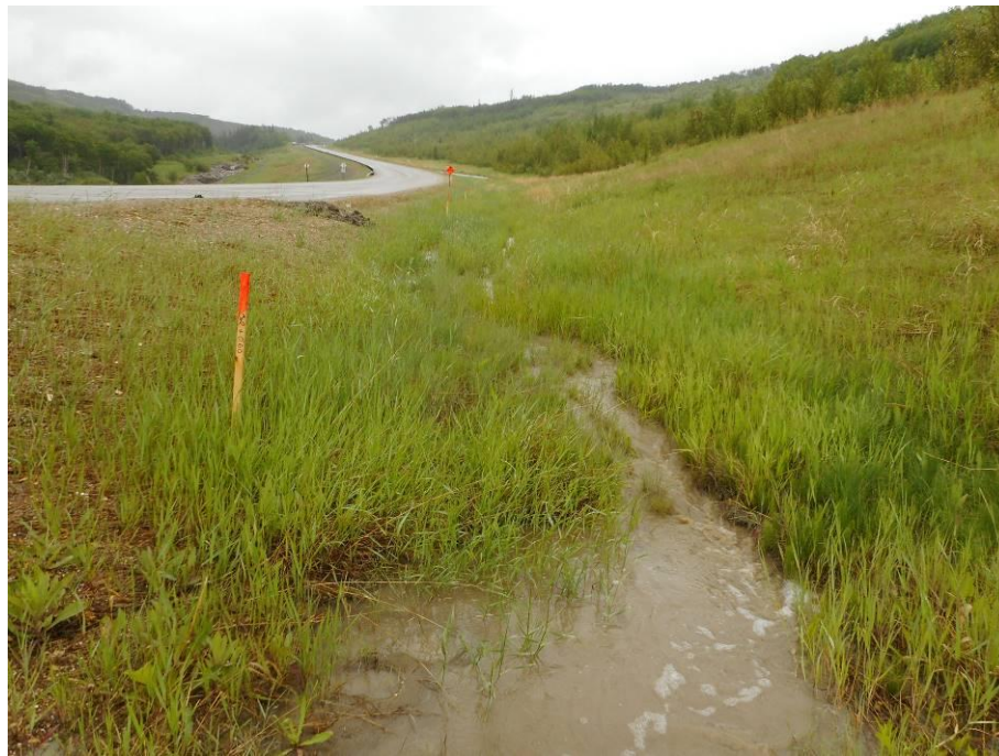
Photo 7-17. Looking east towards rolled erosion control product (turf reinforced matting) section (32+75).
