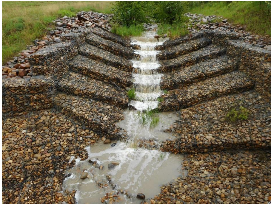
Photo 7-07. Upper segment of the gabion channel bend and drop structure (31+800).
