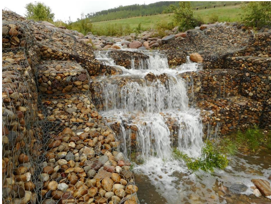
Photo 7-04. Upper gabion drop structure (32+540).
