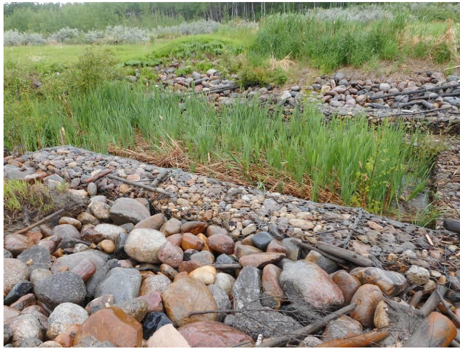
Photo 7-06. North channel inlet structure. Note vegetation and willow growth (32+855).
