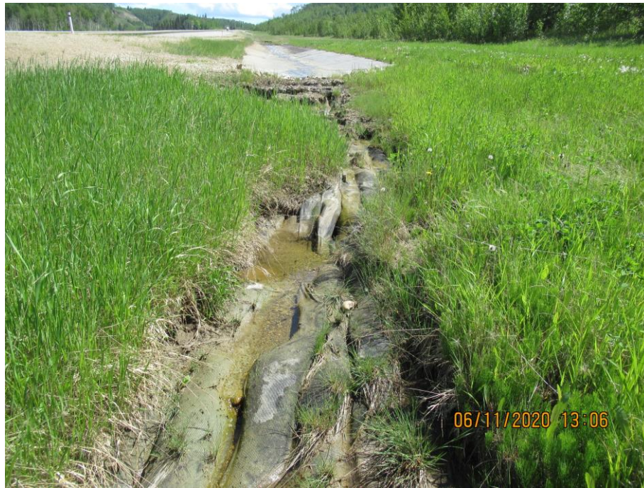
Photo 7-10. Looking east towards 300 m diameter channel sock erosion control section (32+150). Section had good vegetation growth but increased channelized erosion at the top of the section near the boundary of the geomembrane section.
