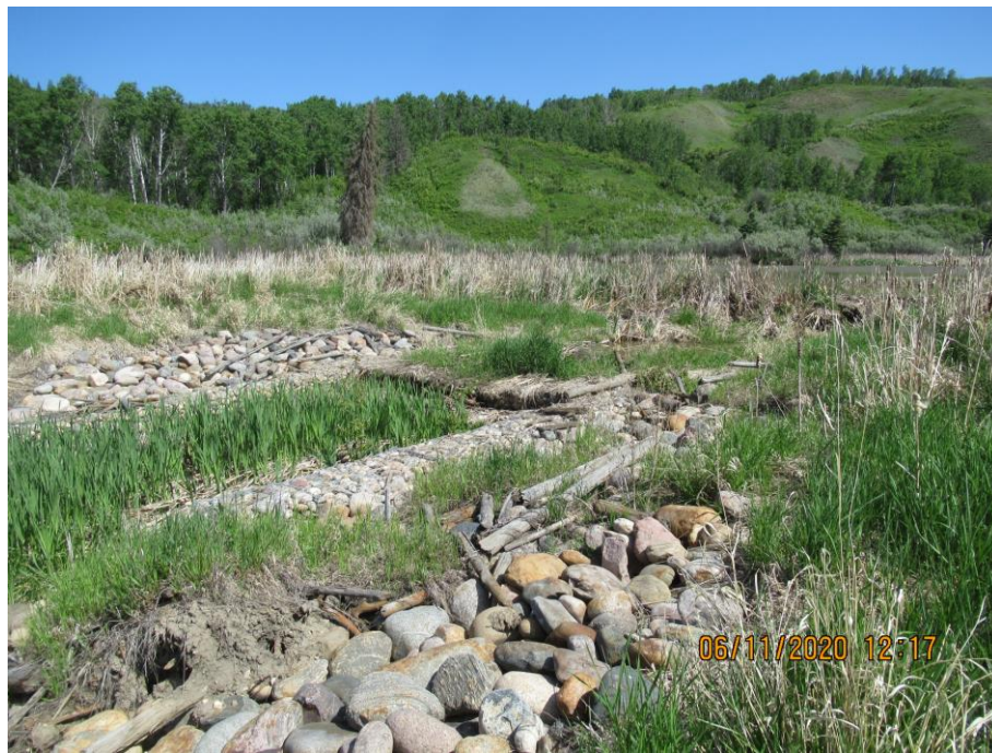
Photo 7-06. North channel gabion inlet structure. Condition was comparable to previous inspections (32+855).
