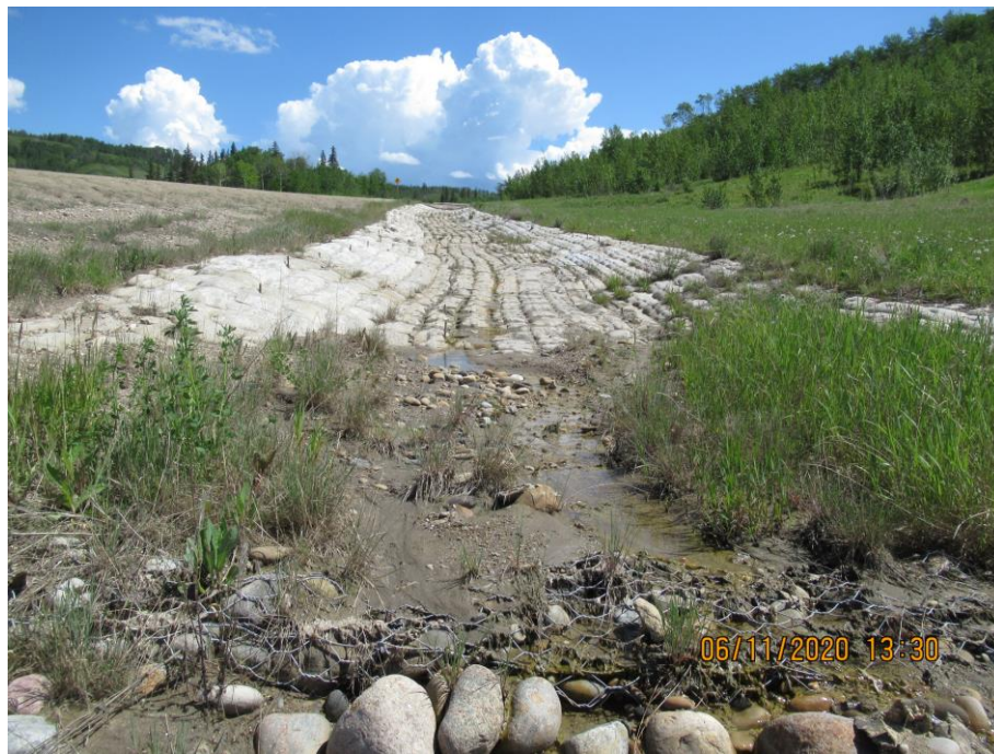
Photo 7-16. Looking east towards pillow concrete section (32+800). Section was performing well. Minor concrete deterioration was noted in select areas but erosion mitigation function was not impacted.
