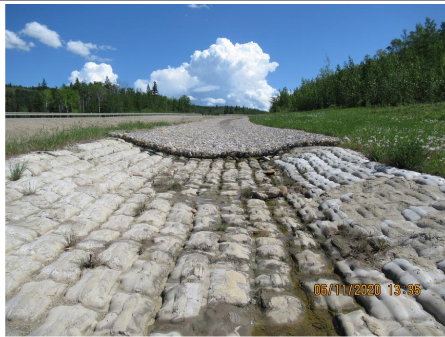
Photo 7-17. Looking east (upslope) at the top of the erosion control test ditch (32+900). Ditch upslope of the test section has been lined with gabion mattress as part of the 2018/2019 East Daishowa (PH42) mitigation work. The ditch and new mitigation works were in good condition.
