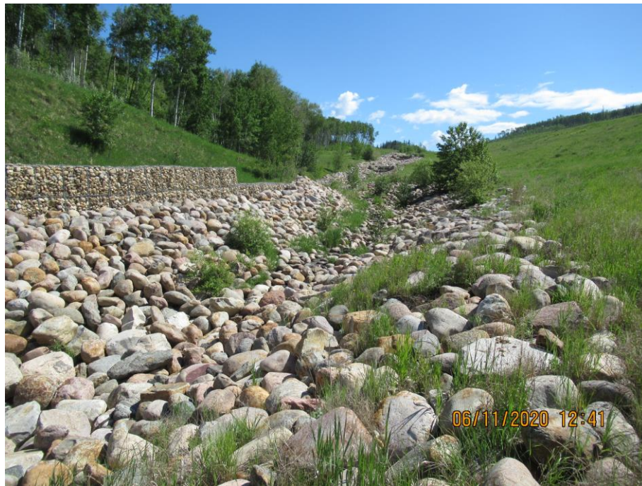
Photo 7-01. Gabion retaining wall and armoured channel observed in good condition (32+290).
