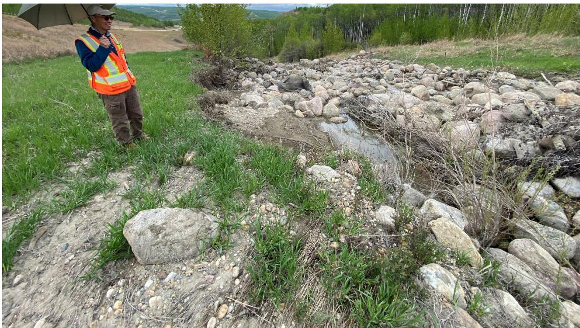
Photo 7-07.: Looking west (downstream) along the south channel bank where an upstream buildup of washed out riprap has infilled the channel and caused overflow above the south bank and outside the upper gabion drop structure (32+550). High flow path evident from grass disturbance and sediment buildup outside the banks.
