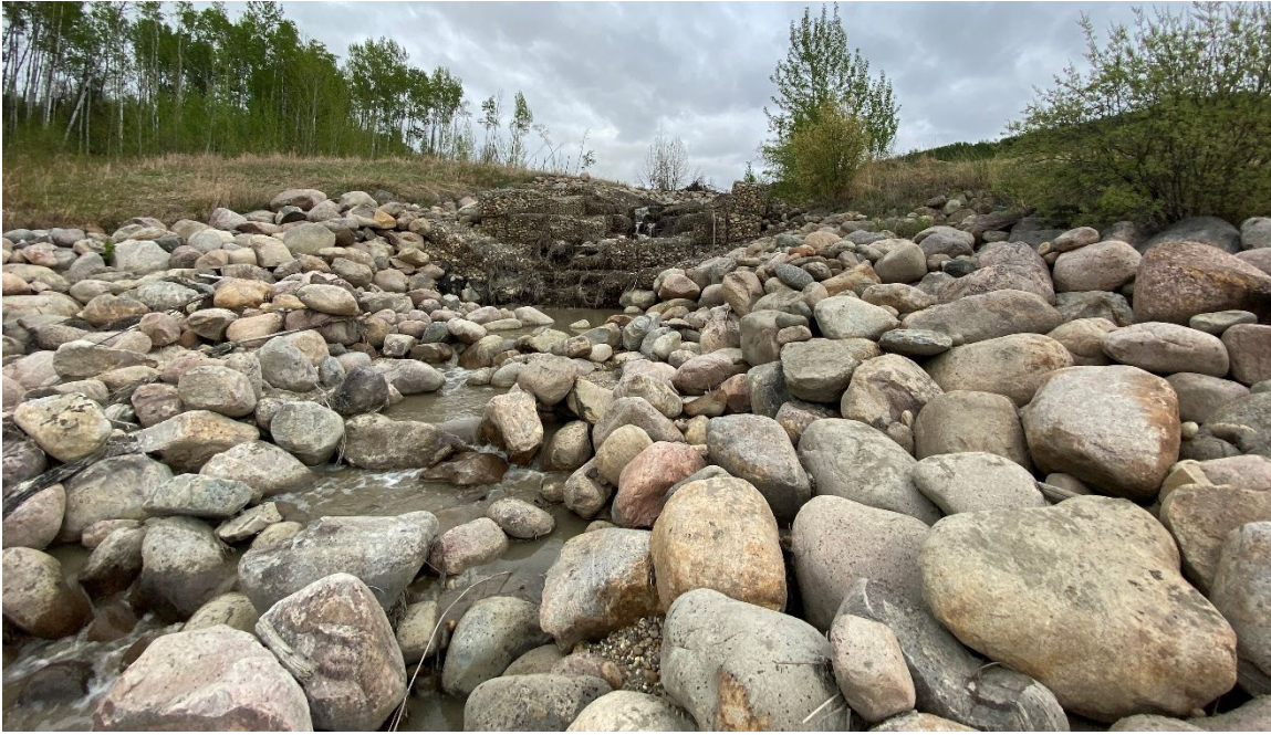
Photo 7-09.: View east towards the upper gabion drop structure (32+550) with major basket deformation and damage. Some riprap was displaced at the toe of the structure, but the downstream channel riprap was intact up to the lower drop structure approximately 40 m further downstream.
