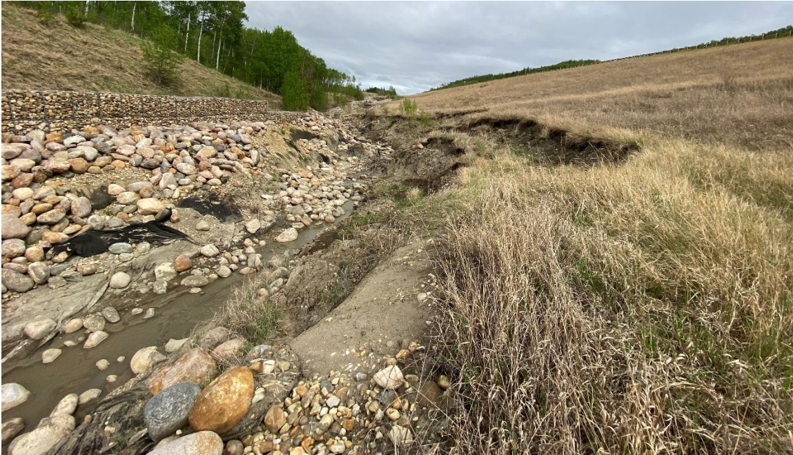
Photo 7-15.: View east of the channel segment with major channel downcutting and undermining of the south bank that has resulted in the development of slides into the north toe of the highway embankment between approximately 32+275 and 32+350.
