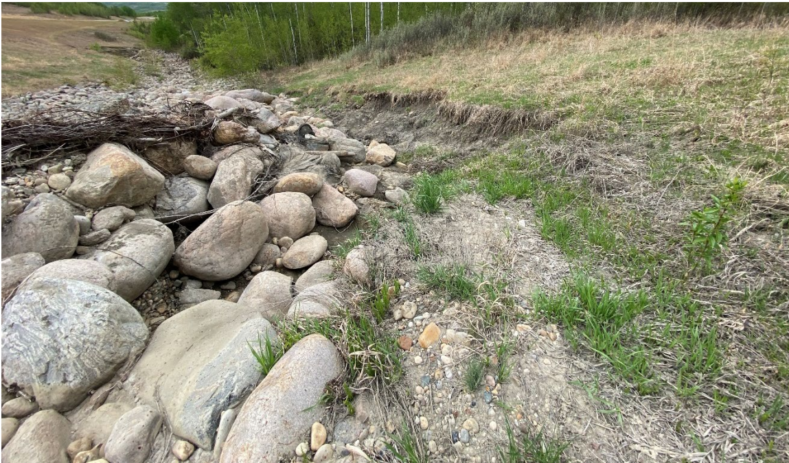
Photo 7-11.: View west at the top of the lower gabion drop structure (32+480). The 2024 high flow went outside the drop structure on the north side and formed an erosion gully which in 2025 was approximately 6 m wide and 2 m deep. Previous erosion damage has been observed in this area in the past.
