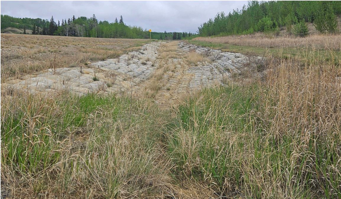
Photo 7-28.: Looking east towards pillow concrete section (32+800). Section was performing well. Minor concrete deterioration was noted in select areas and there were some protruding rebar pins, but erosion mitigation function was not impacted.
