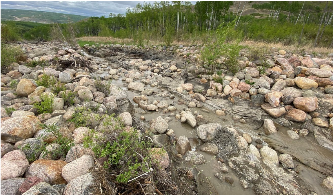
Photo 7-05.: Looking west (downstream) at channel erosion (32+650). There was slightly worse channel downcutting and washout of the riprap rock within the bottom of the channel since the 2024 callout inspection.
