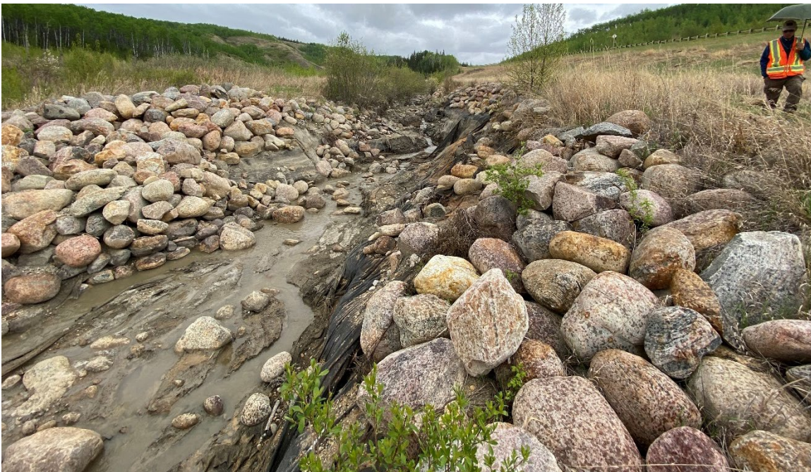
Photo 7-04.: Looking east at channel downcutting (up to 2 m depth) and bank washout creating near vertical bank exposures within the channel bottom resulting in collapse of the riprap along the top of bank (32+650).
