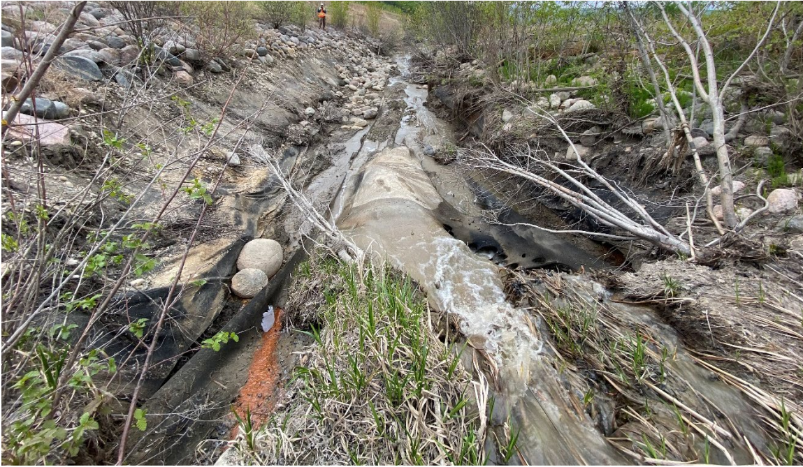
Photo 7-03.: Looking west (downstream) at the eastern end of the primary scour (up to 1.5 m deep) and initiation of severe channel degradation and bank washout within the north channel segment that extends from approximately 32+800 to 32+600.
