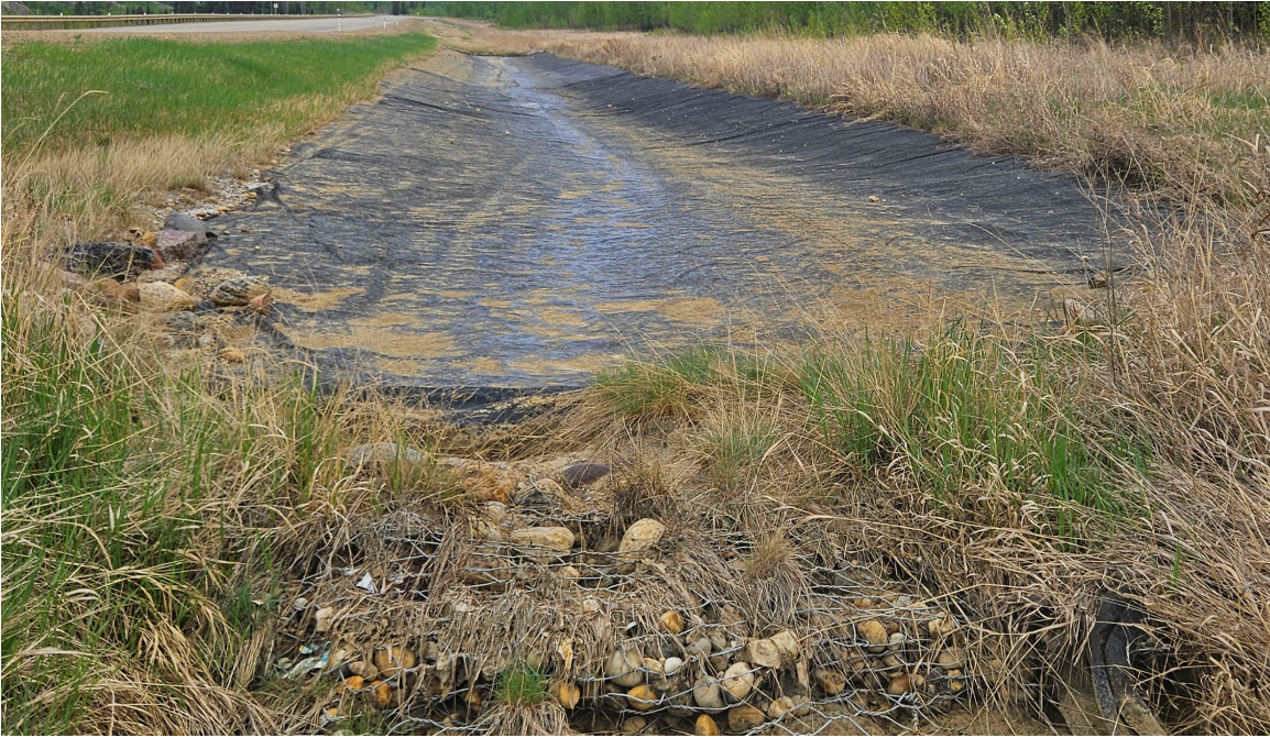
Photo 7-23.: Looking upslope (east) at the Coletanche geomembrane erosion control section (32+250). Was in good condition with no new damage observed in previous patch repair area.
