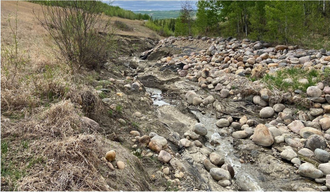
Photo 7-13.: View downstream (west) of major channel downcutting (up to 5 m in depth) and washout for an approximately 100 m length of the channel between 32+280 and 32+380.
