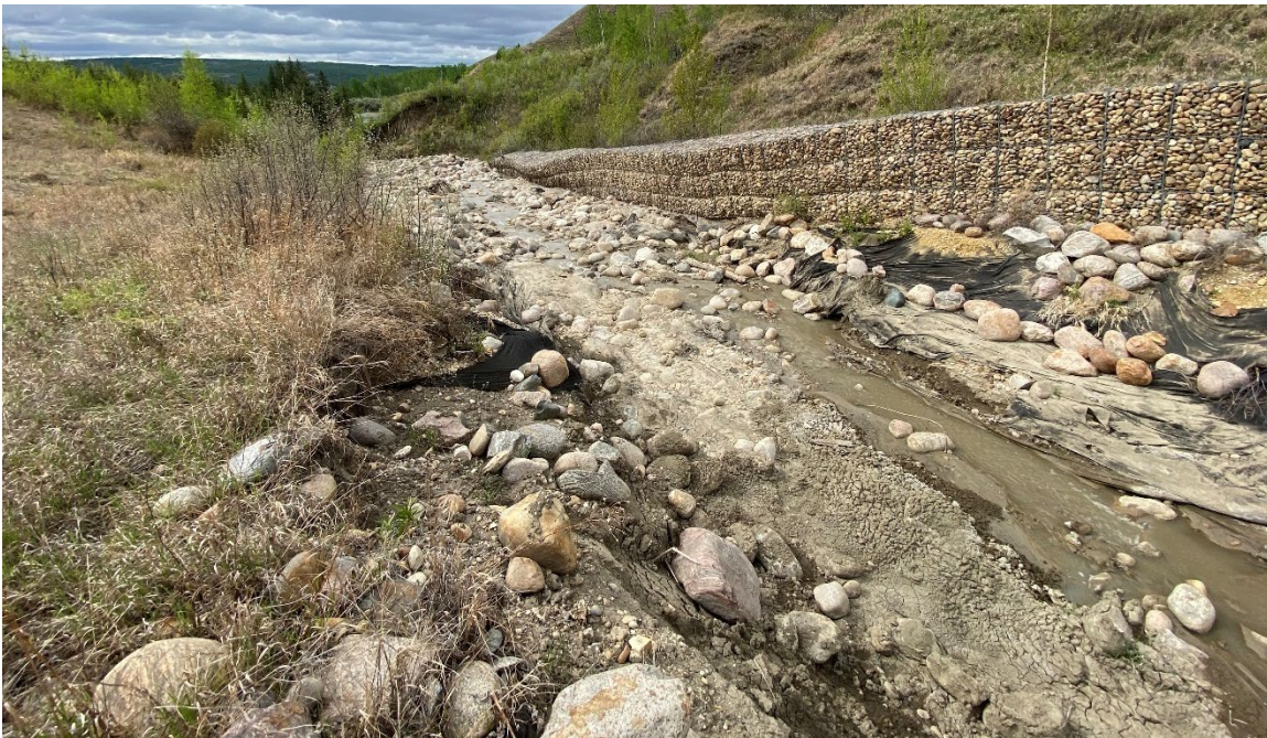
Photo 7-16.: View northwest towards the gabion retaining wall near 32+275 where the riprap at the base of the wall has been washed out as a result of severe channel downcutting.
