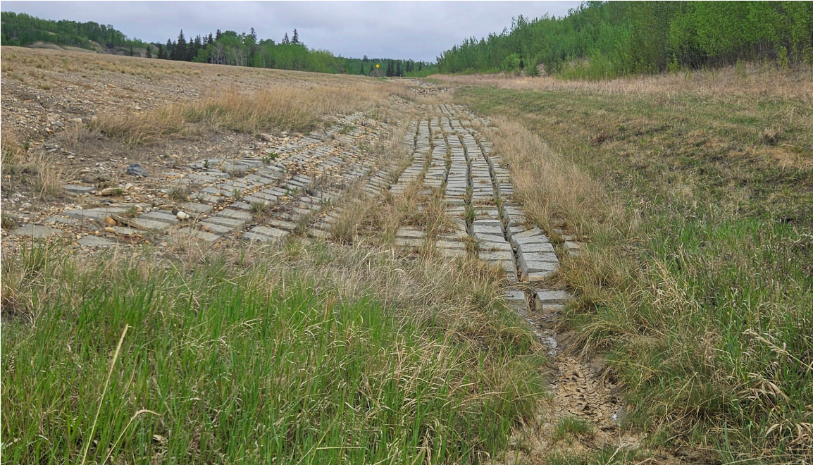
Photo 7-27.: Looking east towards cabled concrete section (32+700). Section was performing well. Minor erosion damage was noted on the north side of the ditch. No major change from the 2023 condition.
