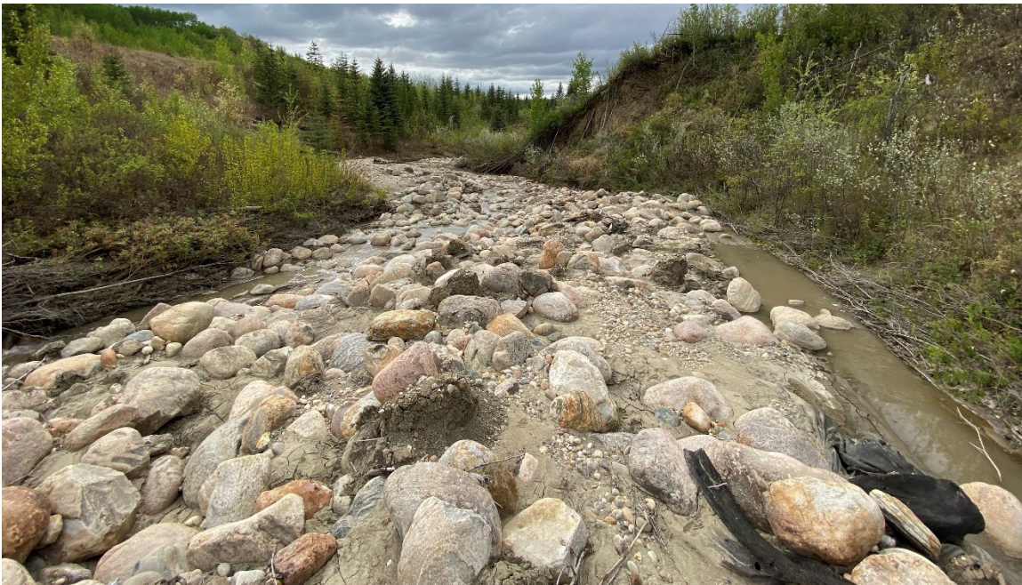
Photo 7-18.: View downstream from west end of the gabion retaining wall (32+250) where channel was infilled with a buildup of washed out channel riprap and sediment, displacing water flow to the channel sides.
