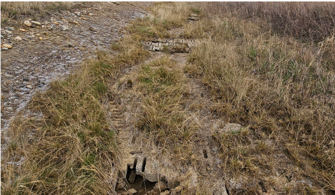
Photo 7-26.: View of the damage within the interlocked concrete block (i.e., Lafarge paving stones) paving stone section (32+600). Blocks have deteriorated and broken up in numerous locations and have been undermined by erosion exposing geotextile fabric beneath. Overall section is worse relative to the other test sections but had no major changes since the 2023 condition.
