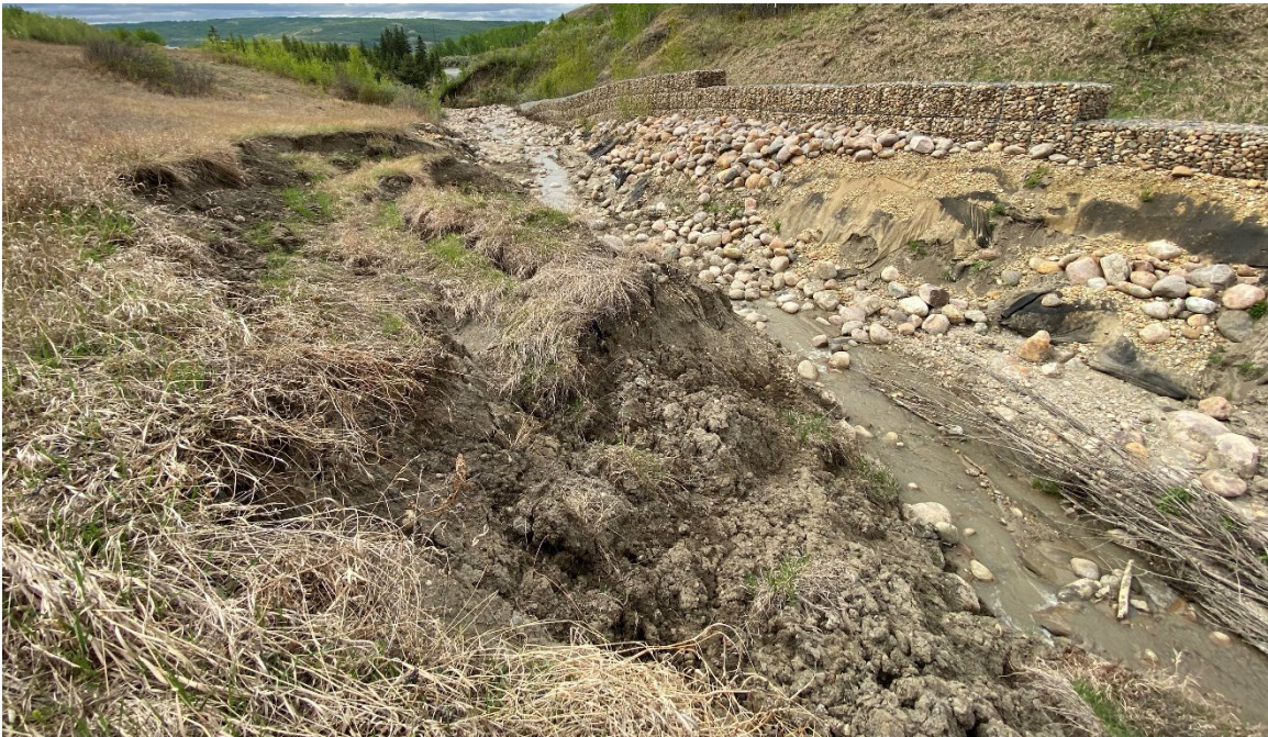
Photo 7-14.: View northeast of the channel segment with major channel downcutting and washout near 32+325. Undermining of the south bank has resulted in bank collapse and sliding towards the highway embankment. Near vertical bank exposures have developed on the north bank.
