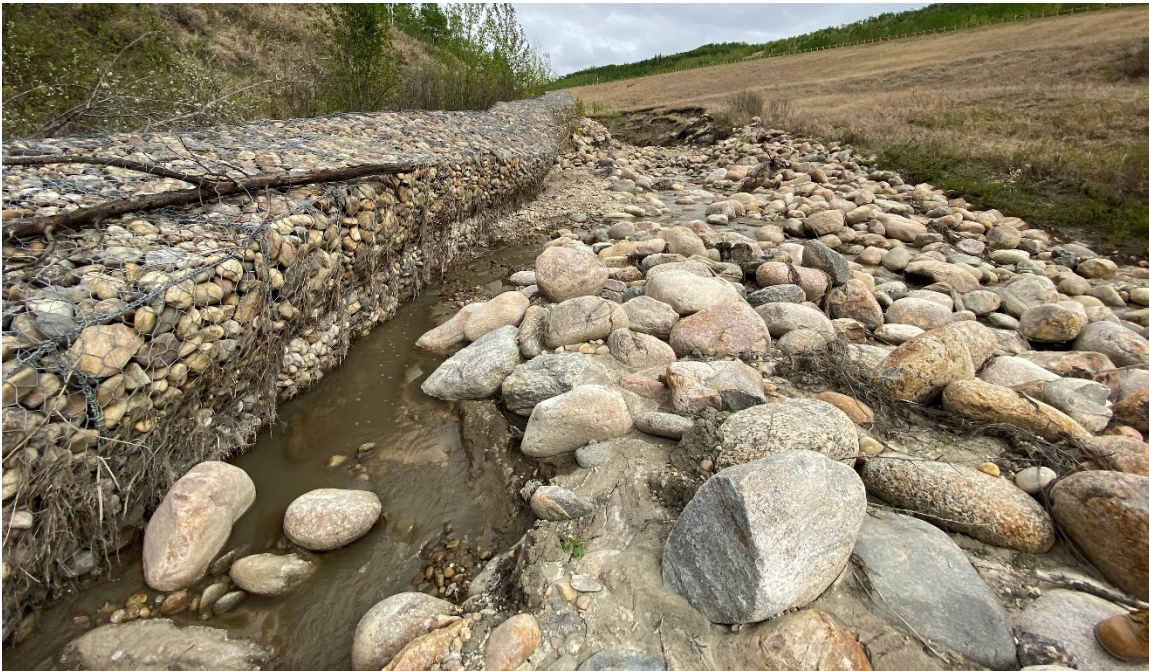
Photo 7-17.: View east along the west end of the gabion retaining wall with visible tilt towards the channel due to undermining at the base from channel scour (32+225).
