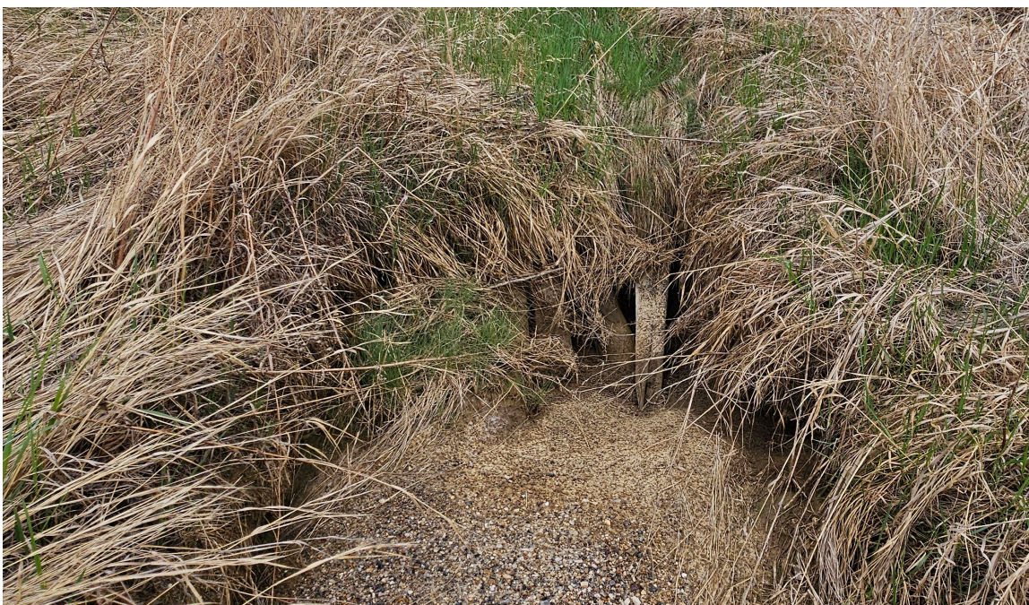
Photo 7-22.: Looking east towards 300 m diameter channel sock erosion control section (32+150). Section generally had good vegetation growth within previous erosion gully in ditch bottom. A 0.5 m deep scour pool was observed downstream of the Coletanche erosion control transition.
