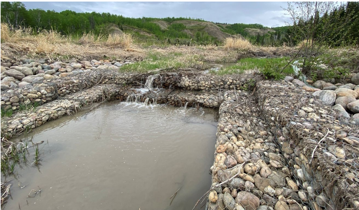
Photo 7-02.: View upstream at the gabion inlet structure near 32+850. Debris buildup and vegetation displacement (willows laid over) from the 2024 high flow event. Minor deformation of the gabion baskets at the inlet.
