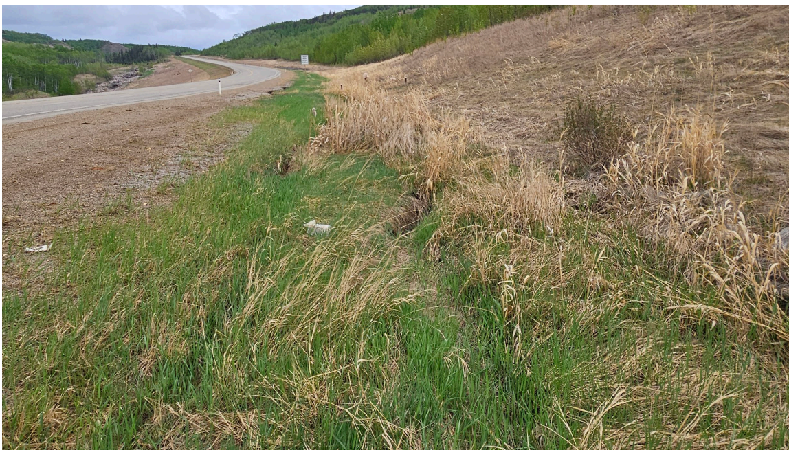
Photo 7-21.: Previously observed channelized erosion has since revegetated within the rolled erosion control product (turf reinforced matting) test section (32+100). Minor erosion was present along tire ruts.
