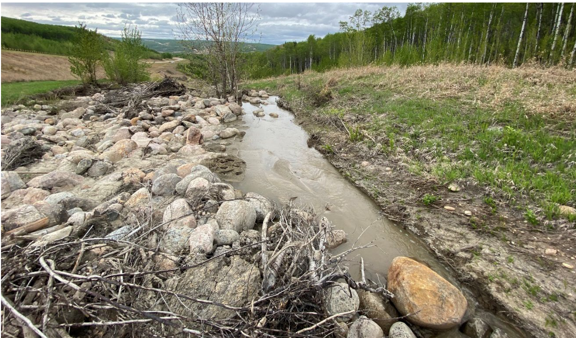
Photo 7-06.: Looking west (downstream) at a buildup of washed out riprap, sediment and woody debris from erosion within the upstream north channel that has caused channel infill near 32+575 and diverted the high water flow to overtop both banks and flow around the upper drop structure on the south side.
