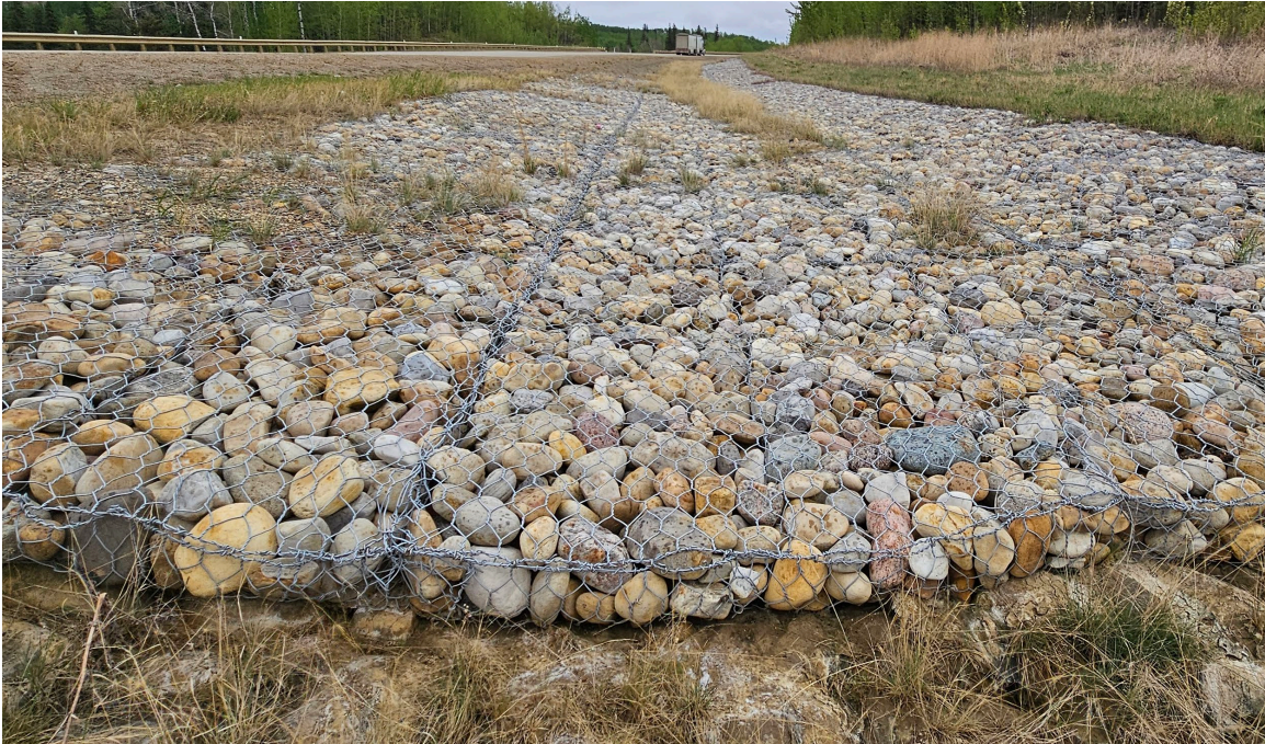
Photo 7-29.: Looking east (upslope) at the top of the erosion control test ditch (32+900). Ditch upslope of the test section has been lined with gabion mattress as part of the 2018/2019 East Daishowa (PH042) mitigation work. The ditch and new mitigation works were in good condition with no observable change apart from increased vegetation growth since 2023.
