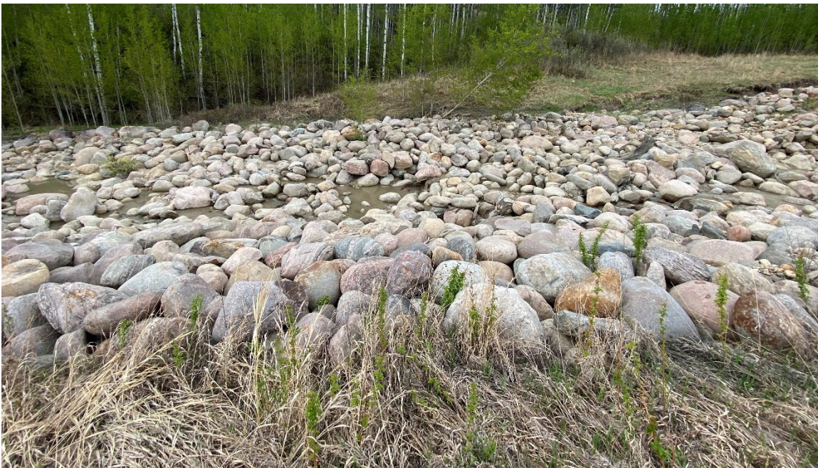
Photo 7-12.: Multiple areas with localized scour and riprap displacement were observed within the channel segment for an approximately 100 m length downstream of the lower drop structure (32+425). Majority of riprap was intact and there was no major erosional downcutting or washout.
