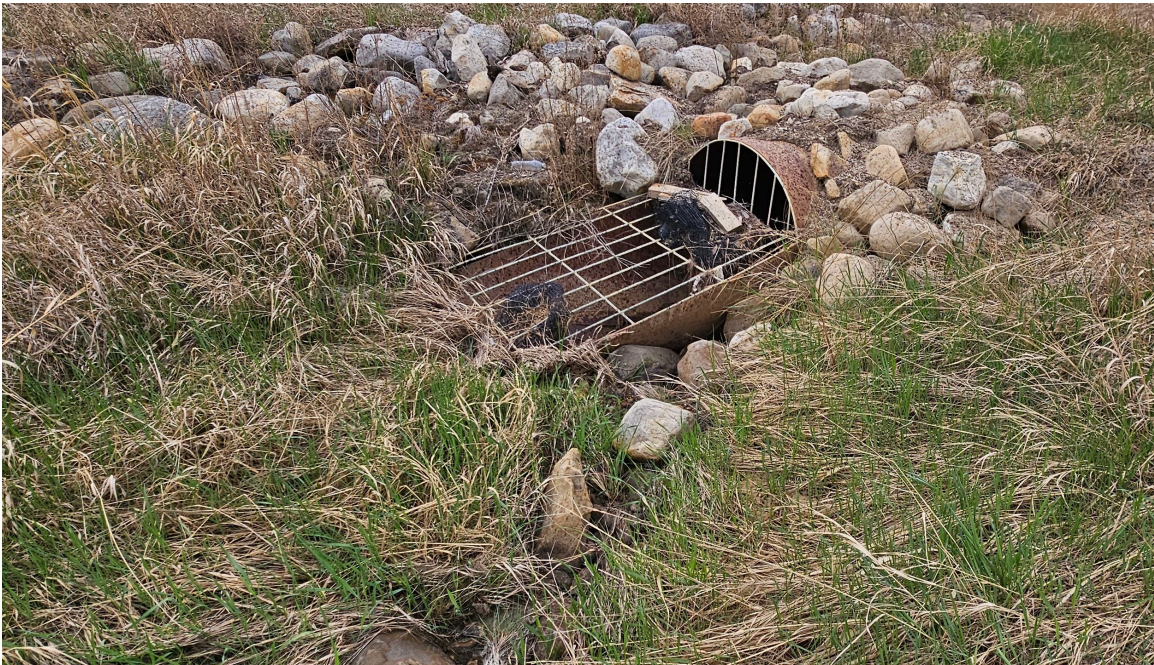
Photo 7-20.: Centreline culvert inlet at the south ditch near 32+050. Minor ditch erosion and partial flow beneath the culvert.
