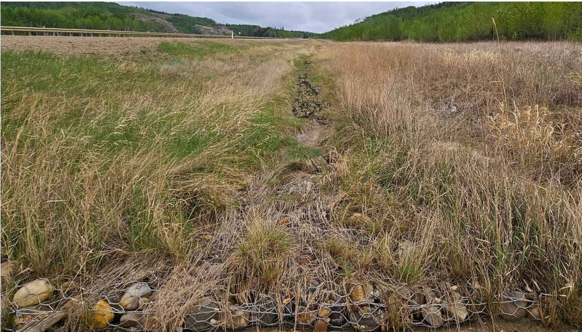
Photo 7-24.: Looking upslope the ditch (east) at the geoweb control section (32+400). No major change since the 2023 condition. Section had vegetation growth and some cells along the ditch bottom were only partially filled and broken.
