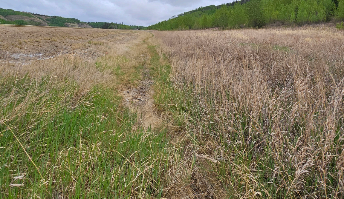
Photo 7-25.: Looking upslope the ditch (east) at the gabion mattress section (32+500). Section had vegetation growth and was performing well. Minor rill damage was noted on the north side of the ditch.
