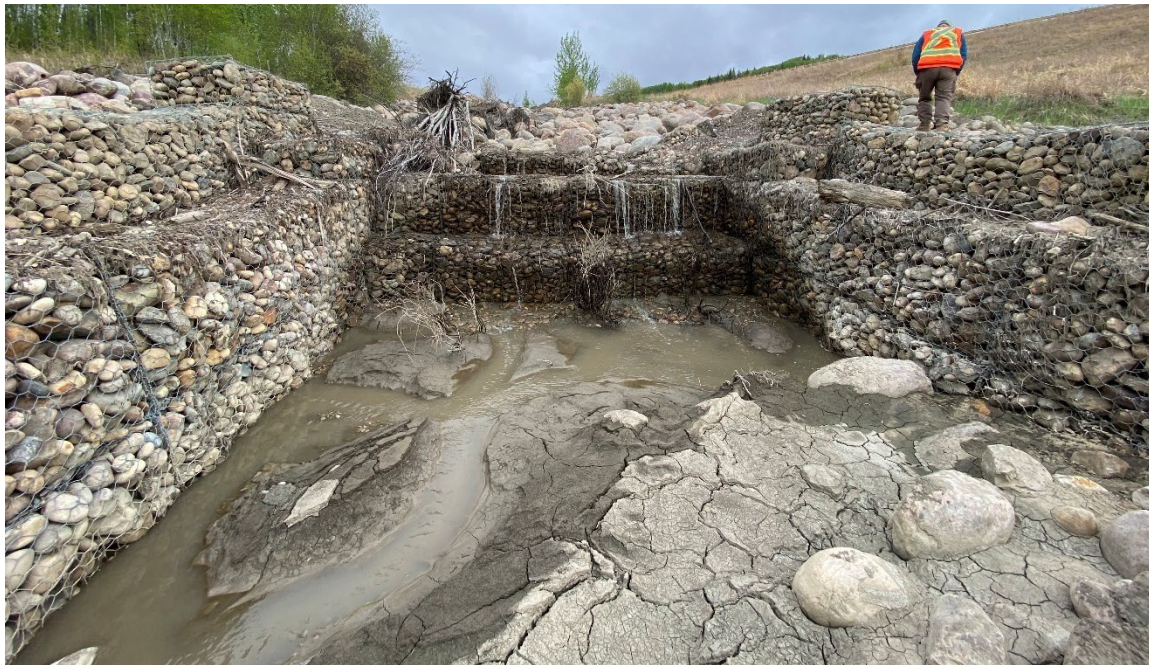
Photo 7-10.: View east towards the lower gabion drop structure (32+480). Minor basket deformation in the southeast inlet area. Debris and sediment buildup indicative of high flow around the outside of the structure with an erosion gully formed on the north side.
