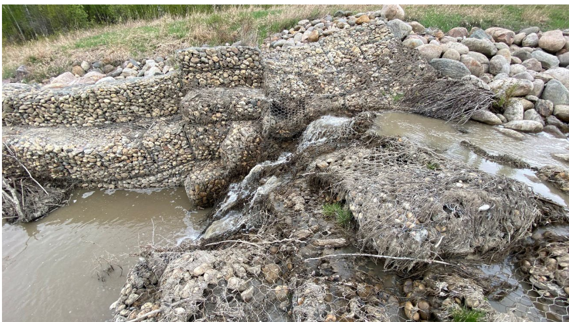
Photo 7-08.: View north towards the upper gabion drop structure (32+550). Major basket deformation and wire damage along channel centreline. Scour within the bottom of the structure has caused sag of the sidewalls. Sediment buildup and pooling in bottom.
