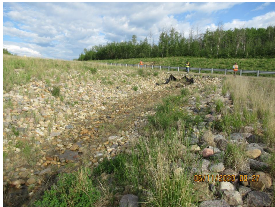
Photo 71-6. View of the armored swale at the culvert outlets (26+650). No issues were noted at the time of inspection.
