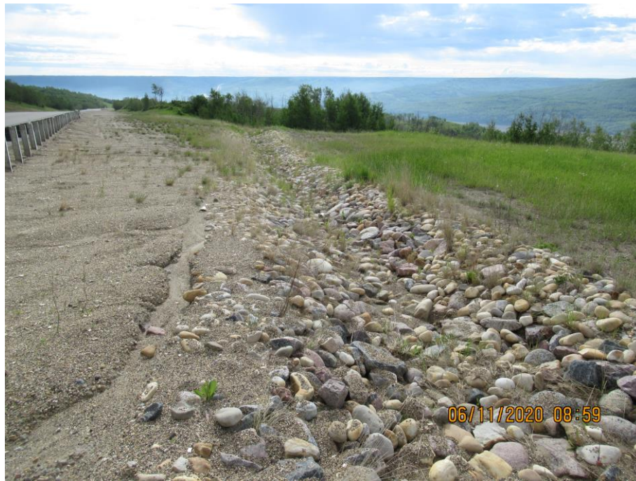
Photo 71-11. Looking towards the east at the east end of the pile wall at the armoured drainage swale. Minor rill erosion was observed between the swale and road edge in areas of poor vegetation.
