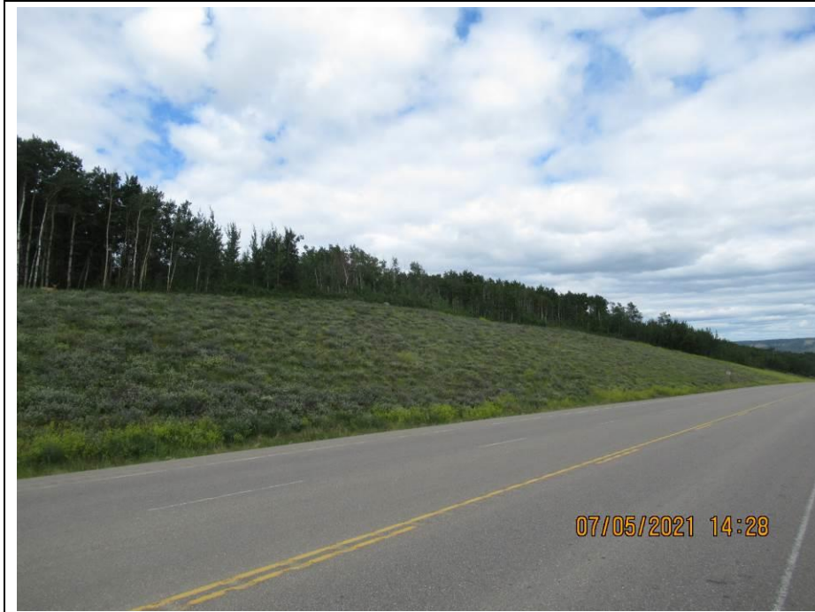
Photo 71-12. Looking northeast towards the backslope area across from the pile wall (26+800). Slope had good vegetation coverage and no issues were observed.
