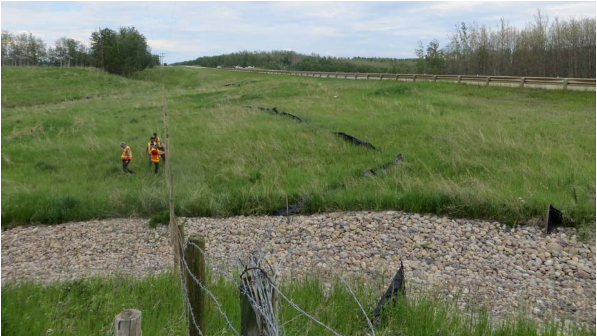
Photo 7 - Looking east along the south embankment slope from the west end.
