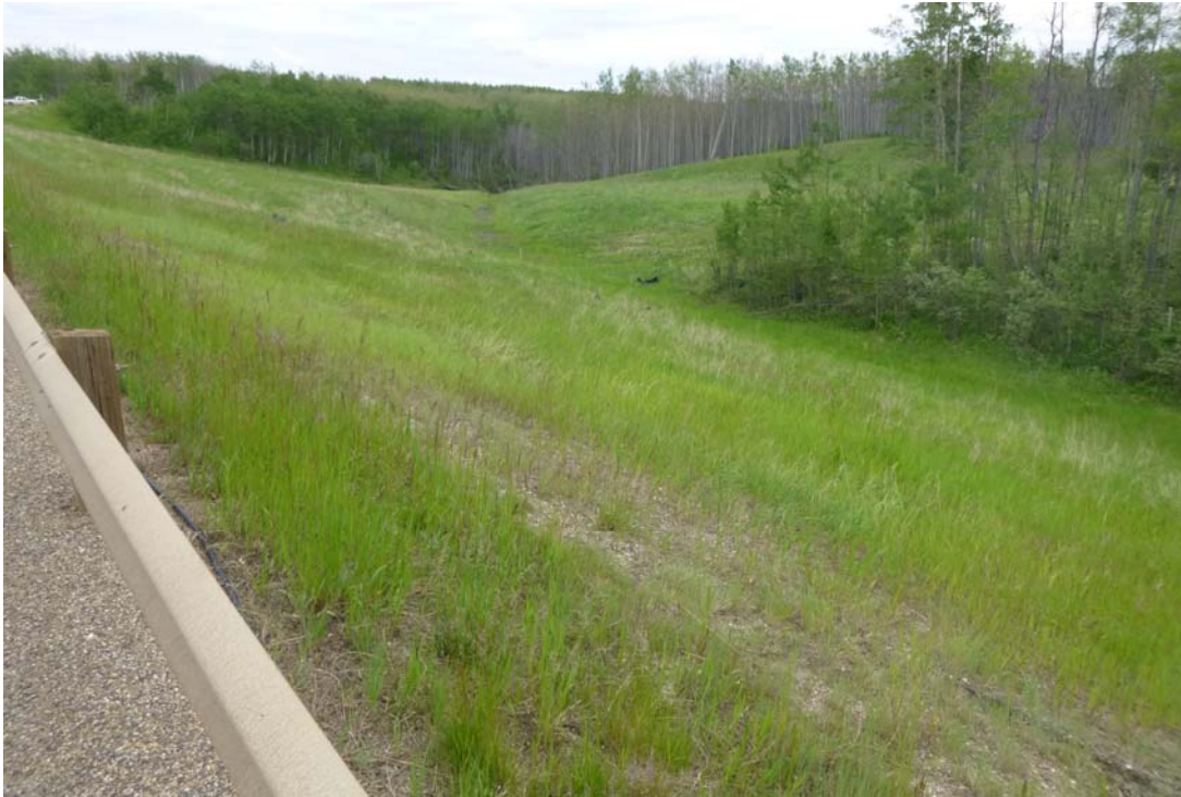
Photo 9 – Looking southeast along the south embankment slope from the west end.
