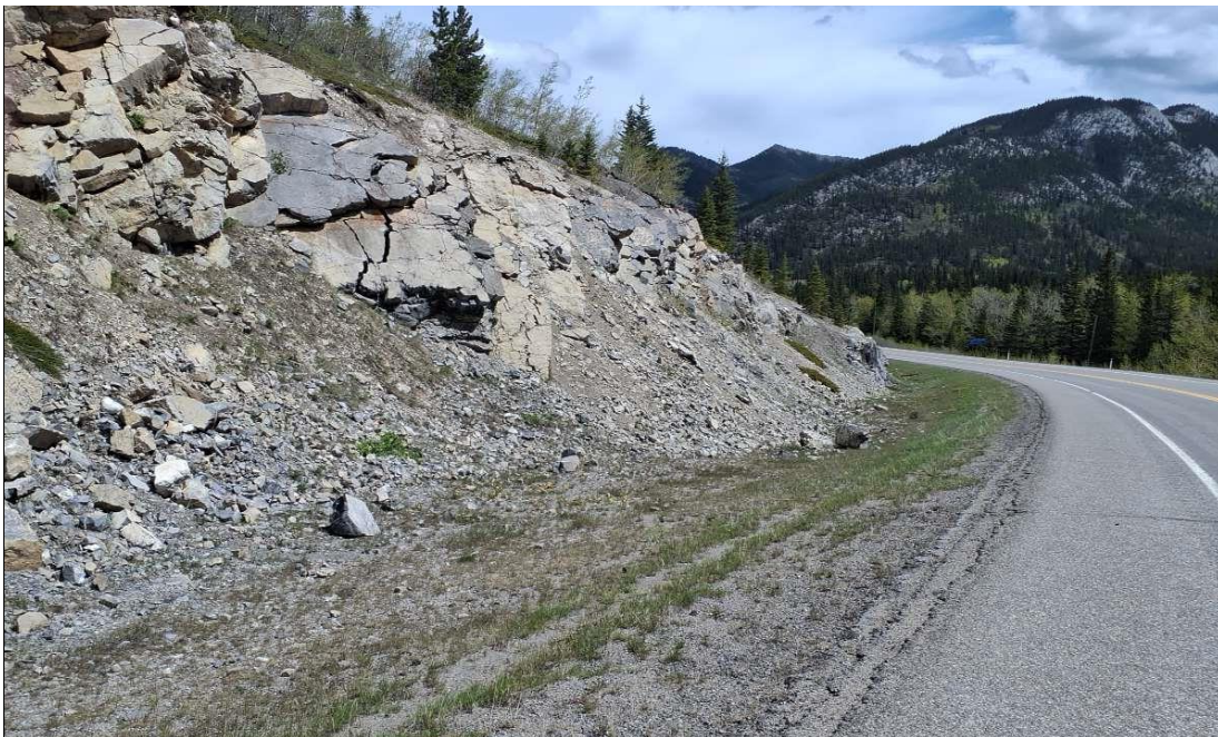
Photo 8 S070-III: Bedrock fracturing leading to future rockfall blocks. Large rock noted in ditch was there during the 2022 inspection. Photo taken facing southeast on May 28, 2024.
