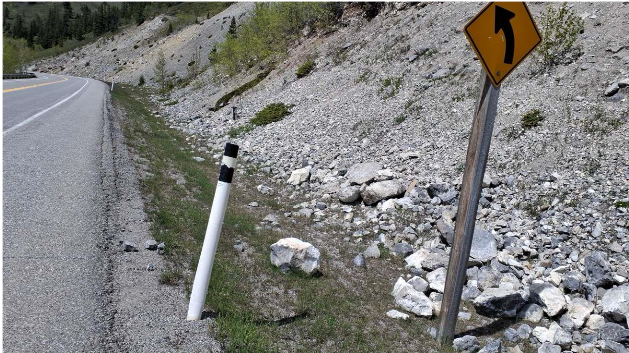
Photo 6 S070-III: Rockfall debris at the toe of the slope in northbound ditch. Photo taken facing northwest on May 28, 2024.
