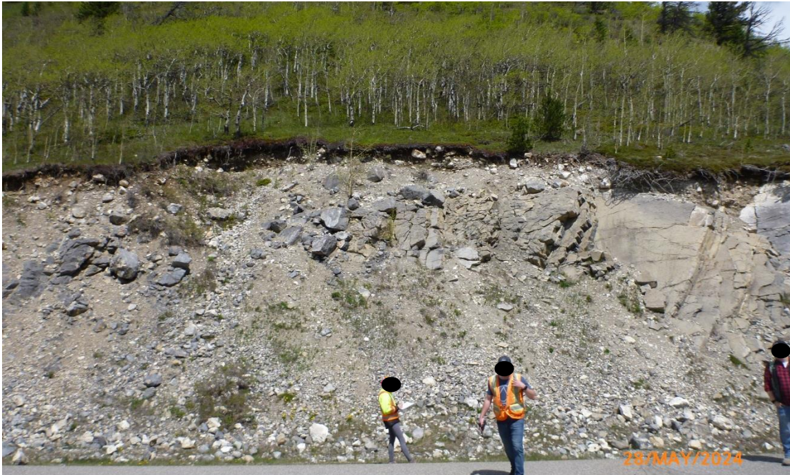
Photo 8 S070-III: Bedrock fracturing leading to future rockfall blocks. Large rock noted in ditch was there during the 2022 inspection. Photo taken facing southeast on May 28, 2024.
