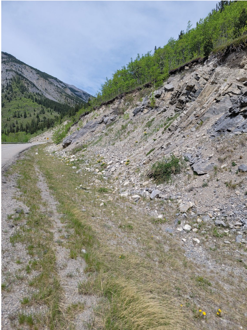
Photo 3 S070-3: Rockfall debris at the toe of the slope in northbound ditch. Photo taken facing northwest on May 27, 2025.
