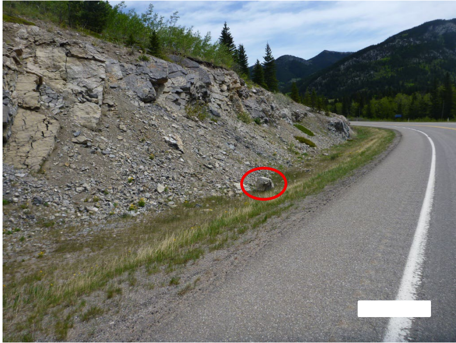
Photo 5 S070-3: Bedrock fracturing leading to future rockfall blocks. Large rock noted in ditch was since the 2022 inspection (red circle). Photo taken facing southeast on May 27, 2025.
