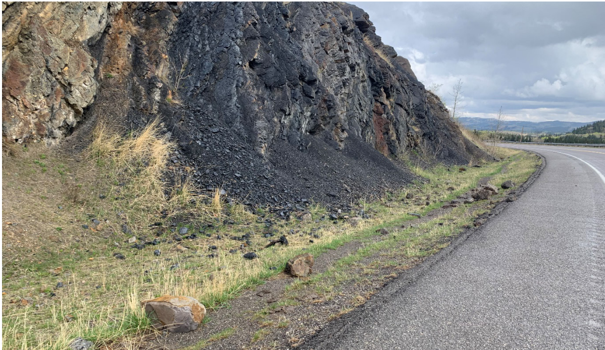
Photo 4 Large debris fan in central portion of the slope. Block adjacent to debris fan (indicated by red circle) is at risk of detaching. Photo taken May 9, 2023, facing north.
