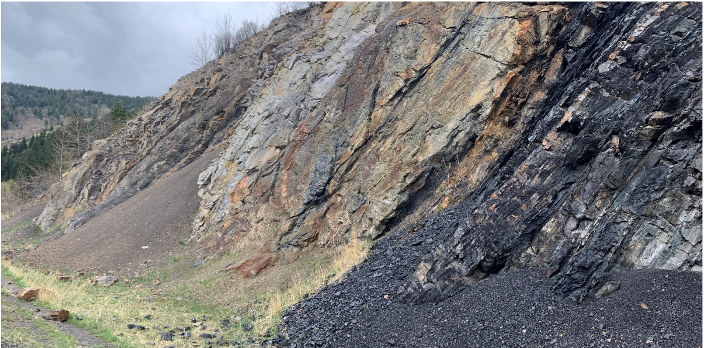
Photo 2 Rockfall material in the ditch and debris fan on the lower portion of the back slope. Photo taken May 9, 2023, facing northwest.
