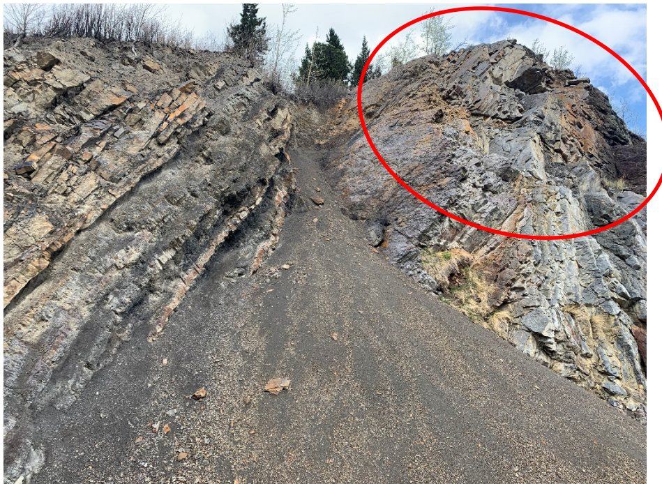
Photo 4 Large debris fan in central portion of the slope. Block adjacent to debris fan (indicated by red circle) is at risk of detaching. Photo taken May 9, 2023, facing north.
