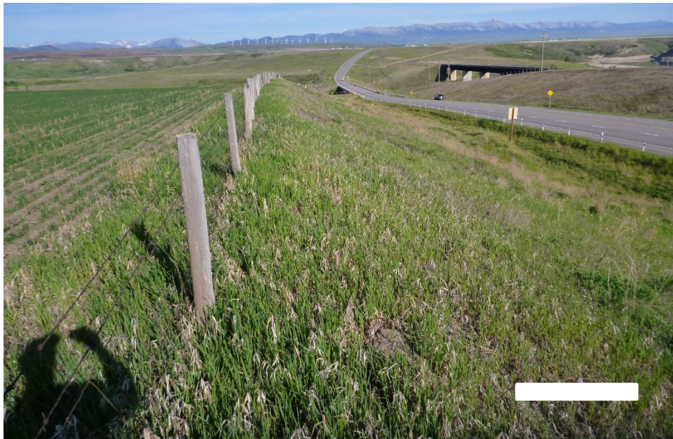
Photo 7 The slope outside of the site limits is even, well-vegetated, and is performing well. Photo taken May 28, 2025, facing west.
