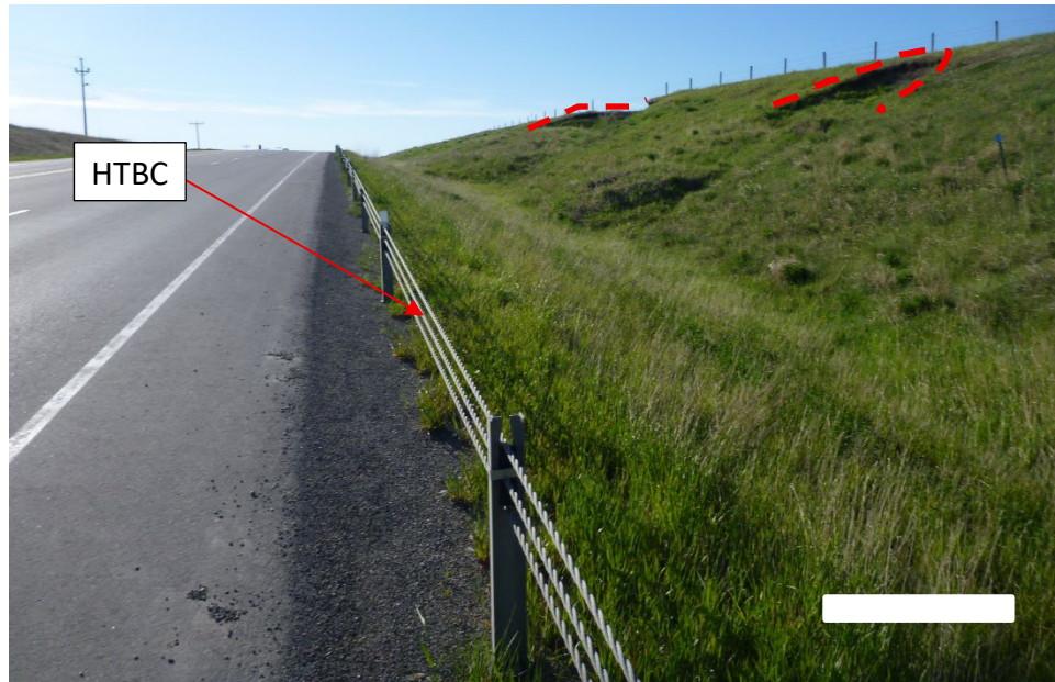
Photo 3 Failed material (red line) partially blocking south (eastbound) ditch. Photo taken May 28, 2025, facing east.
