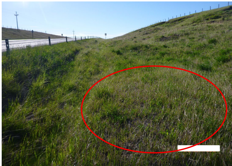
Photo 3 Failed material (red line) partially blocking south (eastbound) ditch. Photo taken May 28, 2025, facing east.
