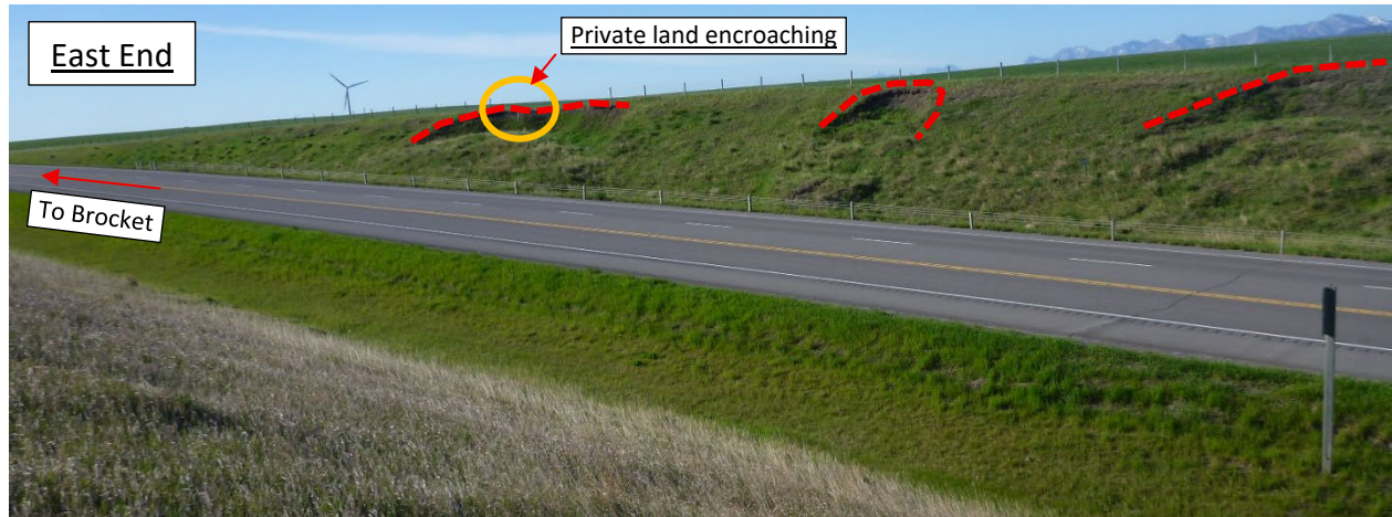
Photo 1 Panoramic view of multiple slides and head scarp (red dashed line) on the south backslope of the highway. Landslides encroaching private land (orange circle). Photos taken May 28, 2025, facing southwest.
