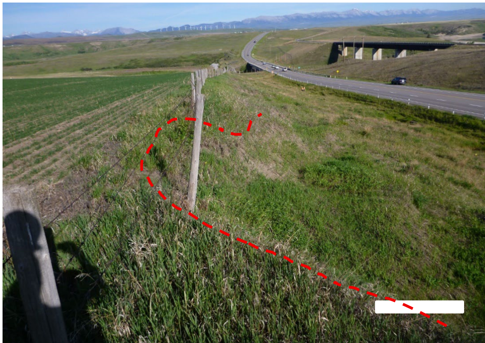
Photo 5 Head scarp (red dashed line) and private fence along the crest of the slope near the west end of the site. Photo taken May 28, 2025, facing west.
