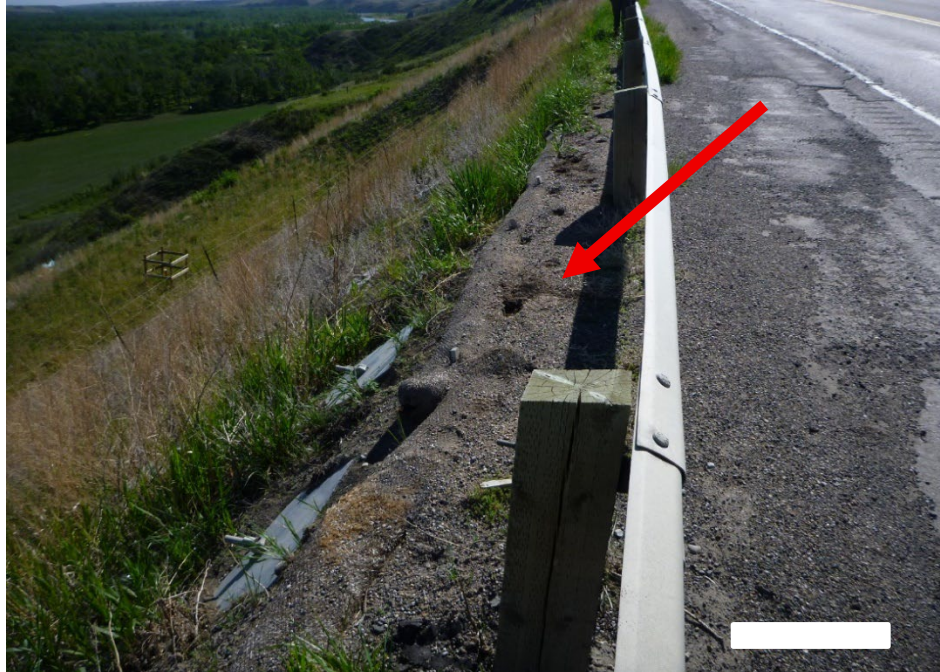
Photo 3 The slope is poorly vegetated, especially in the lower third of the slope. Photo taken May 28, 2025, facing west.
