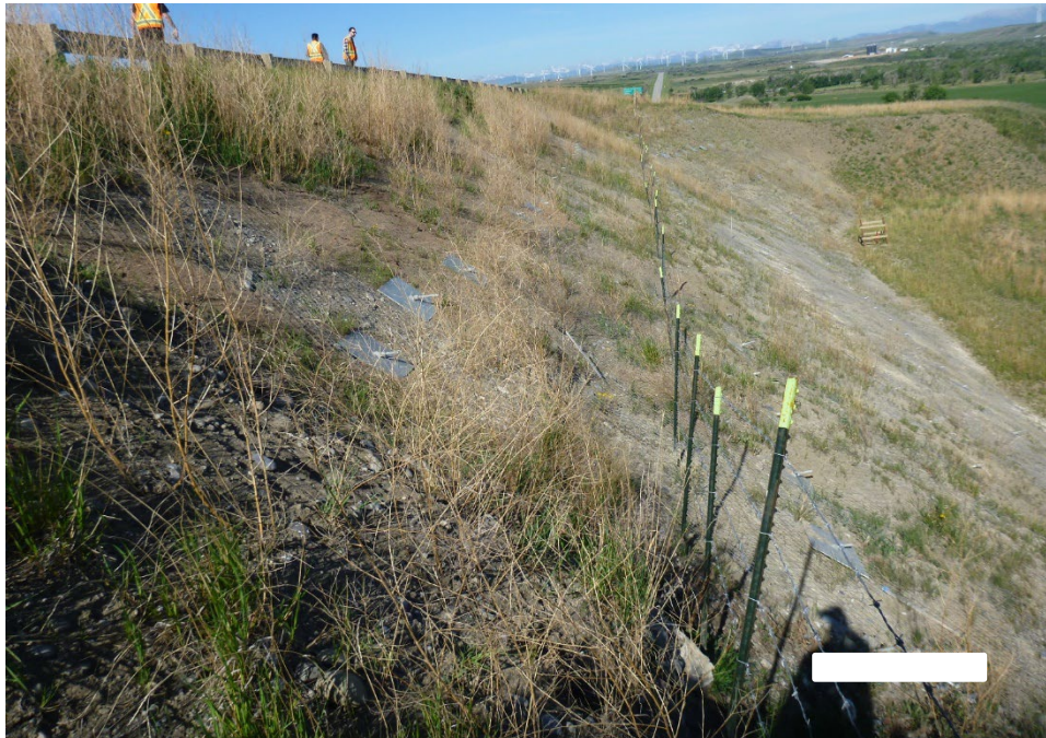
Photo 3 The slope is poorly vegetated, especially in the lower third of the slope. Photo taken May 28, 2025, facing west.
