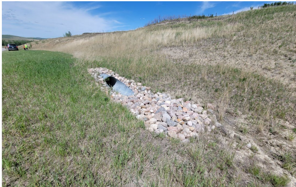
Photo 4 Culvert inlet and riprap apron installed in June 2021. Photo taken May 27, 2025, facing north.
