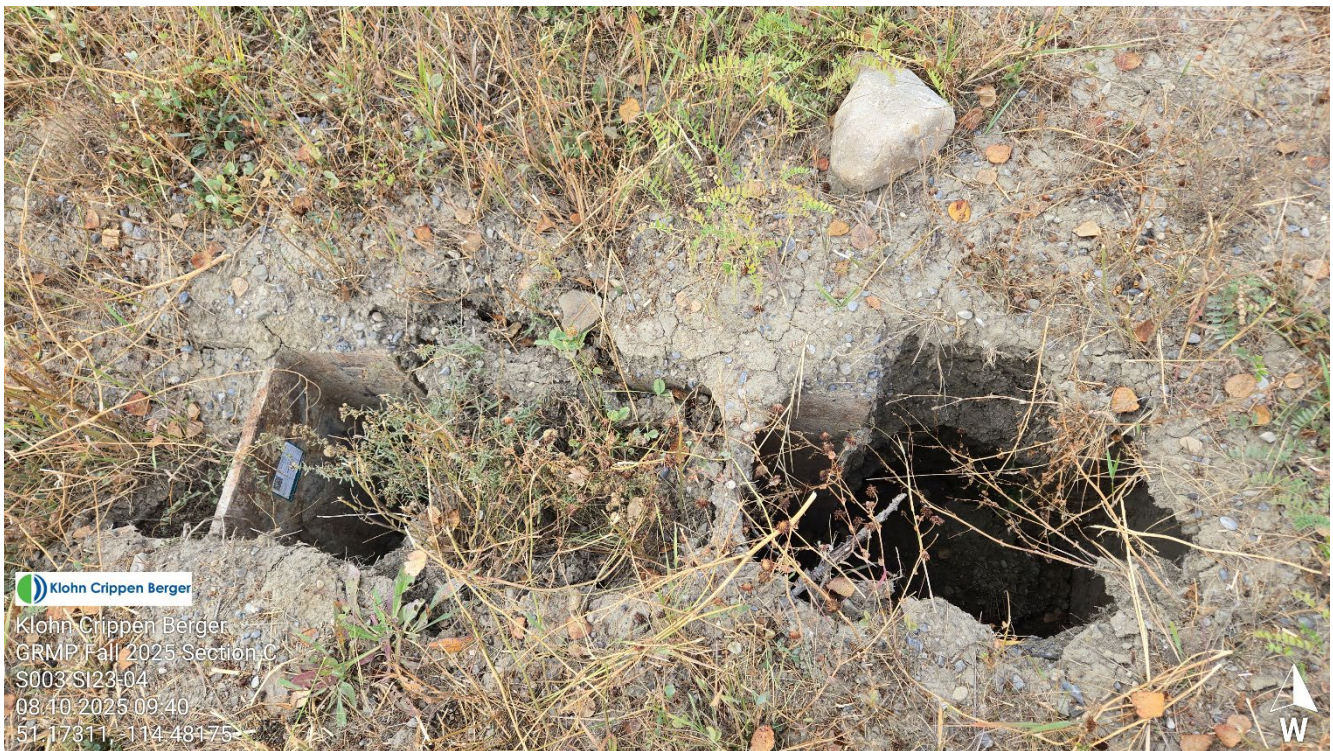
Photo 3.1 Sinkholes between piles of the H-Pile wall near SI23-04 casing.
