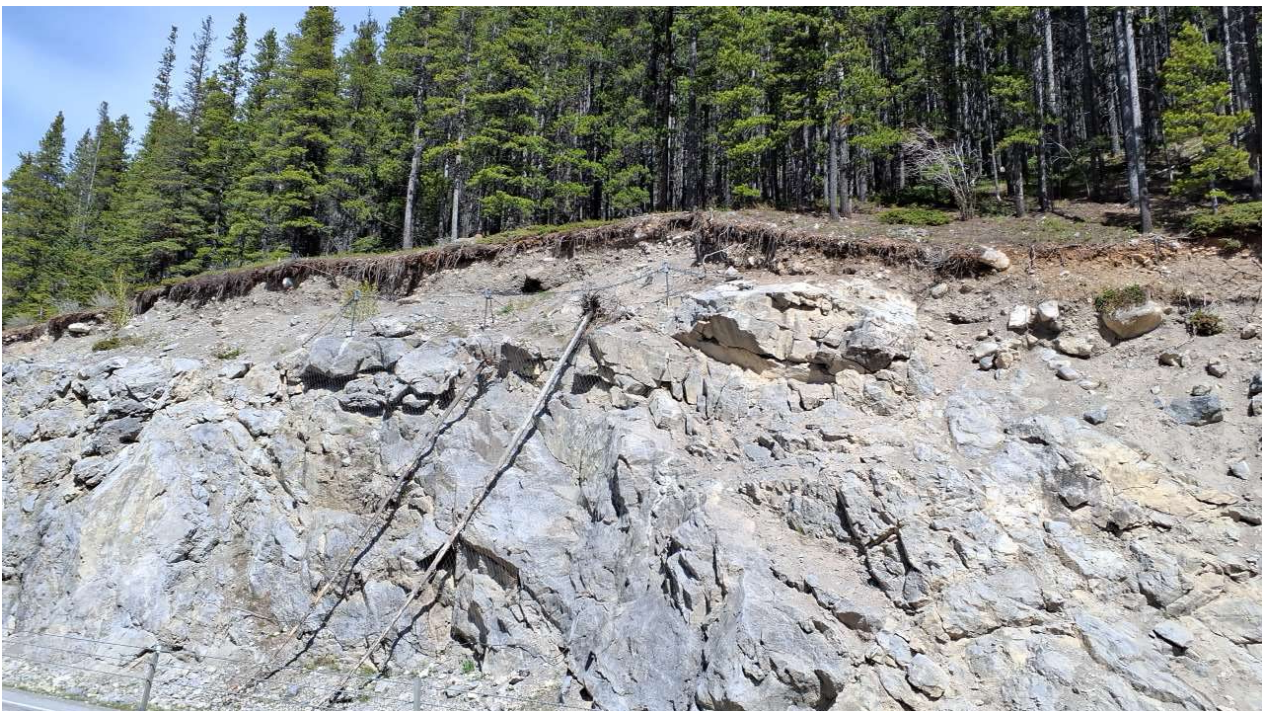
Photo 4 Erosion at brow of slope, above wire mesh depositing rock debris and trees. Photo taken May 27, 2024, facing east.
