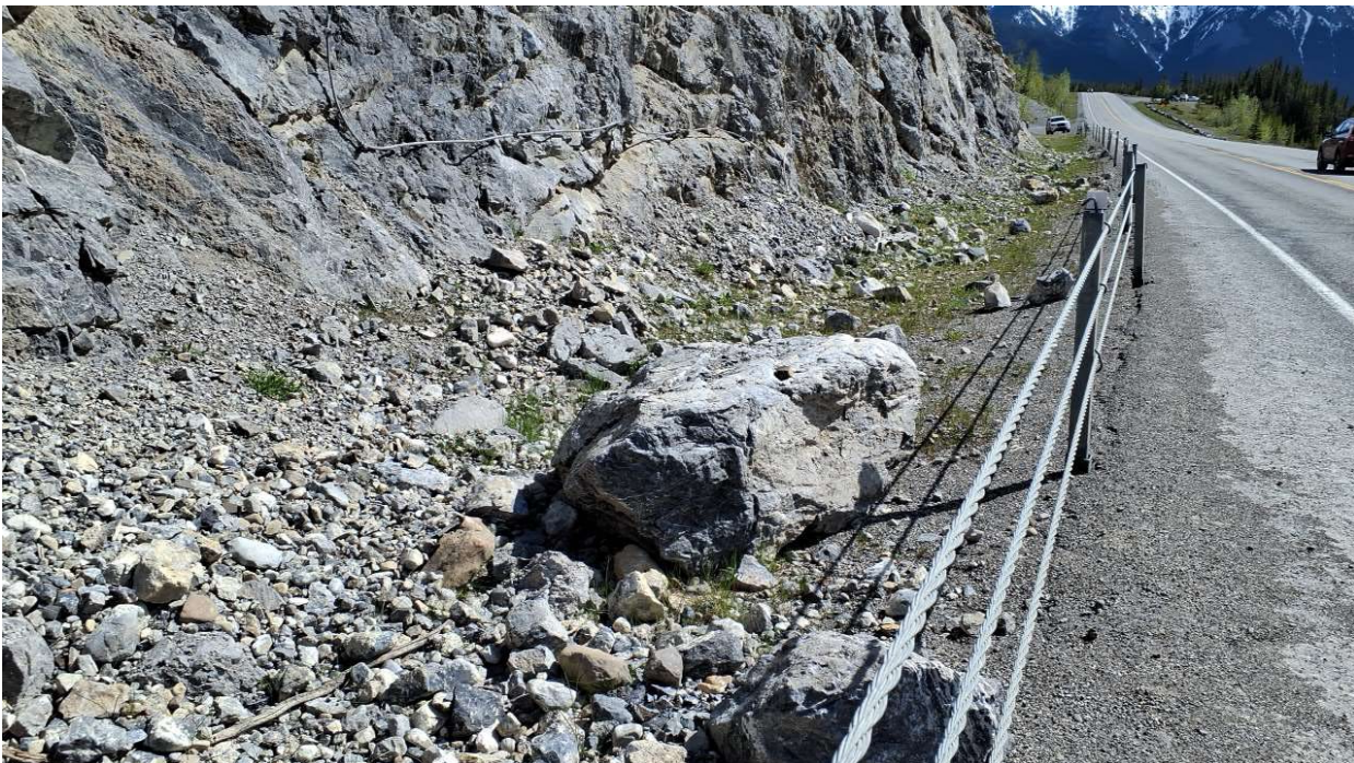
Photo 2 Rock debris in ditch up to 1.7 m x 1.2 m x 0.8 m. Large boulder was in the ditch during the previous inspection in 2019. More debris noted since last inspection. Photo taken facing south on May 27, 2024.
