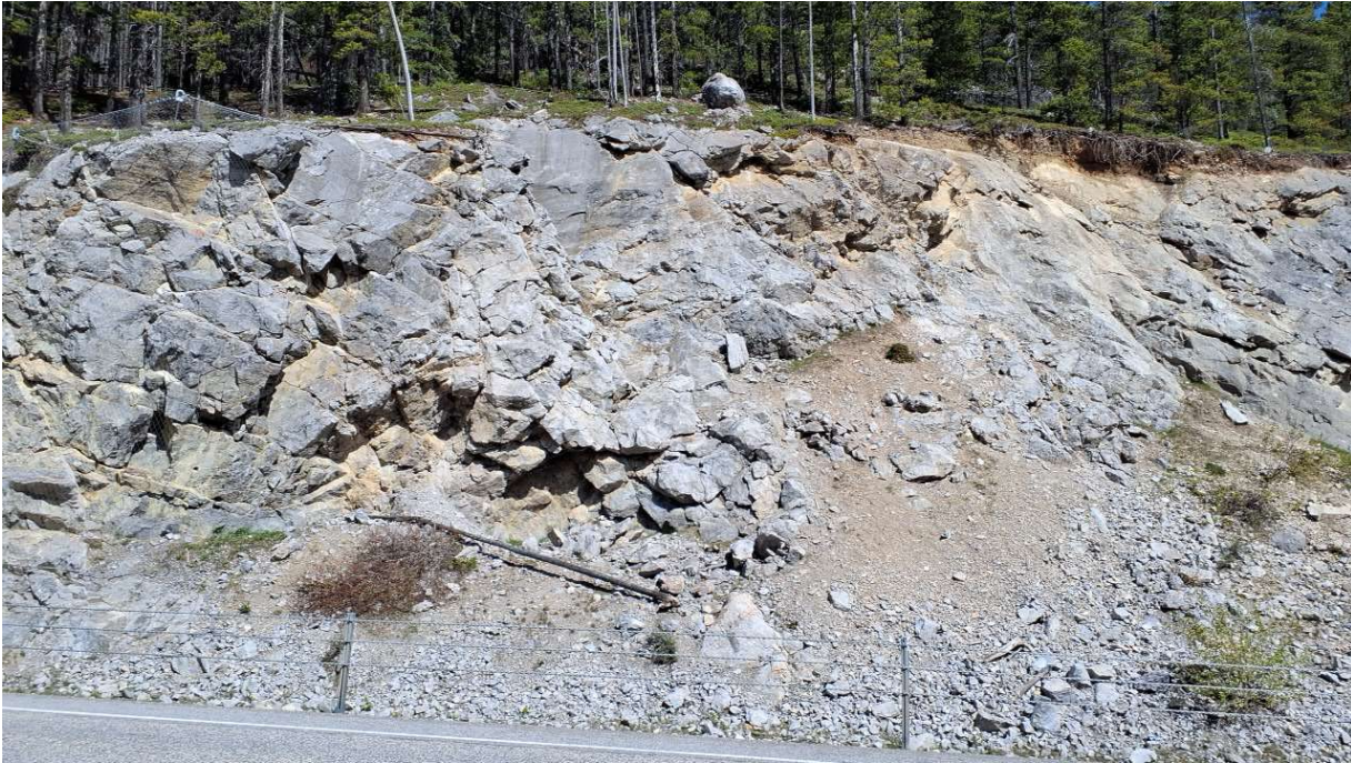
Photo 3 Rock mass dilated, with large blocks noted at the brow of the slope, outside of messed area. Photo taken May 27, 2024, facing east.
