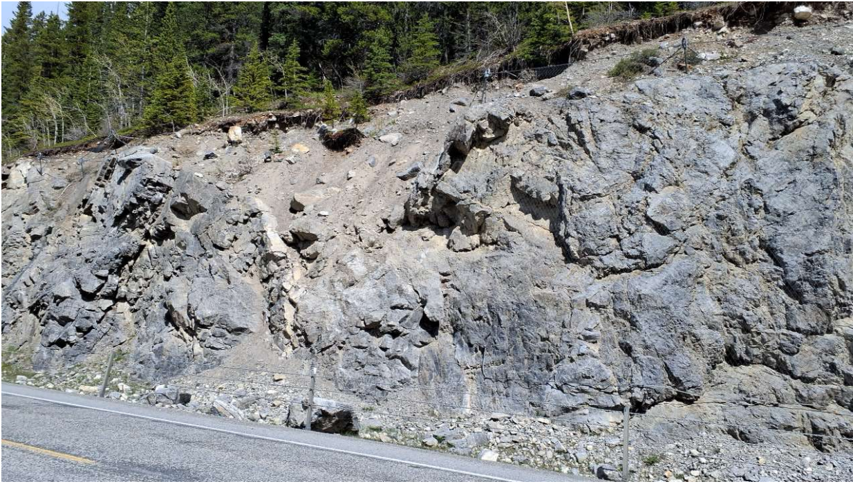
Photo 2 Rock debris in ditch up to 1.7 m x 1.2 m x 0.8 m. Large boulder was in the ditch during the previous inspection in 2019. More debris noted since last inspection. Photo taken facing south on May 27, 2024.
