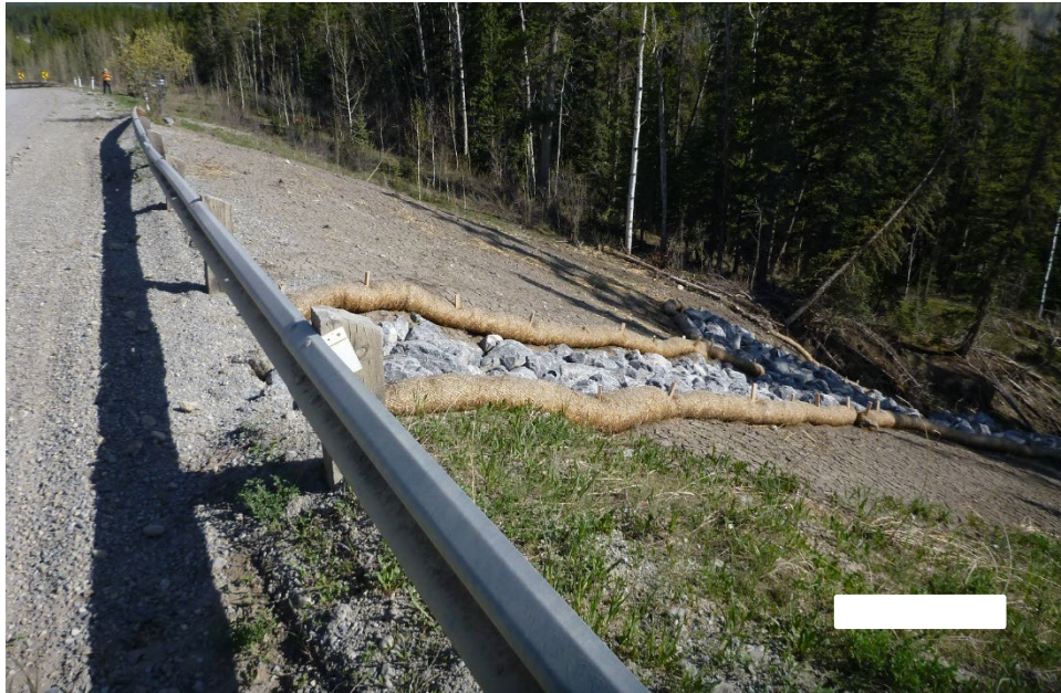
Photo 6 North check dam of cobbles and boulders at the culvert inlet. Photo taken May 26, 2025, facing northwest.
