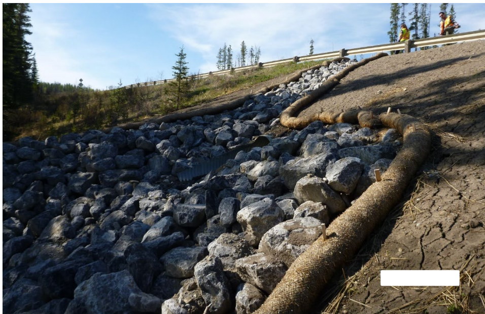
Photo 4 Straw wattles were installed around the riprap armoured channels as part of the 2024 construction. Photo taken May 26, 2025, facing south.
