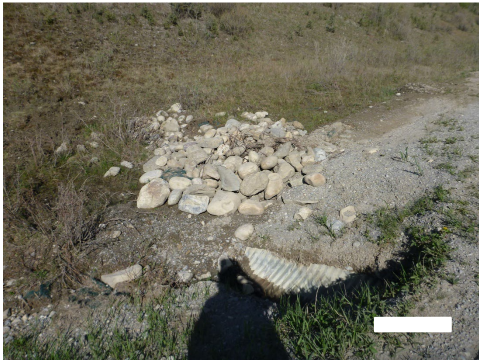
Photo 6 North check dam of cobbles and boulders at the culvert inlet. Photo taken May 26, 2025, facing northwest.
