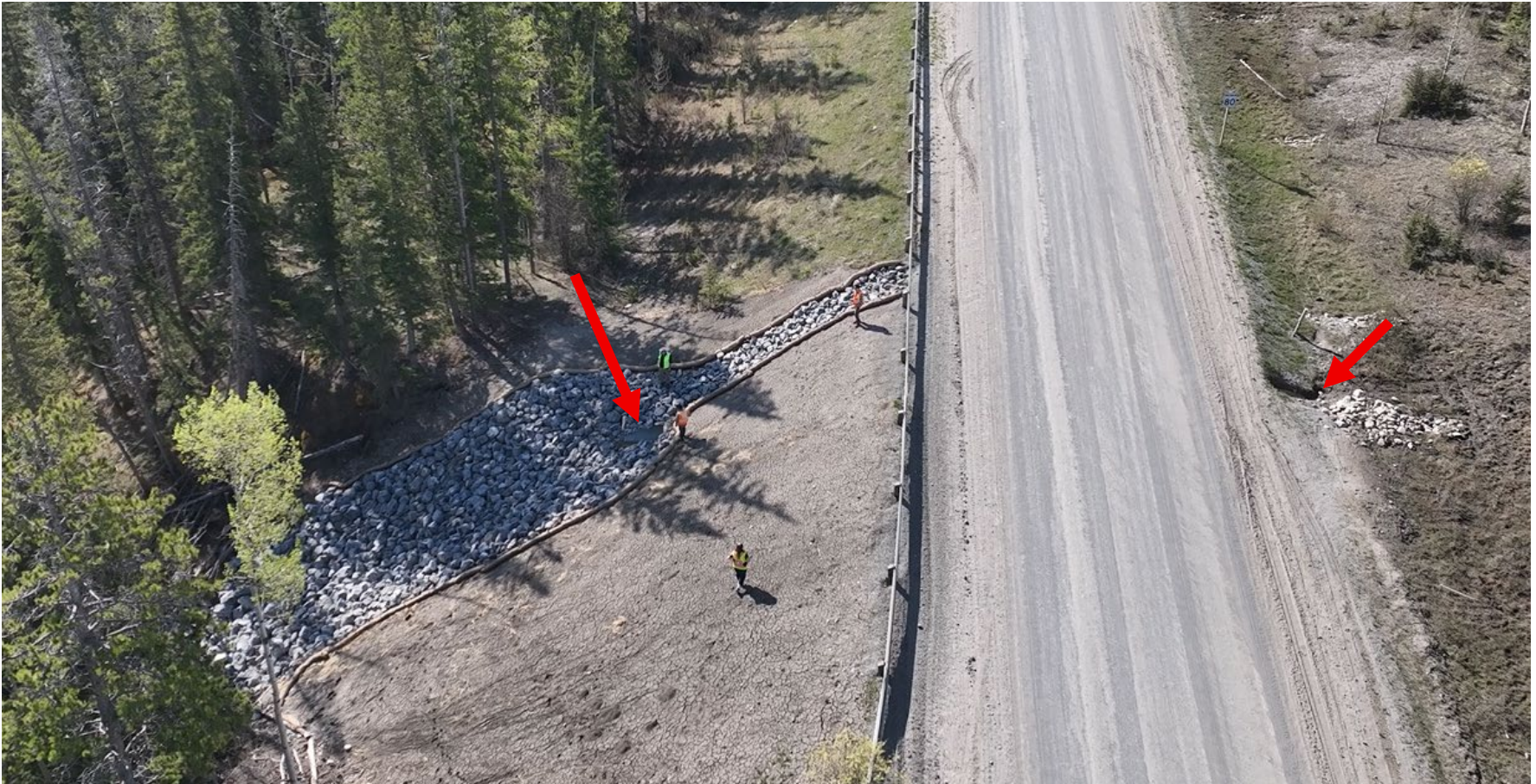
Photo 1 Aerial photo of the site showing the rebuilt slope, riprap armoured channels, and culvert outlet and inlet (indicated by red arrows). Photo taken May 26, 2025, facing southeast.
