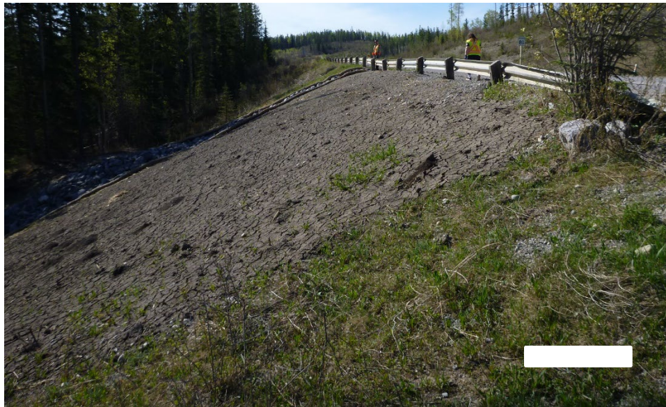
Photo 4 Straw wattles were installed around the riprap armoured channels as part of the 2024 construction. Photo taken May 26, 2025, facing south.
