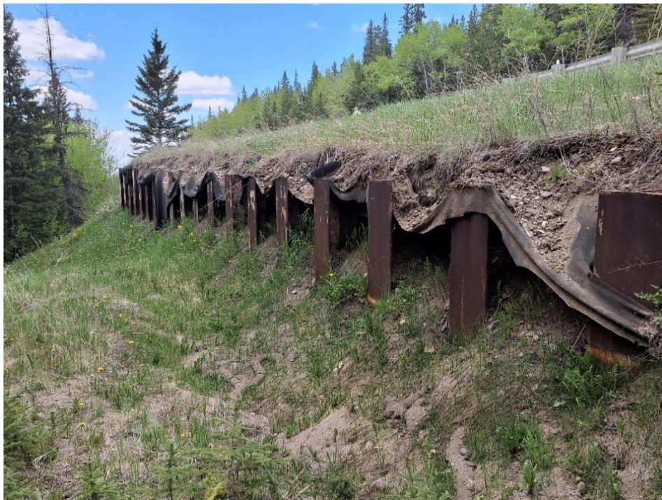
Photo 8 Exposed non-woven geotextile and upper portion of the H-piles. Photo taken May 28, 2025, facing northwest.
