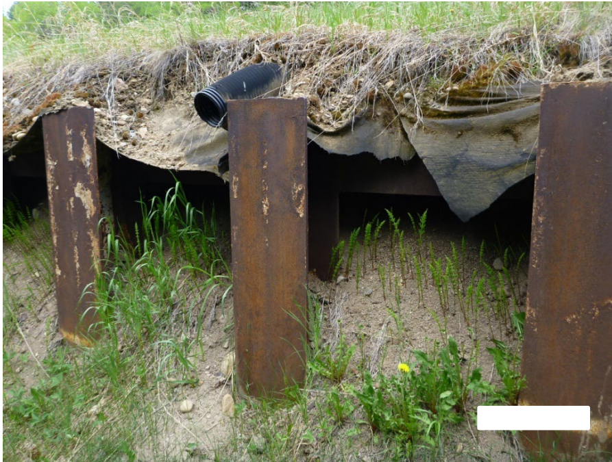
Photo 8 Exposed non-woven geotextile and upper portion of the H-piles. Photo taken May 28, 2025, facing northwest.
