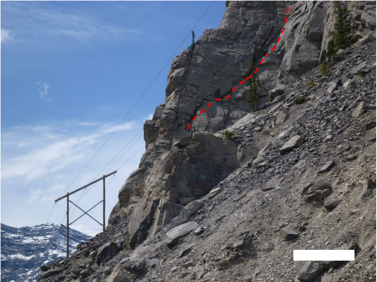
Photo 5 Pre-sheared joint set (red dashed line) located between the north and south side of the site. Photo taken May 26, 2025, facing south.
