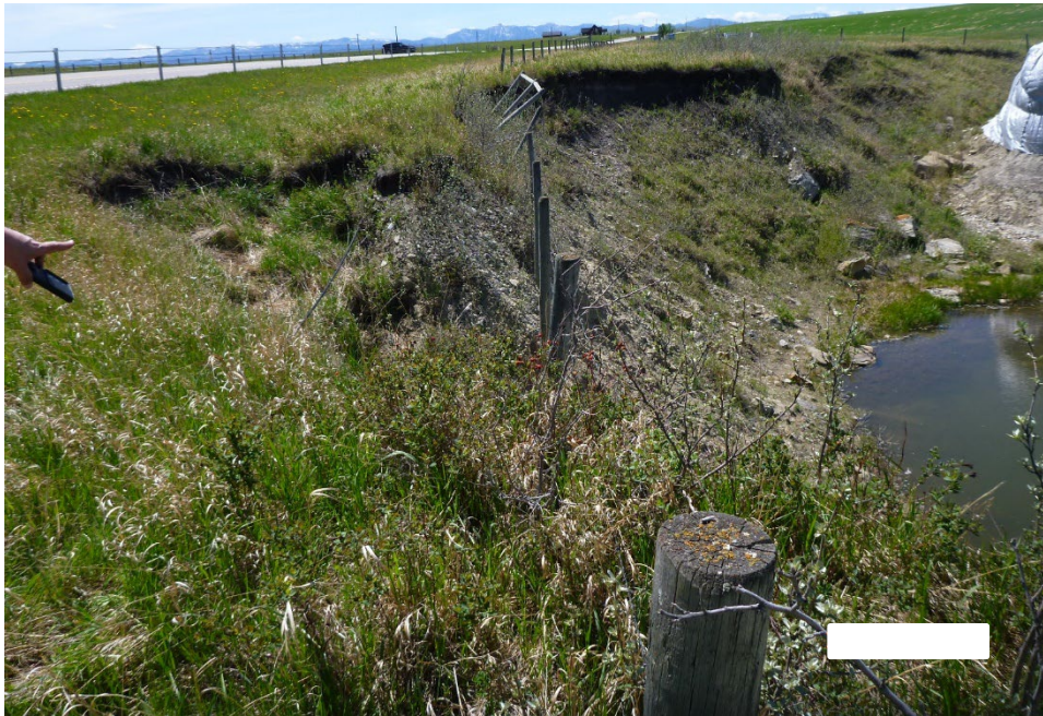
Photo 4 Erosion and hanging barbed wire fence along the site. Photo taken May 27, 2025, facing west.
