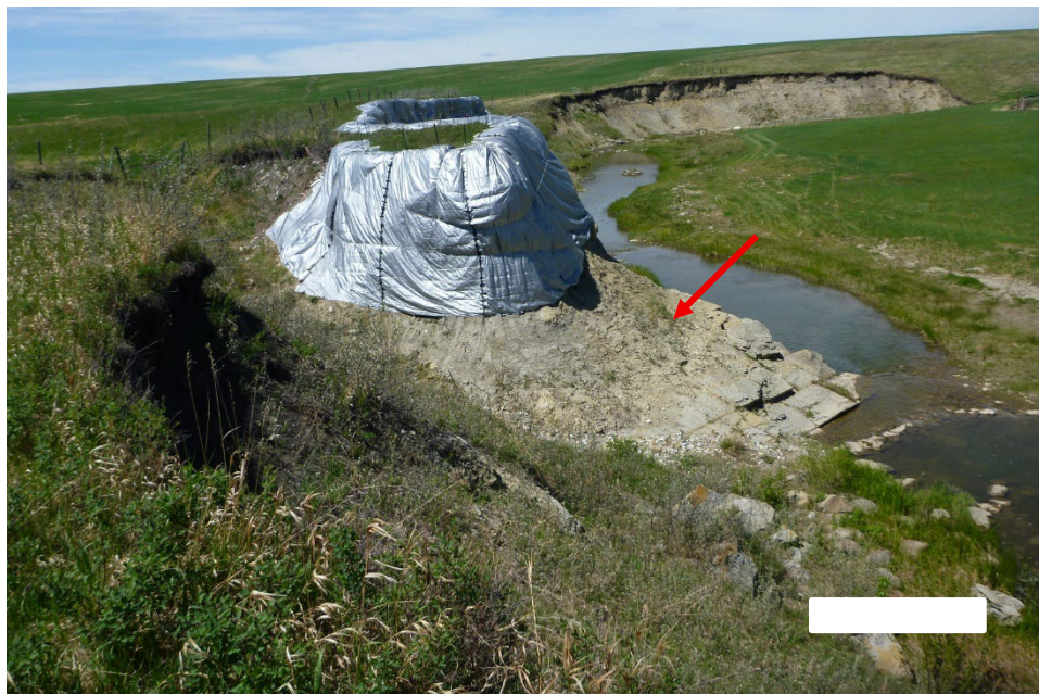
Photo 6 Tarps installed by KCB as part of the ongoing bank swallow mitigation measures. Bedrock outcrop at the toe of the slope indicated by red arrow. Photo taken May 27, 2025, facing northwest.
