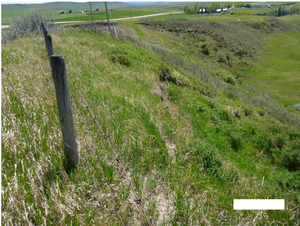
Photo 5 The slide at Site B is well vegetated and no deformation of the fence was observed. Photo taken May 27, 2025, facing south.
