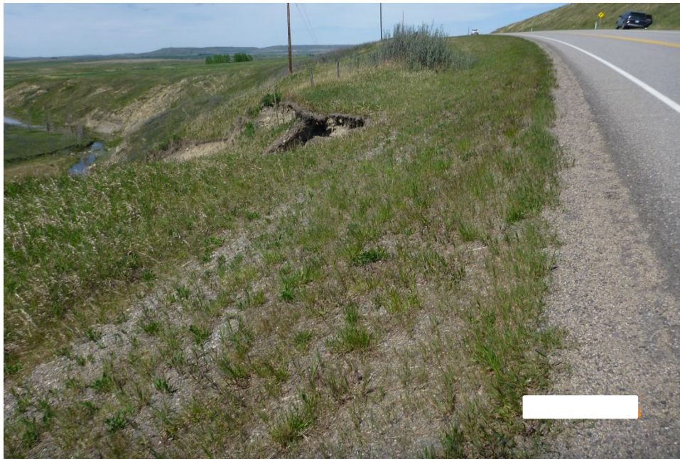
Photo 3 The ditch is well vegetated along Site A. The erosion of the head scarp near the north extent of the site is retrogressing towards the ditch/highway surface. Photo taken May 27, 2025, facing north.
