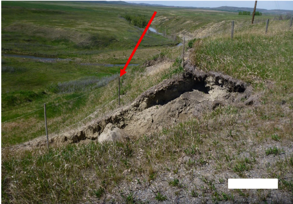
Photo 5 The slide at Site B is well vegetated and no deformation of the fence was observed. Photo taken May 27, 2025, facing south.
