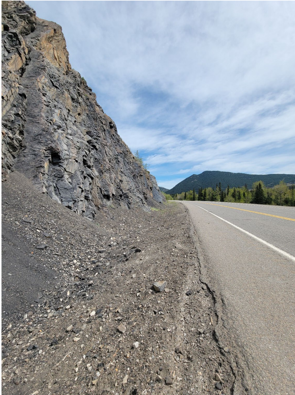
Photo 3 Active rockfall - debris fans and small rocks in the ditch towards the east end of the site. Photo taken facing east on May 27, 2025.
