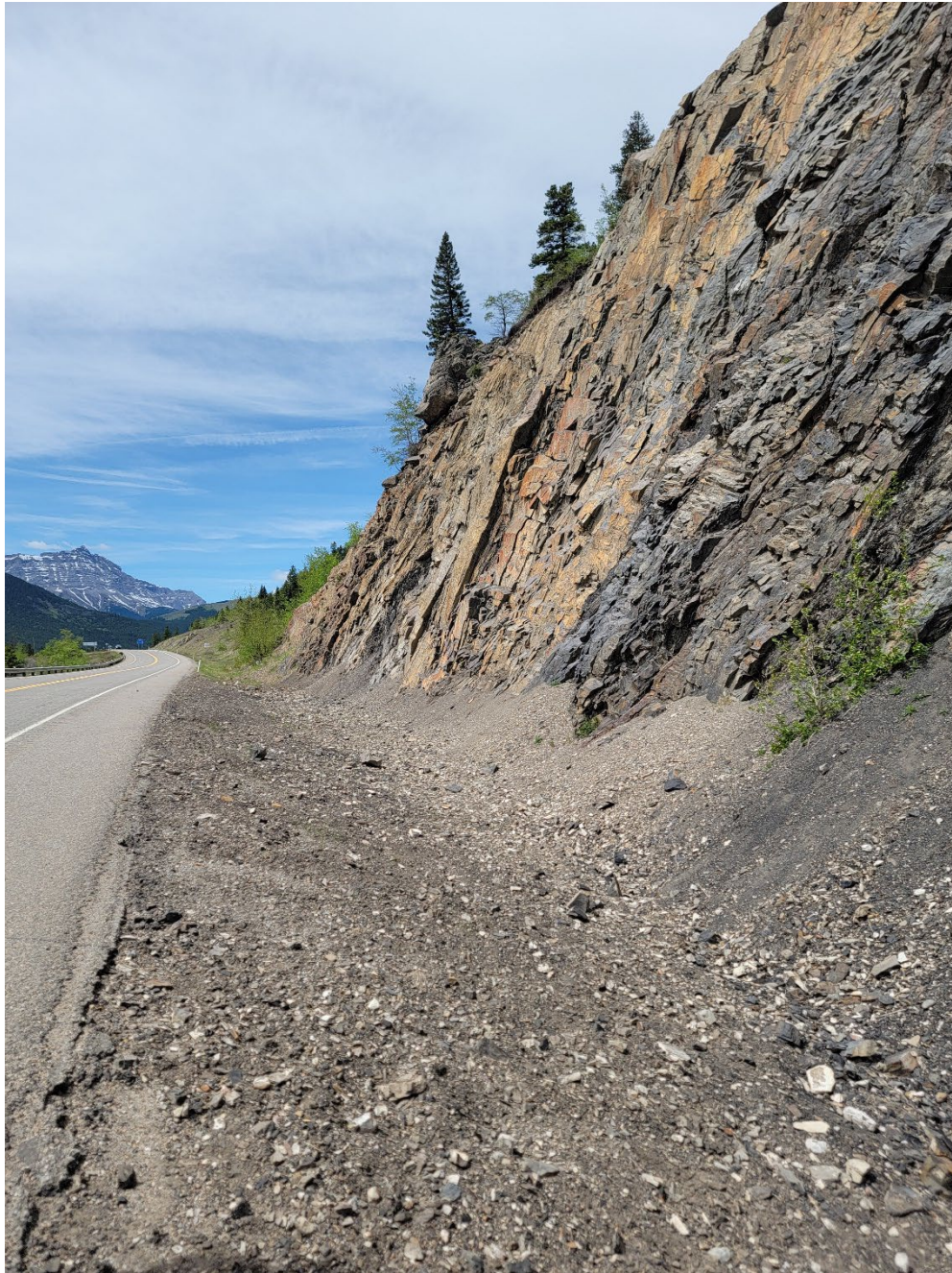
Photo 2 Active rockfall - debris fans and small rocks in the ditch towards the west end of the site. Photo was taken facing north on May 27, 2025.
