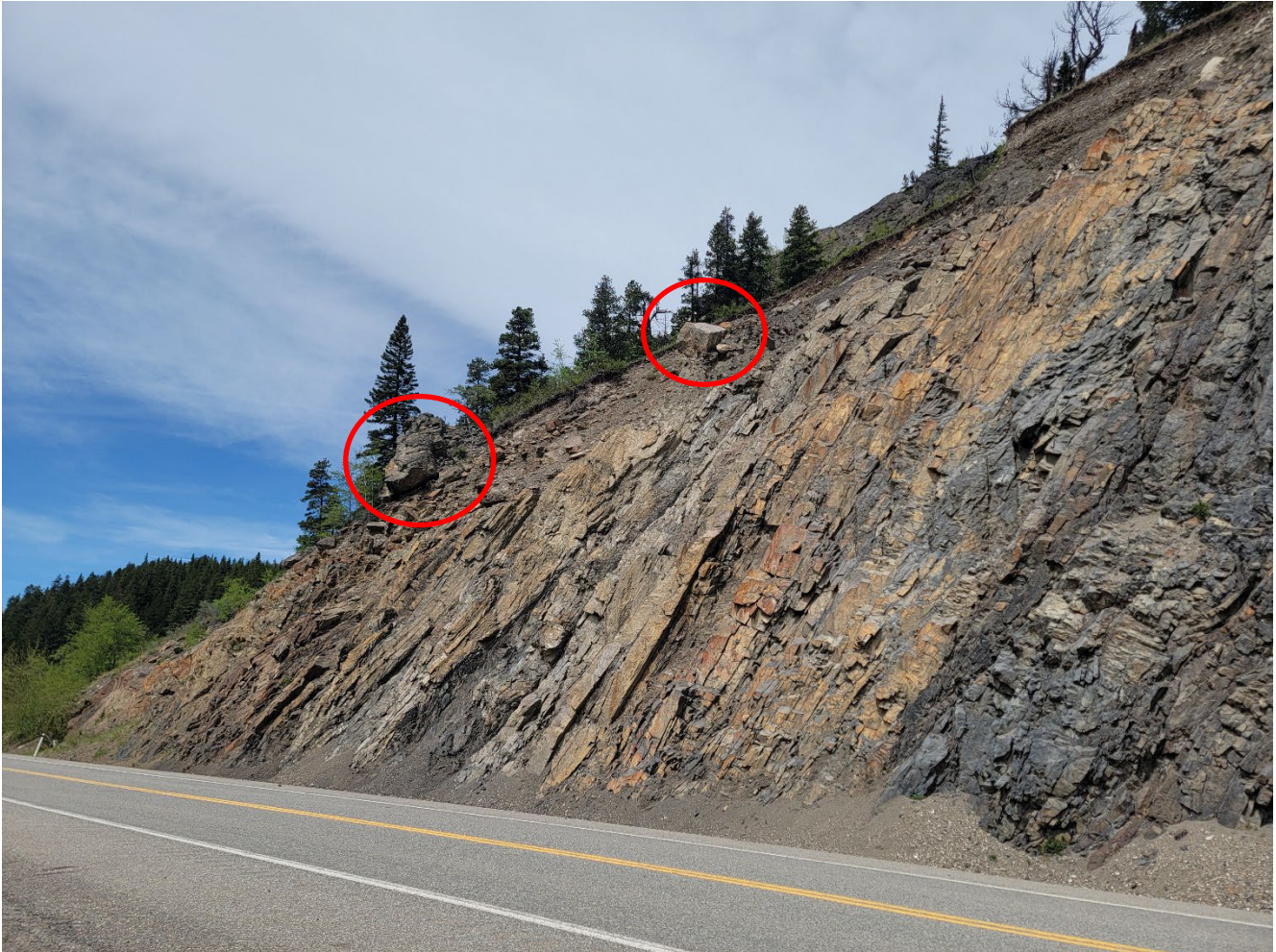
Photo 1 Rock slope cut with a vertical height of about 35 metres, featuring continuous joints and extensive soil erosion at the brow on the west side of the site. Also note the large overhang at the crest of the slope on the west end of the site. Photo was taken facing north on May 27, 2025.
