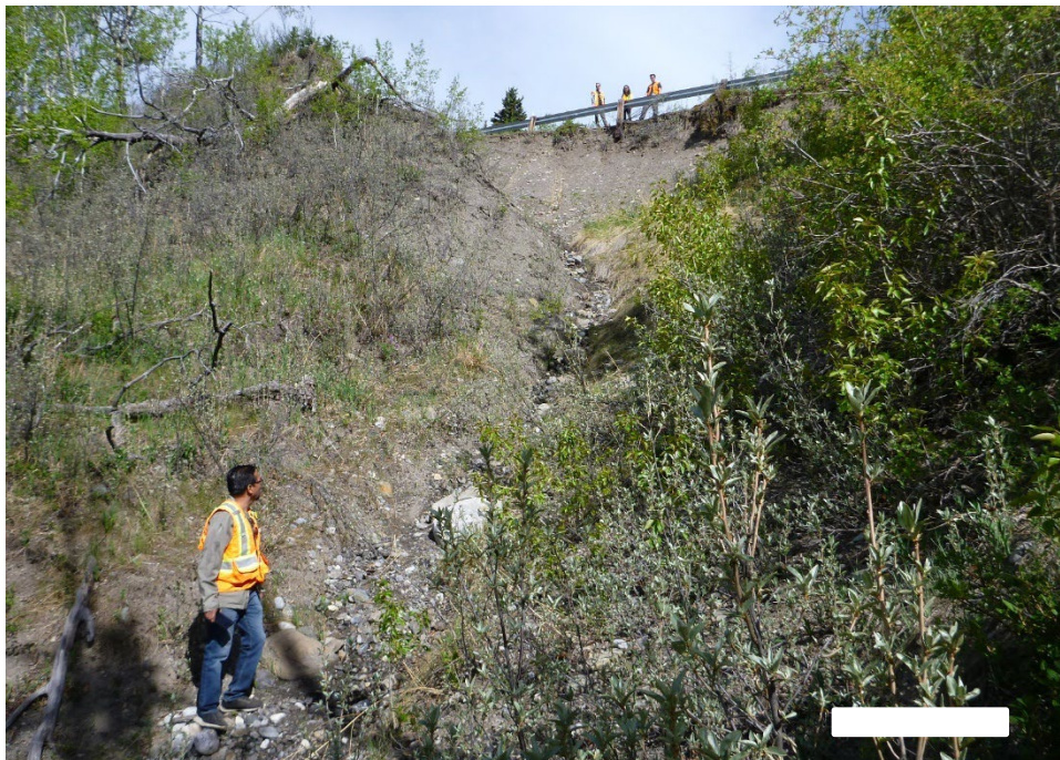
Photo 6 Midslope extent of the erosion where the erosion feature narrows to approximately 3 m to 5 m wide. A relatively shallow erosion gully extends downstream towards Sheep River. Photo taken May 27, 2025, facing north.
