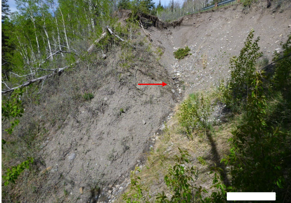
Photo 4 Erosion as viewed from the edge of the south lane. Photo taken May 27, 2025, facing south.
