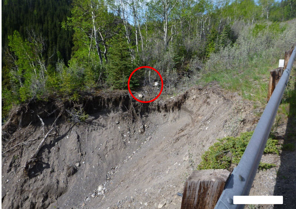
Photo 8 North backslope near the west extent of the site. No evidence of shallow bedrock was observed. Photo taken May 27, 2025, facing west.
