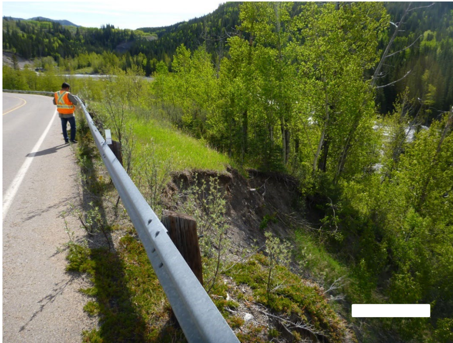
Photo 6 Midslope extent of the erosion where the erosion feature narrows to approximately 3 m to 5 m wide. A relatively shallow erosion gully extends downstream towards Sheep River. Photo taken May 27, 2025, facing north.
