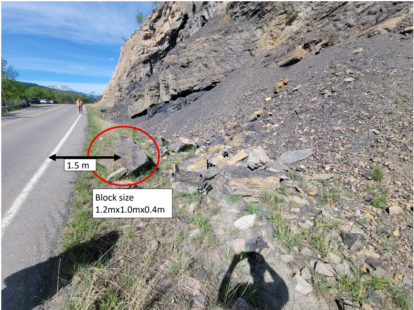
Photo 4 Large rock block in the ditch on the north side of the highway, which was also observed in the 2024 Inspection. Photo taken facing west on May 27, 2025.
