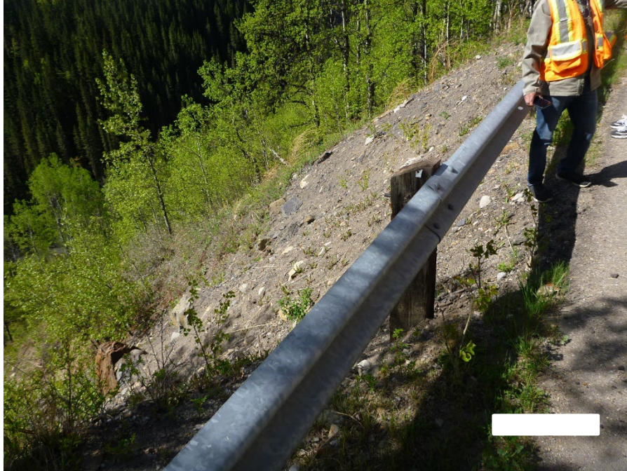
Photo 6 Surface runoff erosion on the south side of highway has undermined the guardrail and reached the pavement edge. There was no evidence of pavement cracks during the 2024 and 2025 inspections. Photo taken facing southeast on May 27, 2025.
