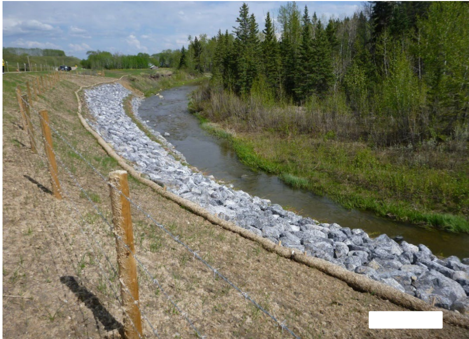
Photo 6 The crest of the slope between the HTCB and barbed wire fence was relatively smooth, and grass was growing on the slope. Photo taken May 26, 2025, facing east.
