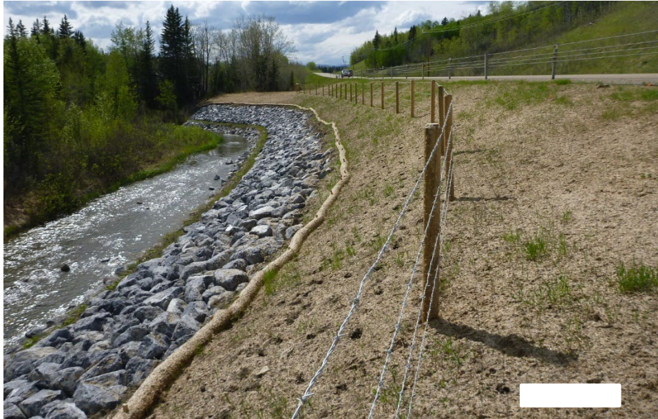
Photo 4 The west extent of the S045-1 site. The riprap appeared to be well-placed, and the brush layer appeared to be growing well during the inspection. Photo taken May 26, 2025, facing west.
