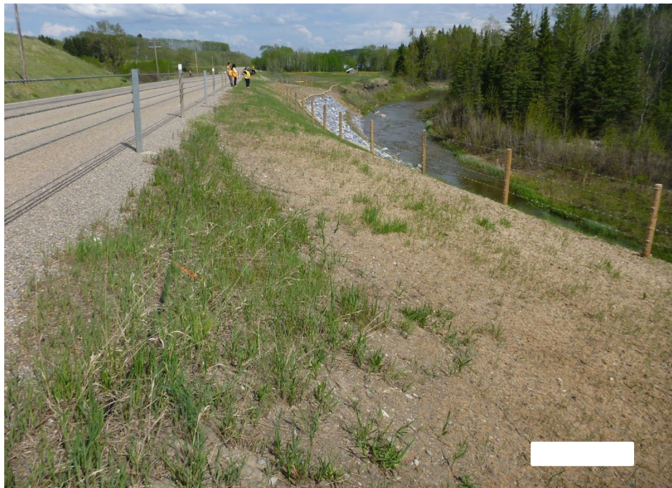
Photo 6 The crest of the slope between the HTCB and barbed wire fence was relatively smooth, and grass was growing on the slope. Photo taken May 26, 2025, facing east.
