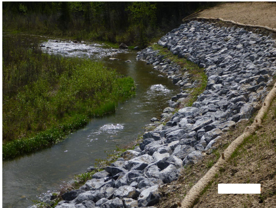
Photo 4 The west extent of the S045-1 site. The riprap appeared to be well-placed, and the brush layer appeared to be growing well during the inspection. Photo taken May 26, 2025, facing west.
