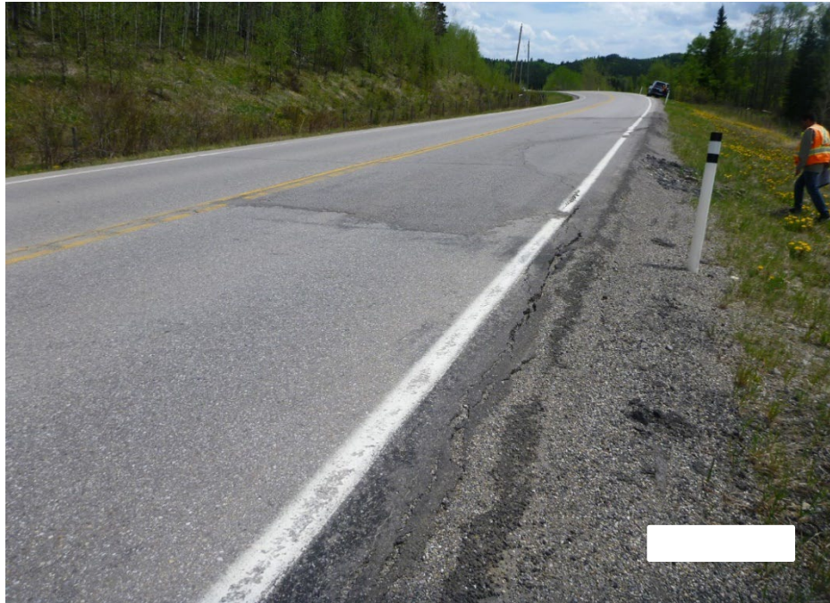
Photo 3 The west (southbound) highway embankment below the area of pavement distress (cracking and settlement). Photo taken May 26, 2025, facing north.
