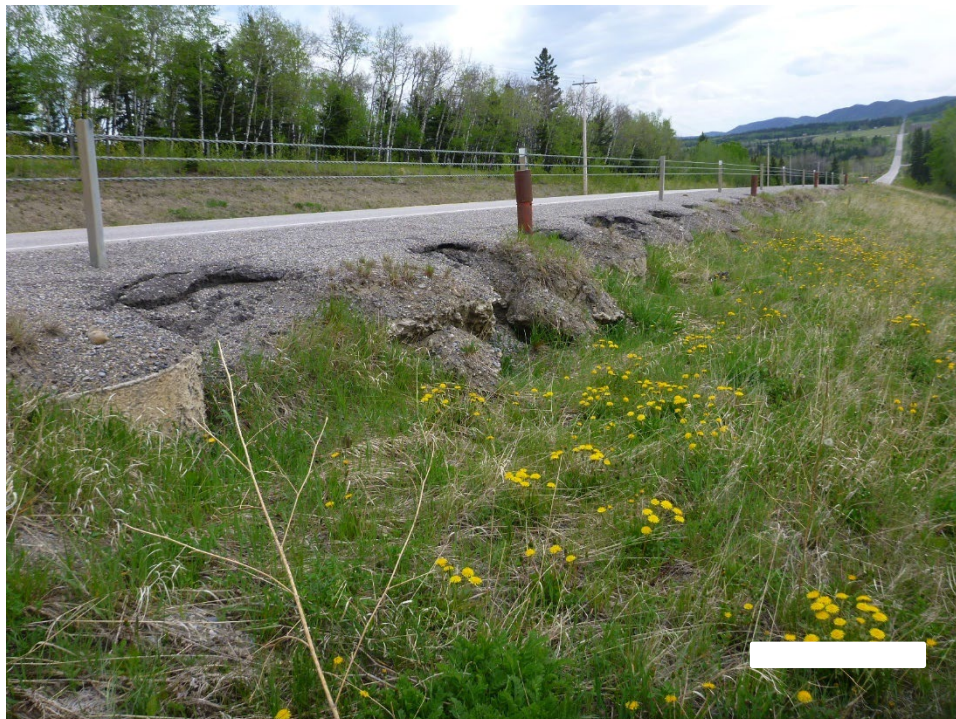
Photo 3 Settlement of the highway embankment slope and void formation along the top of the concrete piles. Photo taken May 26, 2025, facing southeast.
