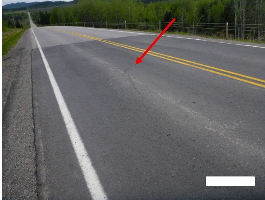
Photo 3 Settlement of the highway embankment slope and void formation along the top of the concrete piles. Photo taken May 26, 2025, facing southeast.
