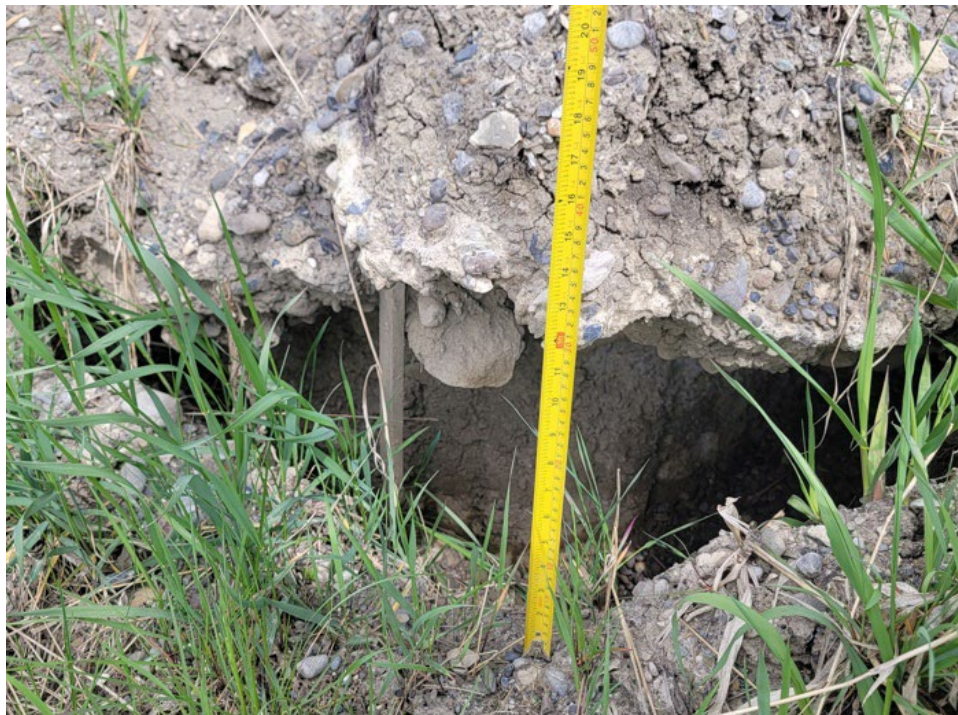
Photo 5 Settlement of the highway embankment slope and void formation along the top of the concrete piles. Photo taken May 26, 2025, facing east.
