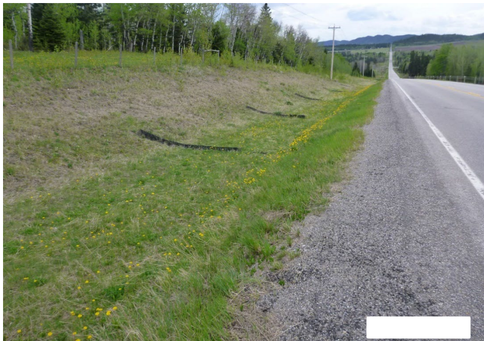
Photo 7 The east (northbound) ditch is well vegetated and is in good condition. Plastic ditch blocks previously installed at an unknown date. Photo taken May 26, 2025, facing south.
