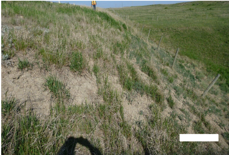
Photo 4 The north (westbound) highway embankment slope was relatively vegetated and appears to be performing well after the 2018 repair. Photo taken May 28, 2025, facing east.
