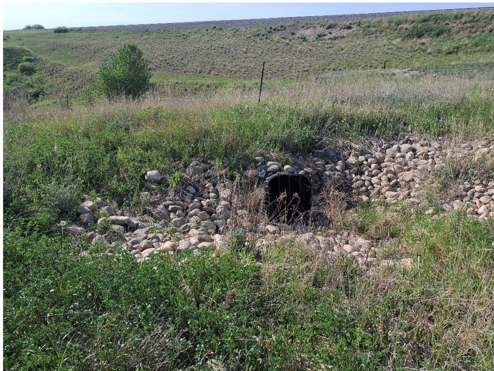
Photo 6 The HDPE culvert inlet appeared to be in good condition. Photo taken May 28, 2025, facing west.
