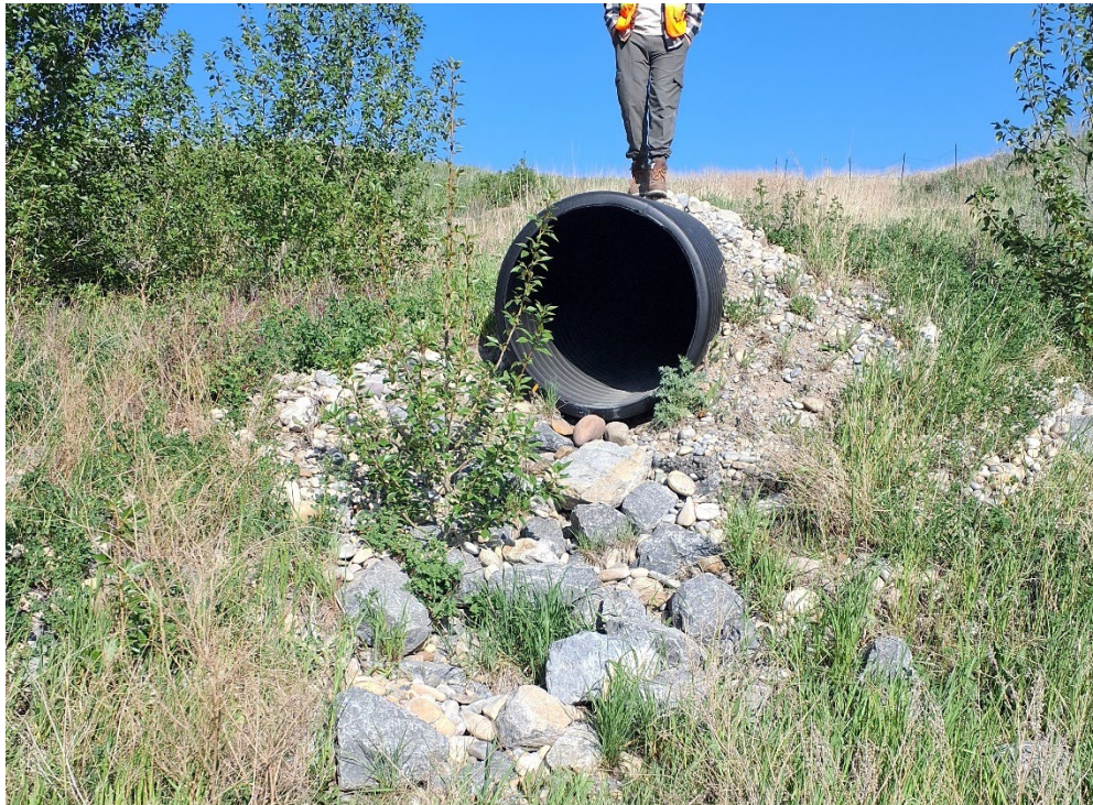
Photo 8 The ditch downstream of the HDPE culvert outlet was well vegetated and appeared to be performing well. Photo taken May 28, 2025, facing east.
