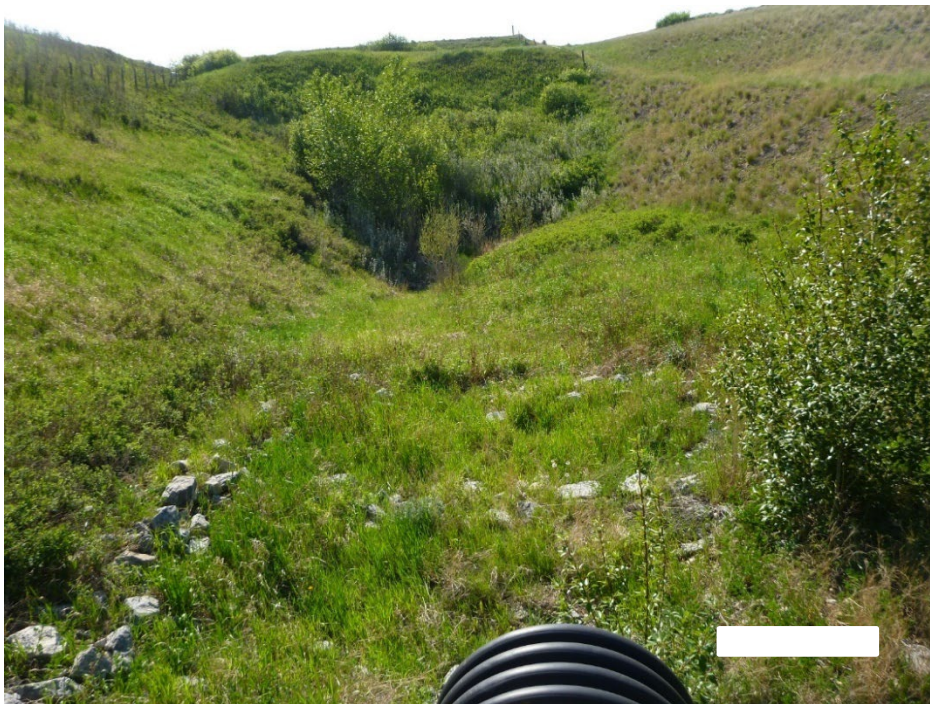
Photo 8 The ditch downstream of the HDPE culvert outlet was well vegetated and appeared to be performing well. Photo taken May 28, 2025, facing east.
