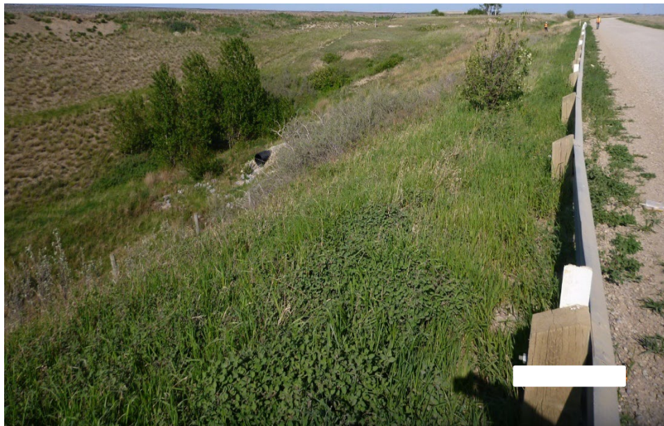
Photo 4 The north (westbound) highway embankment slope was relatively vegetated and appears to be performing well after the 2018 repair. Photo taken May 28, 2025, facing east.
