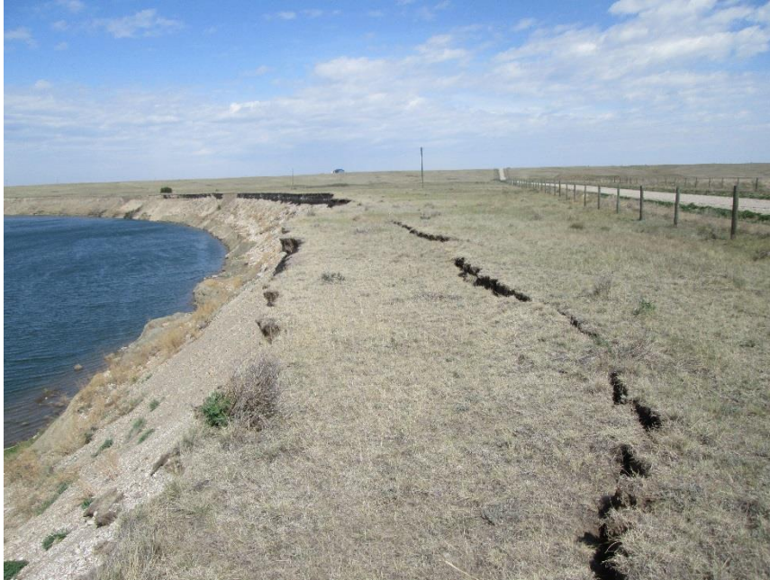
Photo 7 - (May 2016) – New cracks observed north of area of minimum offset. Facing north.
