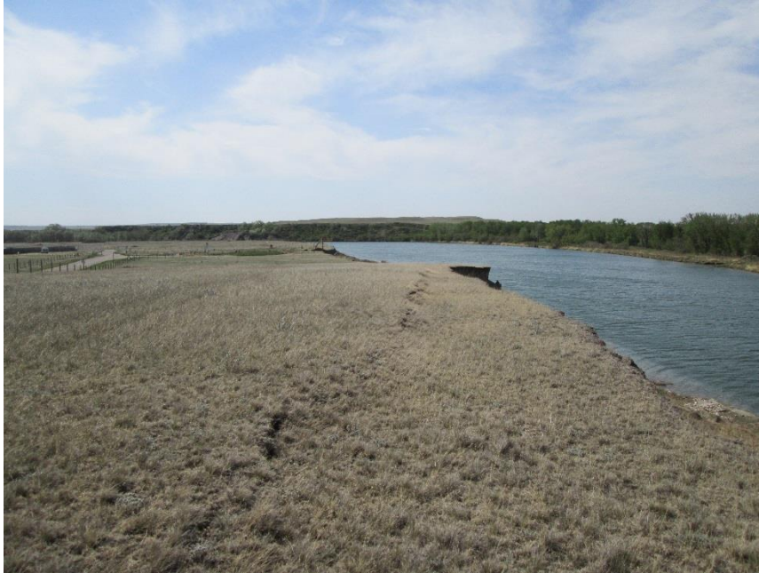
Photo 9 - (May 2016) – Cracks observed south of the main landslide location. Facing south towards ferry terminal.
