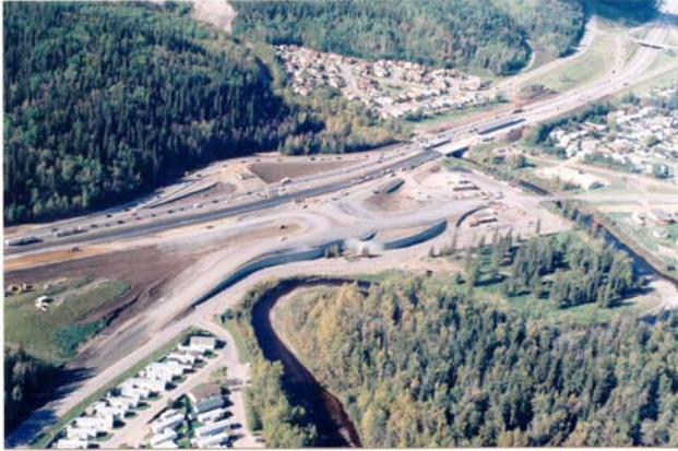
Figure 8. Interchange under construction (Fall, 2002)
