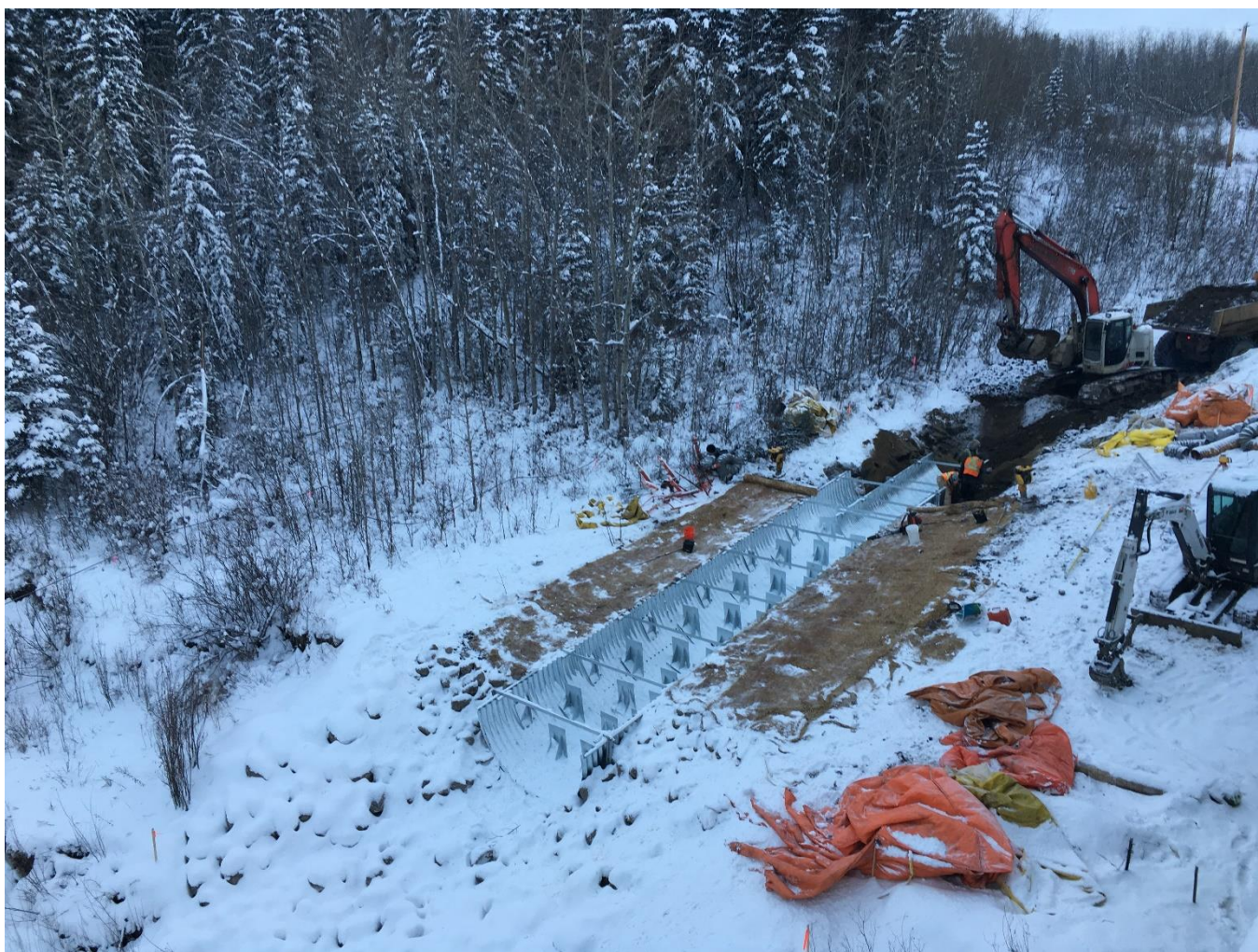
Site 2 – Installation of the 1.8 m dia. half culvert nested overtop the 3 m
