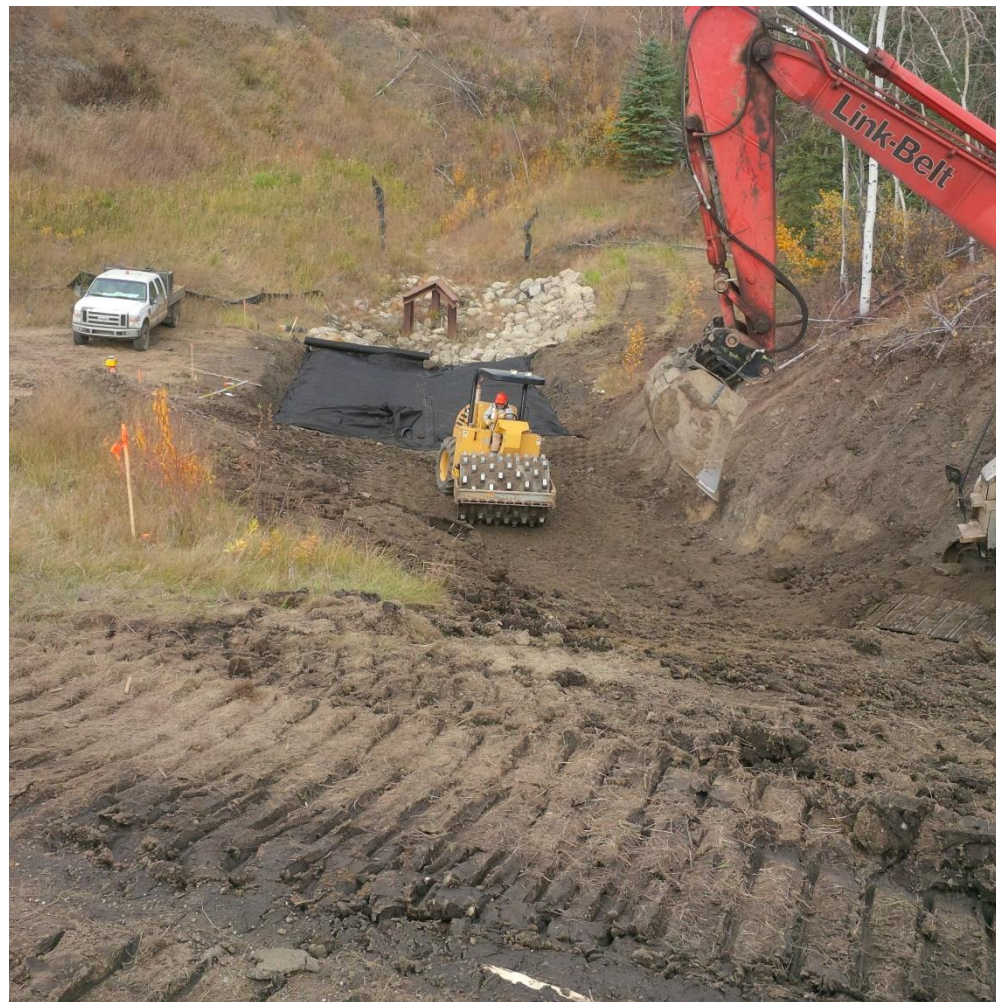
Site 3 – Excavation and Clay Backfill of ACB 60T Mat at Grimms Creek Culvert Entrance
