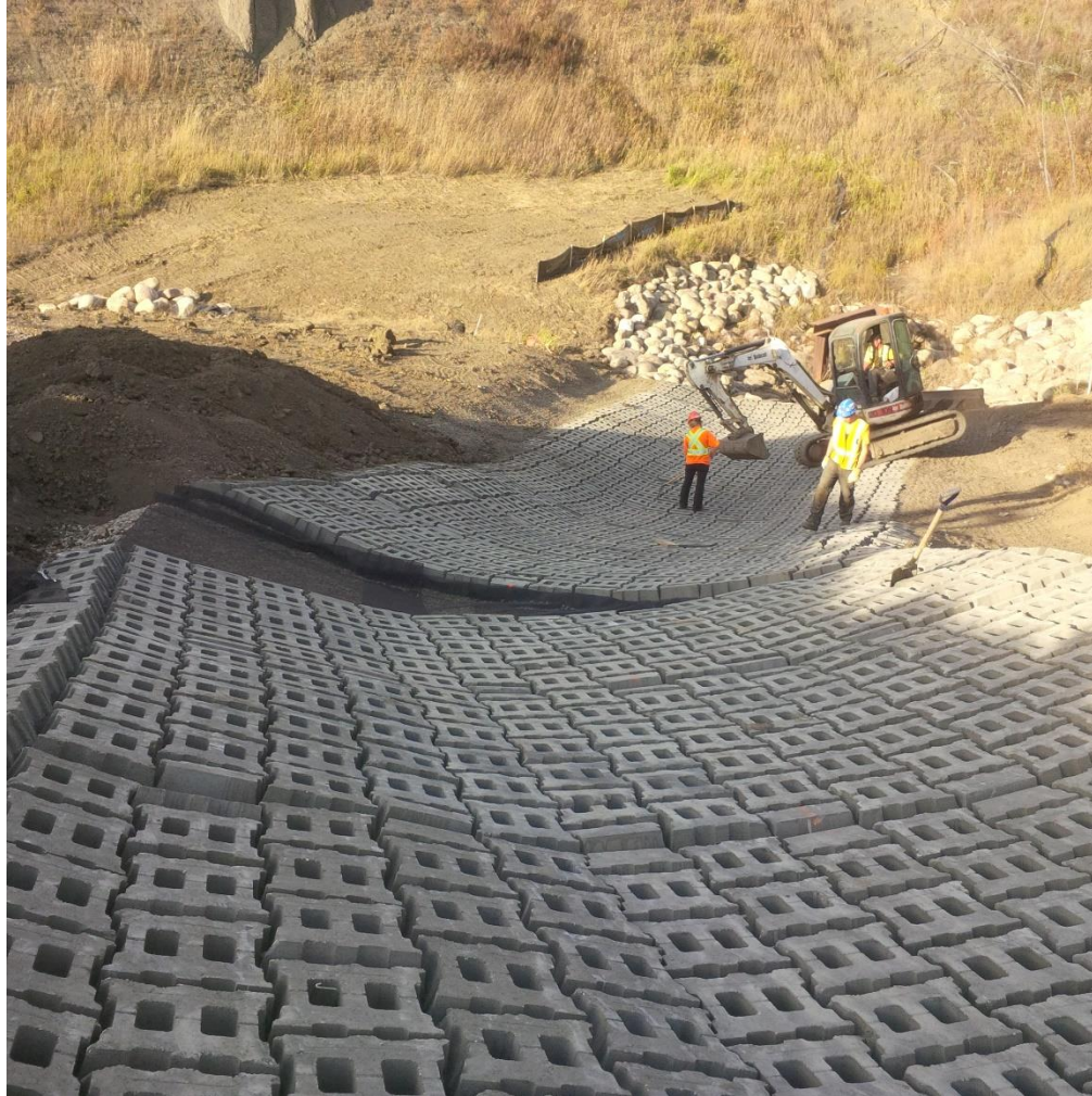
Site 3 – Almost Complete 60T ACB mat placement near entrance to Grimms Creek
