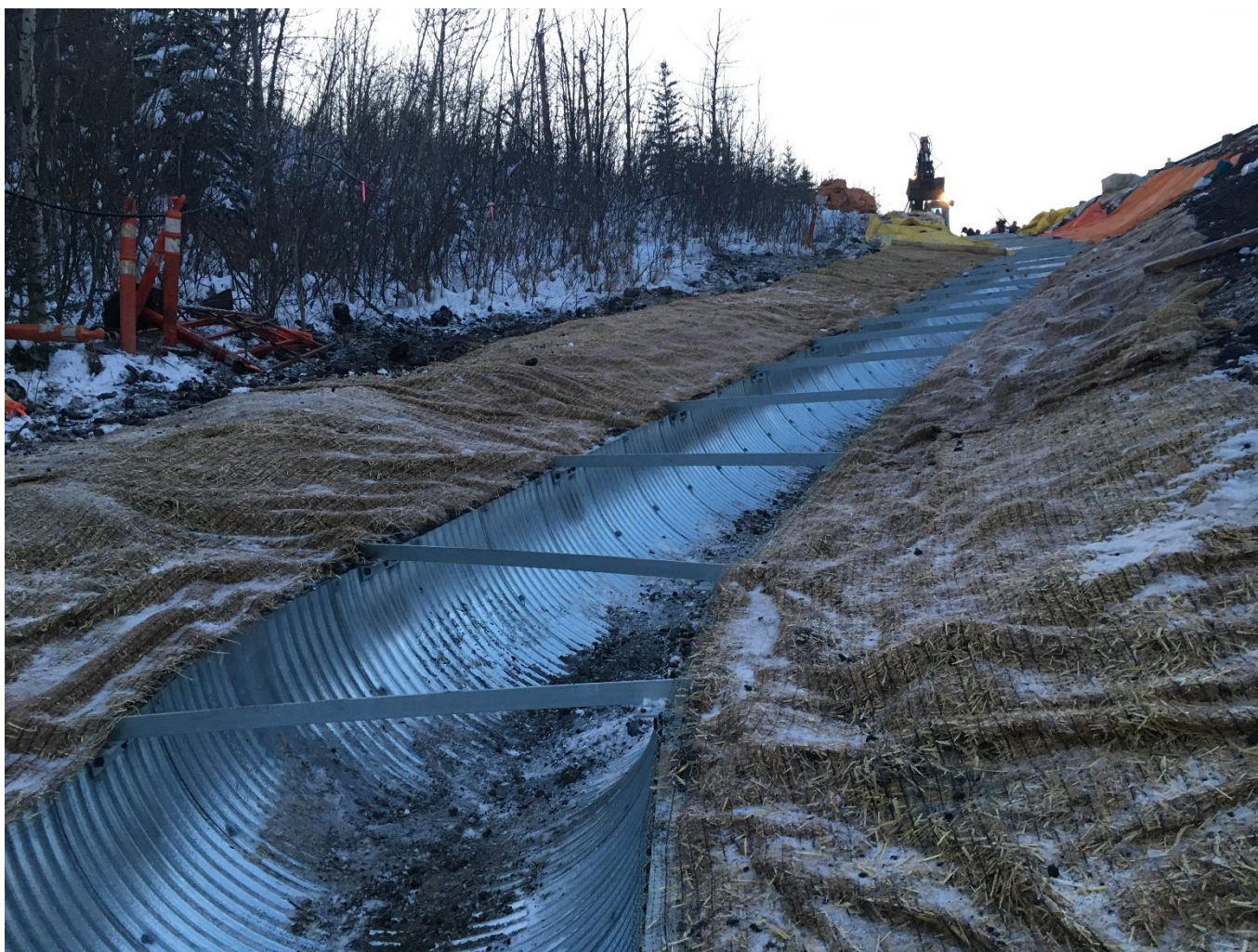
Site 2 – Near Completed 1.8 m dia. half culvert, Nov. 23, 2017
