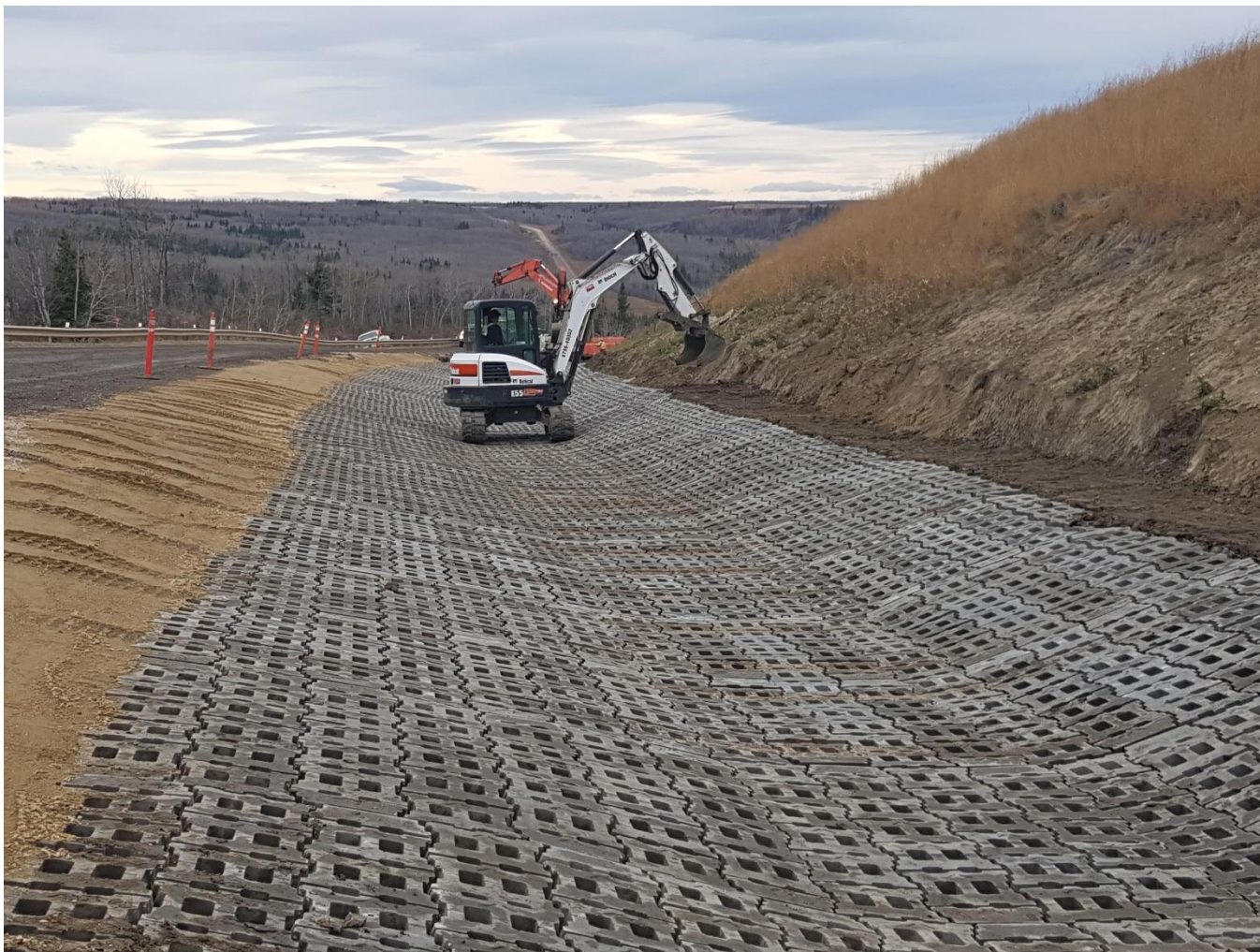
Site 3 – Compacted clay & Topsoil placement adjacent to ACB backslope mat edges
