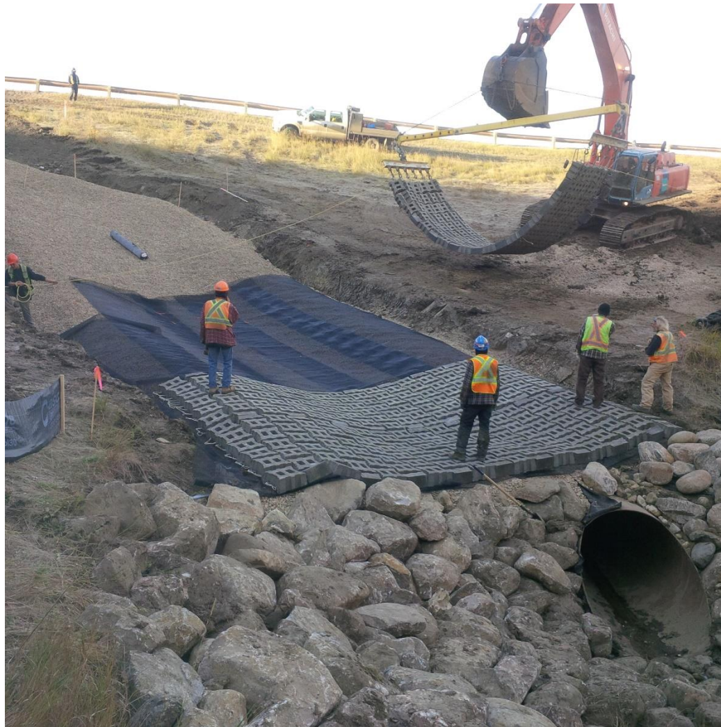
Site 3 – Microgrid and 60T ACB mat placement
