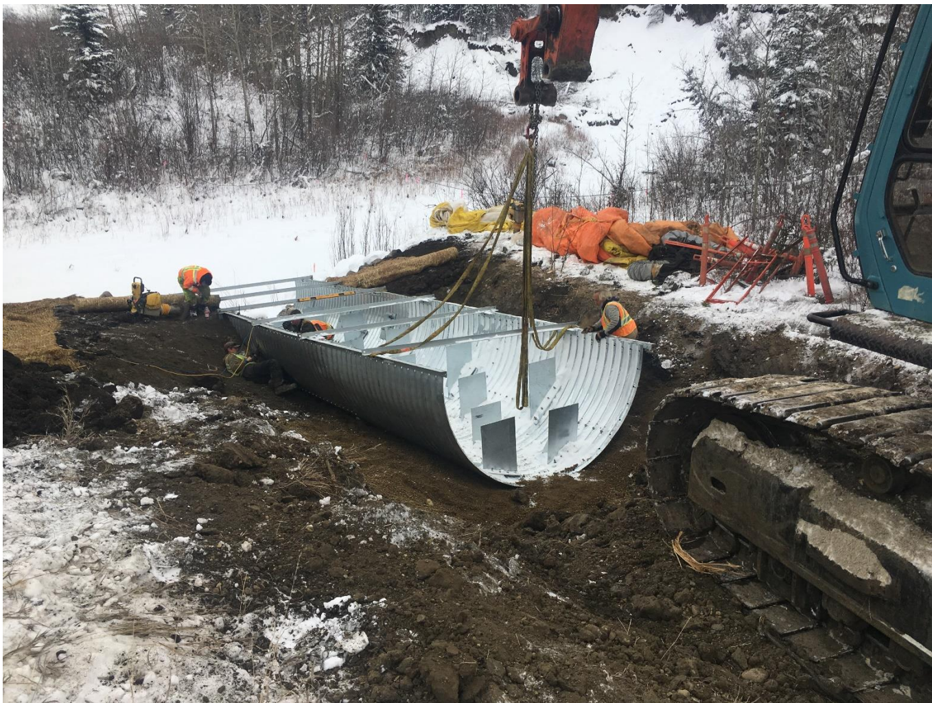
Site 2 – Placing the downstream section of the 3 m dia. baffled half culvert
