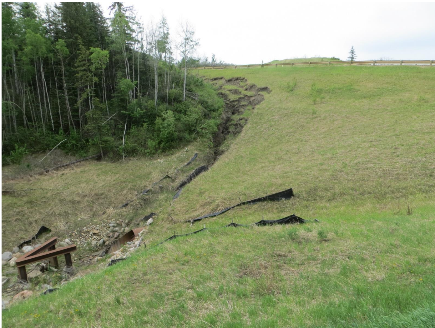
Site 3 Erosion (3 to 25% Ditch Grades)
