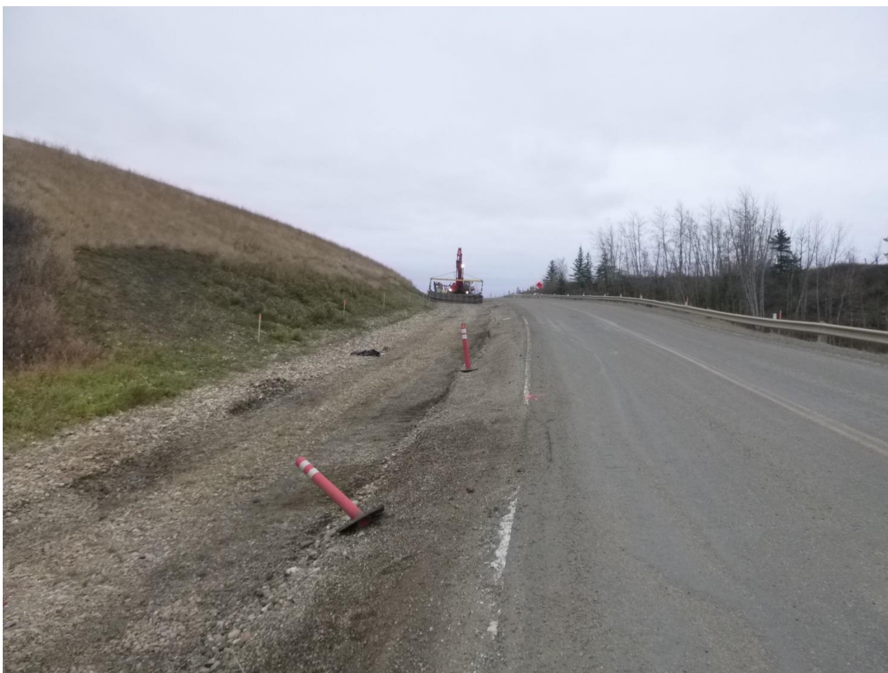
Site 3 – Erosion Void Backfilled with Pitrun Gravel in Fall, 2016 – PreConstruction Condition.
