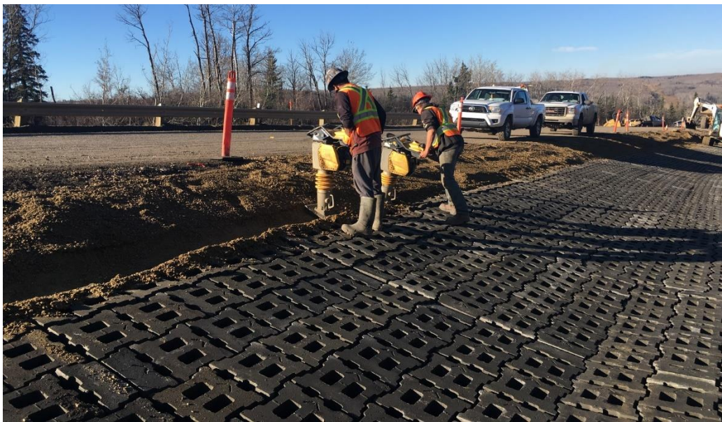
Site 3 – Compacting 2-25 gravel adjacent to ACB mat edges
