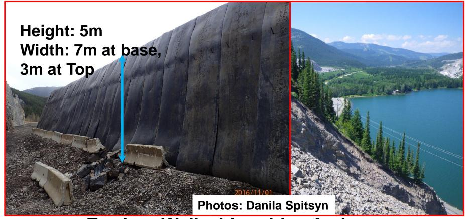
Earthen Wall with gabion facings.
