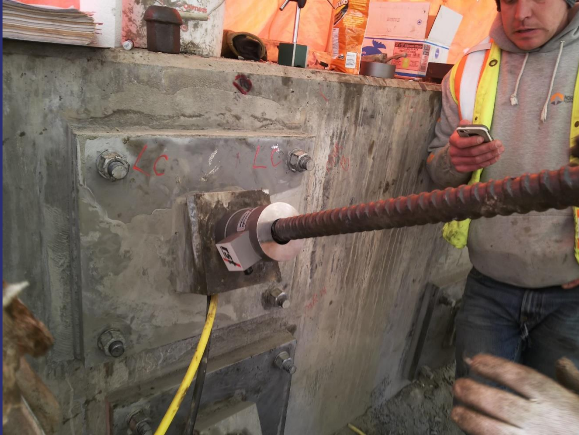
Waler Anchor fitted with VW Load Cell
