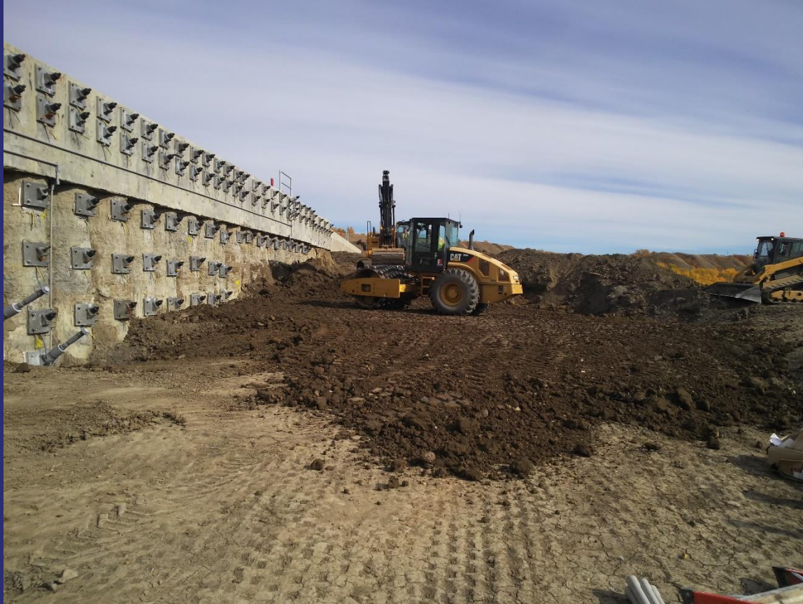
Wall Section 4 Backfill Lower Anchor Rows
