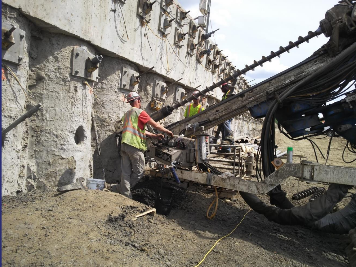
Wall Section 4 Anchor Auger Drilling
