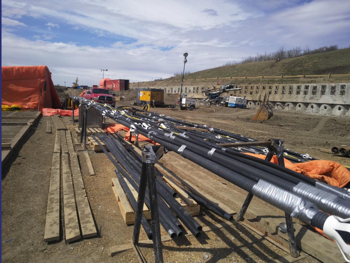
Assembled DCP Tieback anchors
