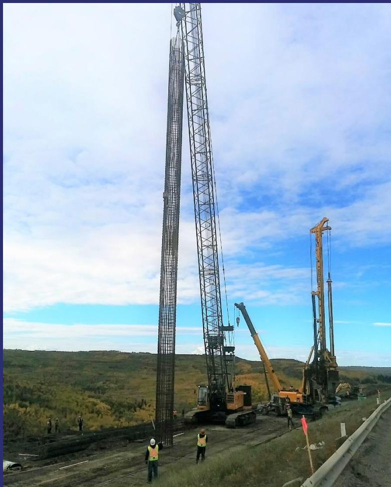
Single Lift Type 4 Steel Reinforcing Cage
