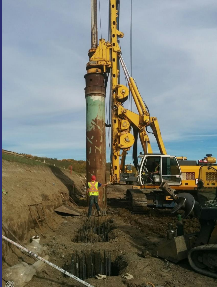
Bauer BG-24H Piling Rig Installing Casing
