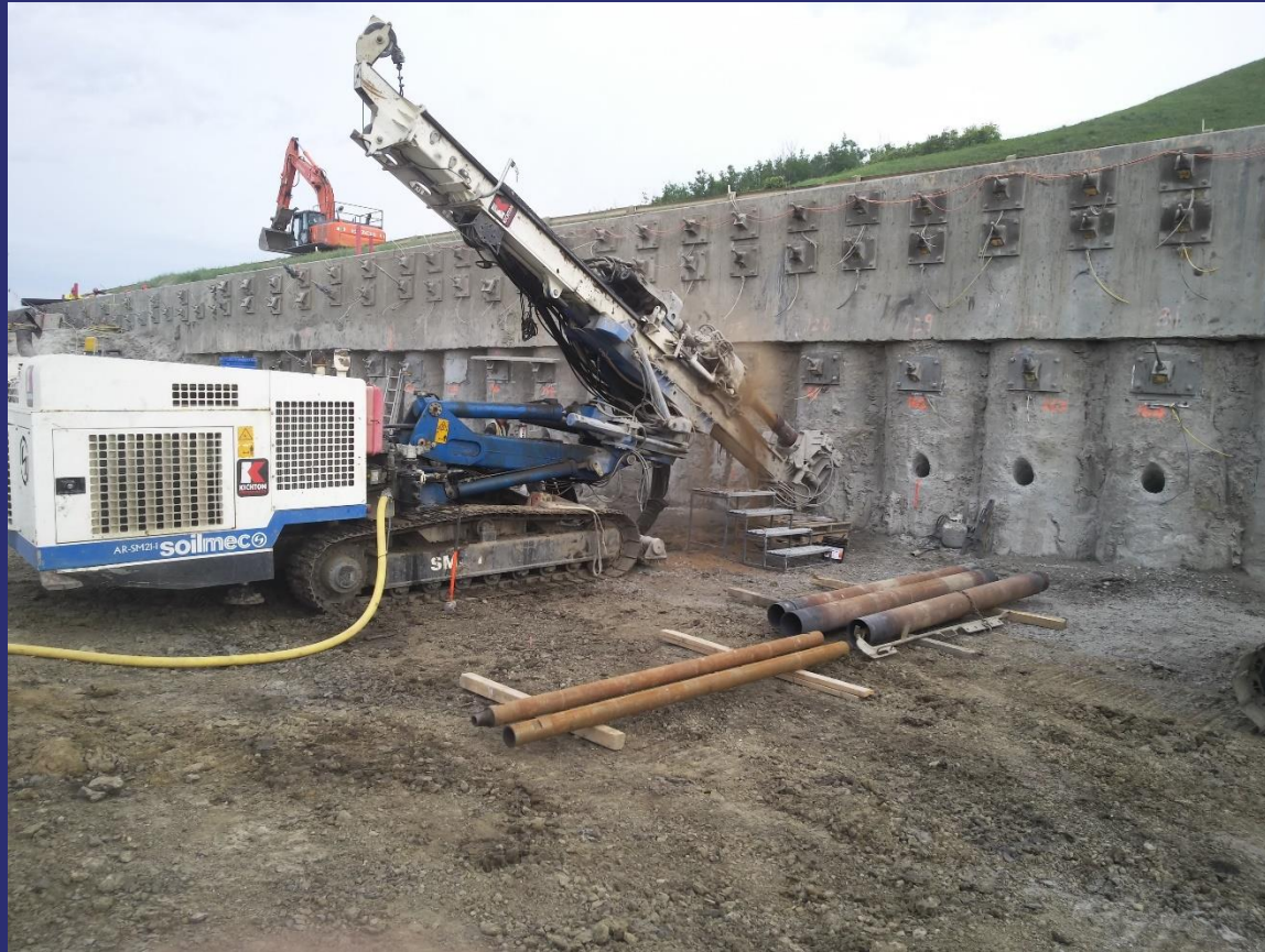
Wall Section 4 Anchor Air Rotary Rig
