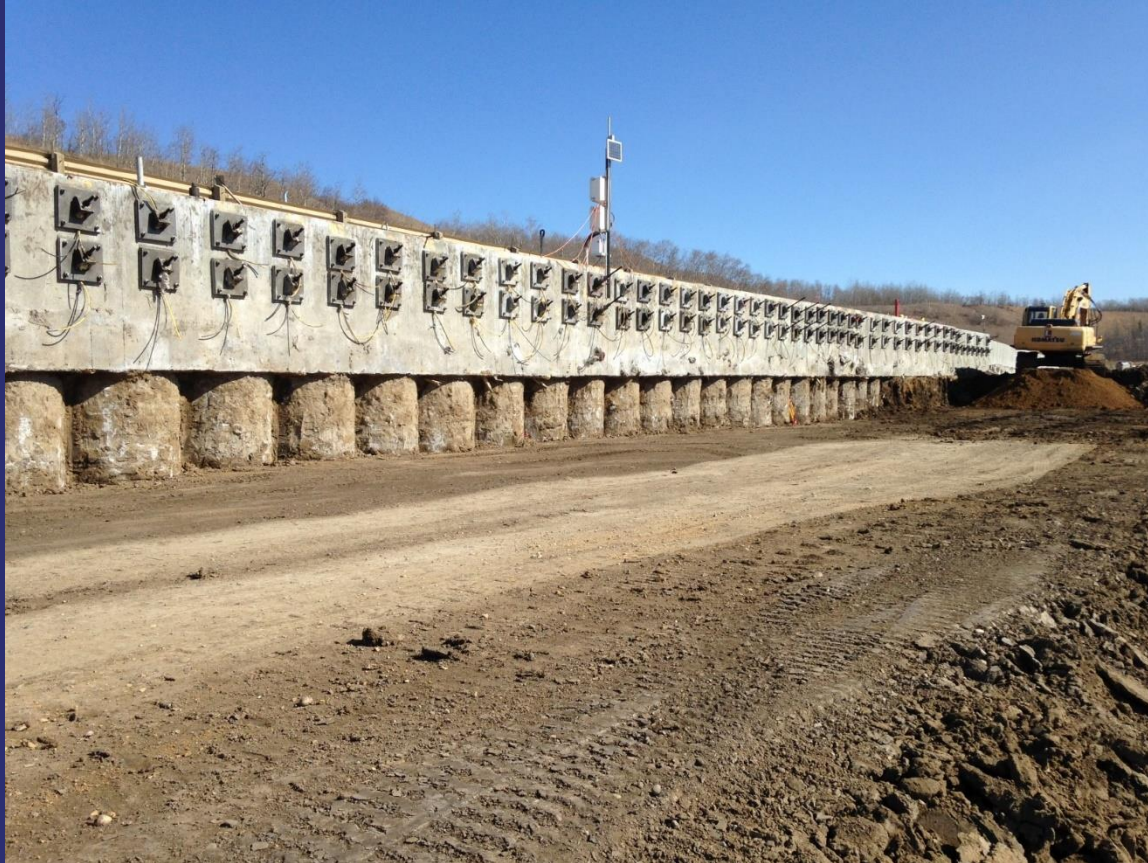
Waler Wall Section 4 Anchors Completed
