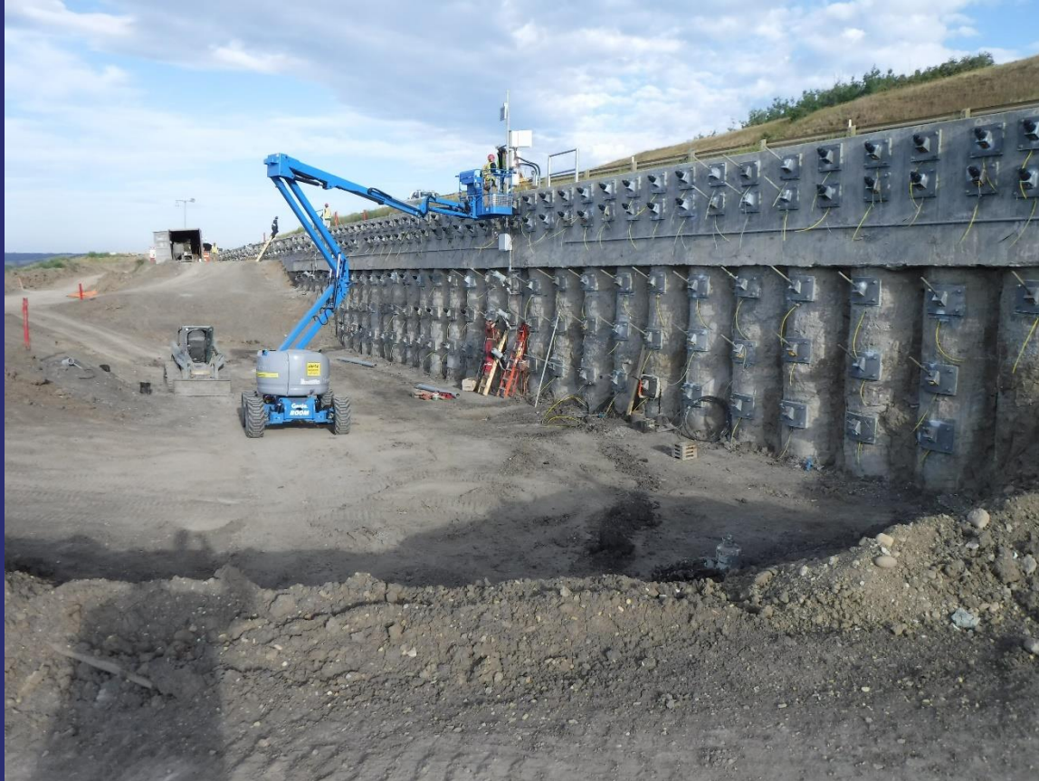
Wall Section 4 Anchors Completed
