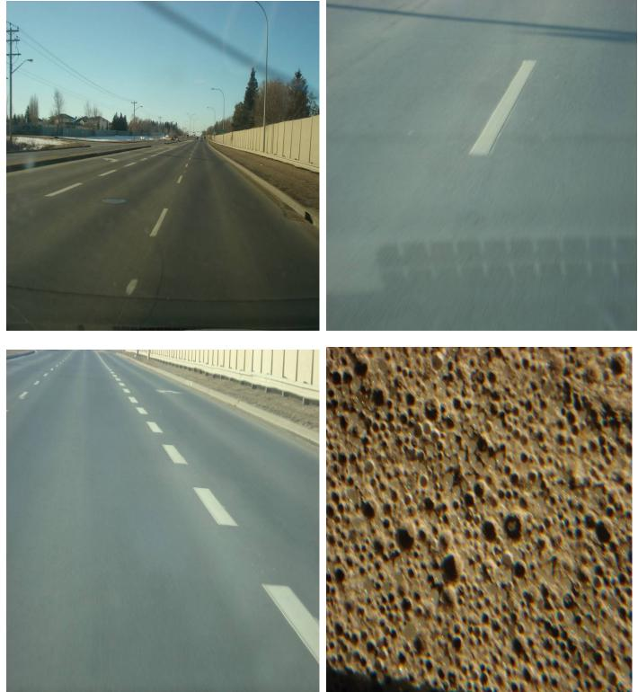
Durable markings at this location are in good shape, plenty of glass beads are present in the material, lines are dirty. This winter has not been harsh, need to access marking after one more winter.
