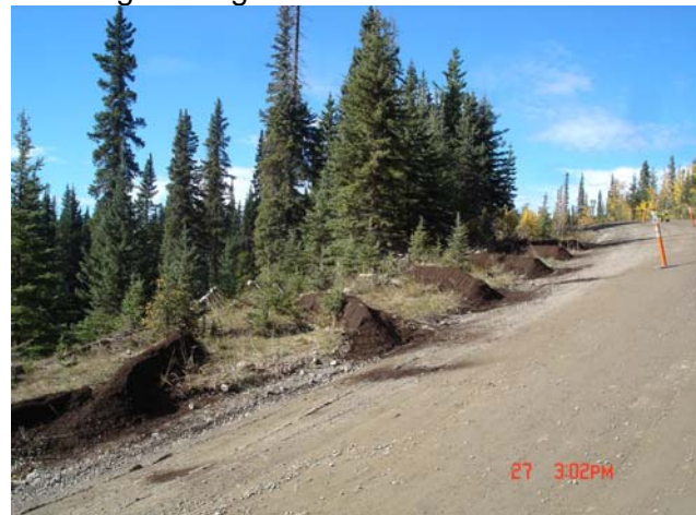
Compost berm alongside steep highway
