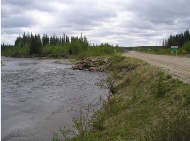
June 1, 2005 - Site 1 (before remediation work):
