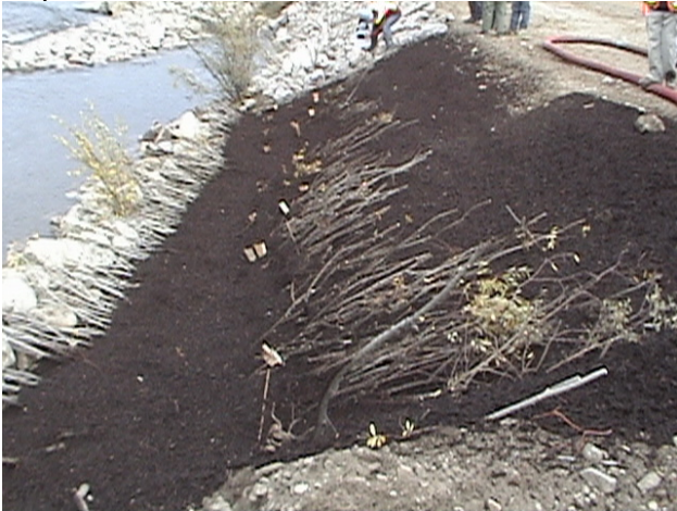
Compost application on slope
