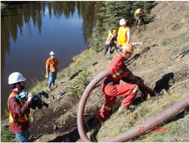
Compost applied on slope
