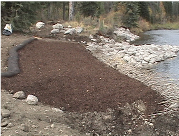
Compost blanket and Fitrex berm
