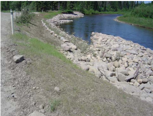
Compost blanket on slope and berm on road side
