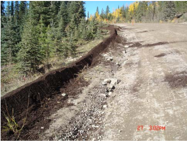
Compost berm along a ditch
