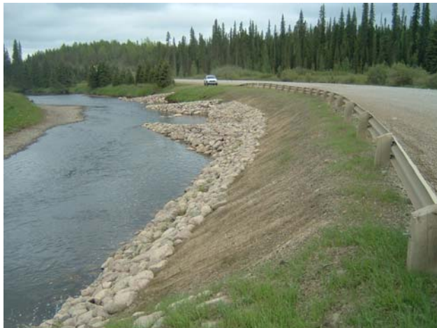
Grass catch along the guardrail
