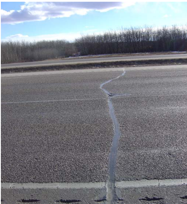
Sealant in good shape; small amount of sidewall adhesion problems.
