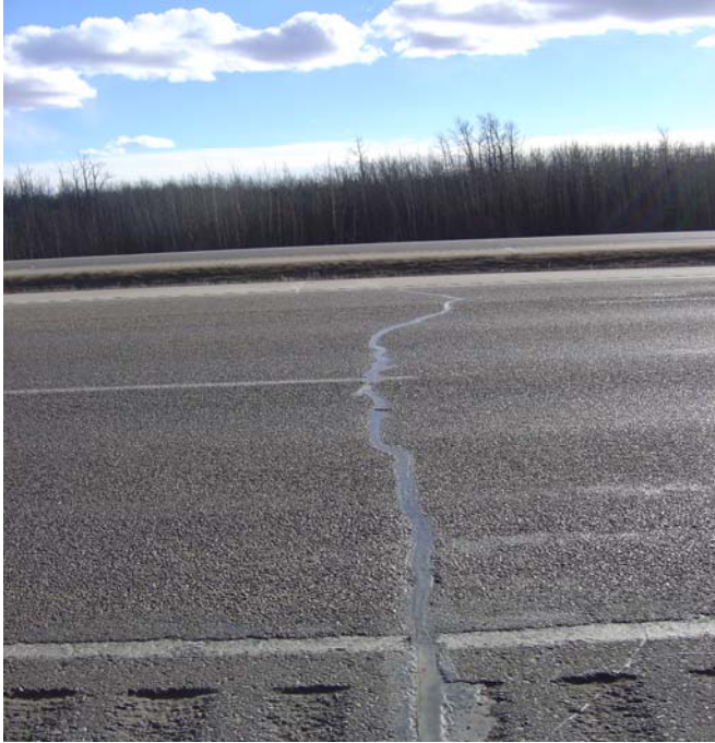
Transverse crack
