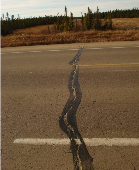
Transverse crack, treated with Deery #3723 sealant
