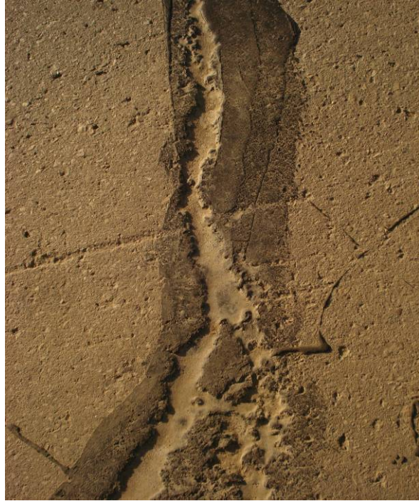
Transverse crack, treated with Deery #3723 sealant
