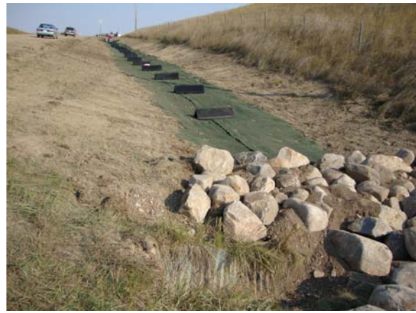
H894:04 – 2009 During construction
