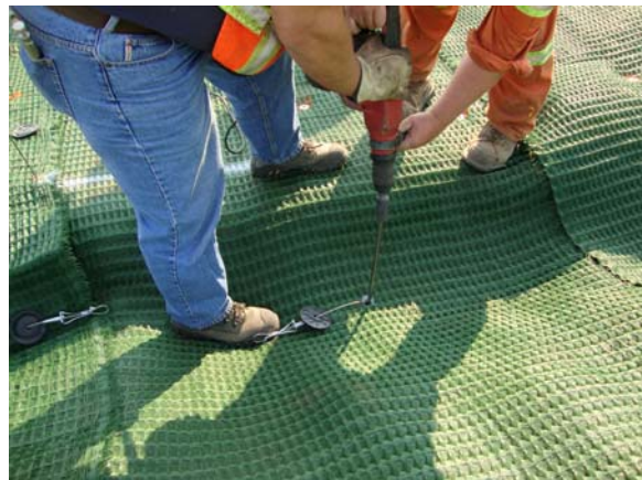
Hilti hammering the duckbill anchors
