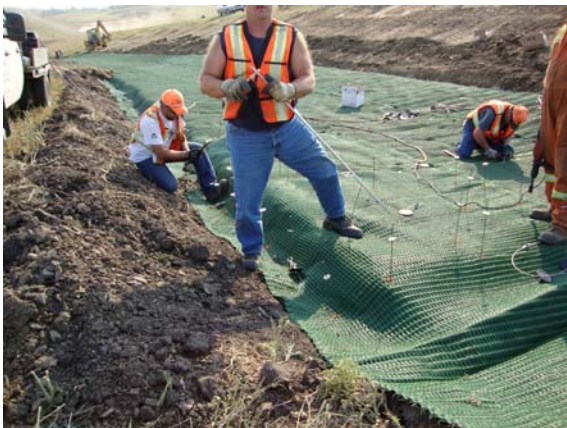
H614:02 - Placement of anchor pins
