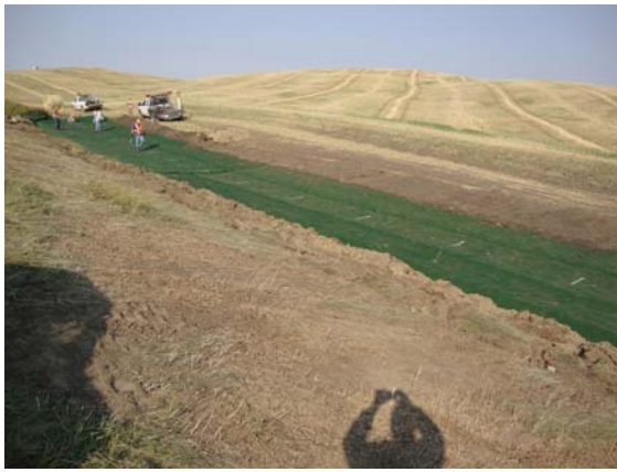
H614:02 – 2009 During construction
