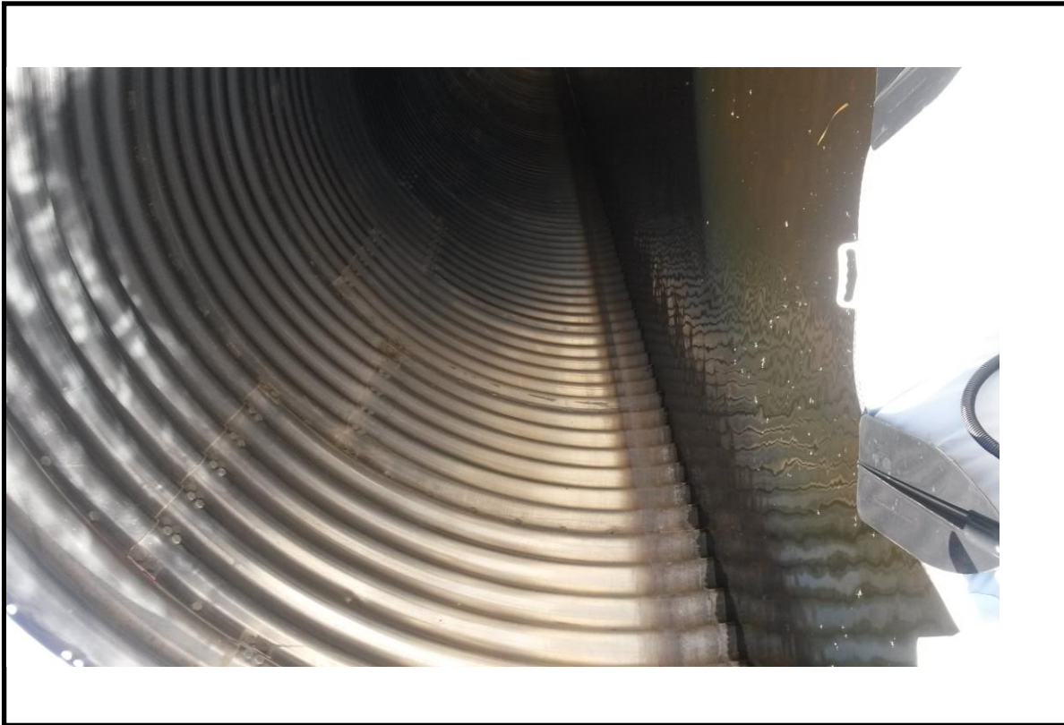
Looking u/s at the west wall of the pipe.
