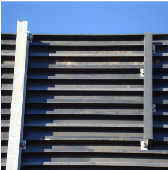
Close-up of sign panel connections, 12" and 24" panels
