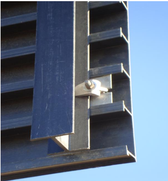
Close-up of sign panel connections, 12" and 24" panels
