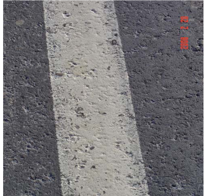
White skip line: good durability and bead retention. Retro readings: 119, 98, 94, 113, 100, 101, 105, 91, 101, 99 Average: 101 Mcd
