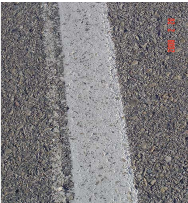
White edge line: good condition
