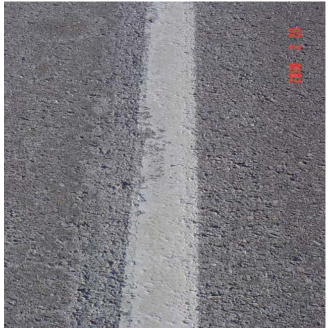
White skip line: some minor scraping, otherwise good condition Retro readings: 122, 110, 98, 86, 84, 118, 107, 108, 90, 107, 114, 98 Average: 104 Mcd
