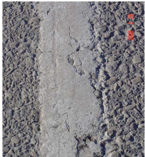
White skip line: good durability, poor bead retention Retro readings: 38, 50, 49, 54, 48, 47, 55, 50, 49, 41, 42, 42 Average: 47 Mcd
