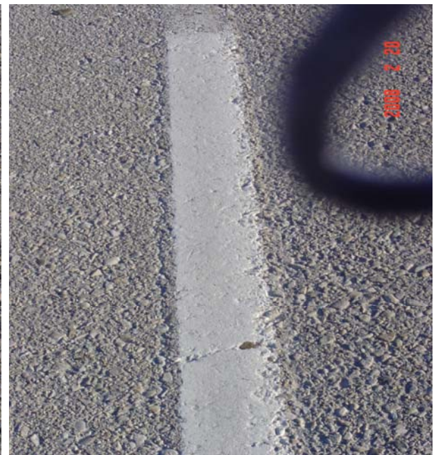
White skip line: very good condition.
