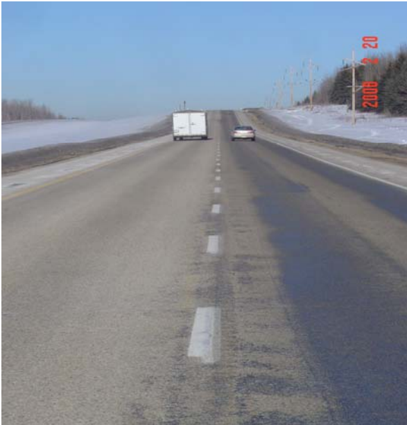
White Skip line: line is performing fairly well at this location. Retro readings: 76, 81, 81, 92, 92, 79, 88, 76, 104, 89, 86, 104
