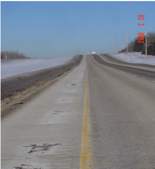
Yellow edge line: more snowplow scapping at this location, however good bead retention. Retro readings: 107, 124, 109, 103, 97, 93, 105, 122, 122, 93 –
