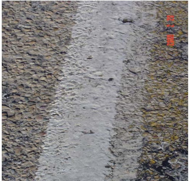
White Skip line: line is performing fairly well at this location. Retro readings: 76, 81, 81, 92, 92, 79, 88, 76, 104, 89, 86, 104
