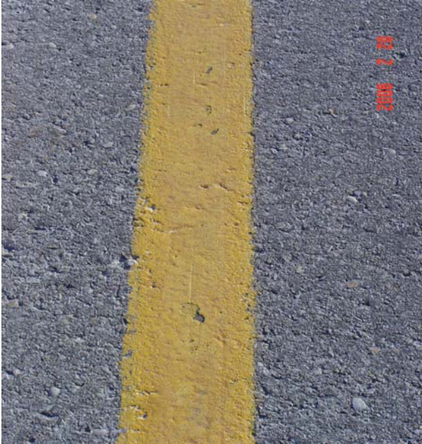
Yellow edge line: very good condition Retro readings: 75, 68, 70, 79, 66, 87, 91, 73, 82, 72, 76 Average: 77 Mcd
