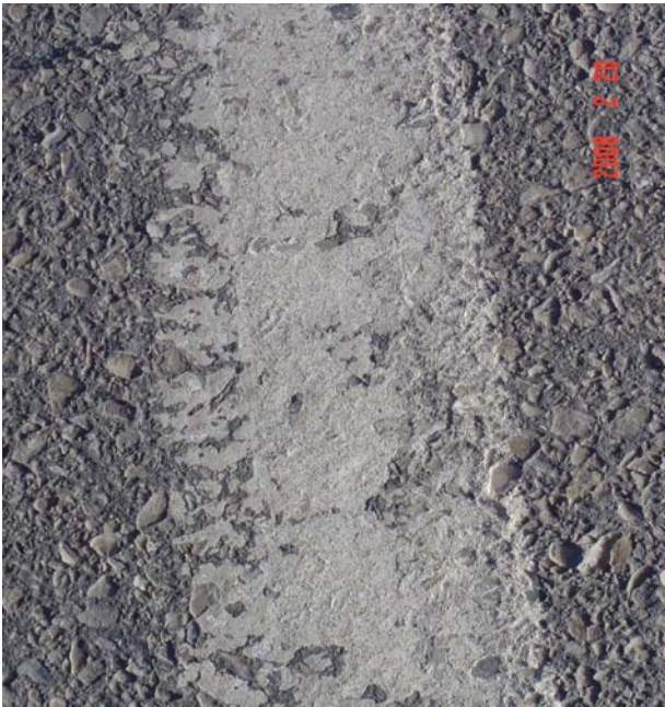
White edge line: fair durability, poor bead retention Retro readings: 33, 47, 42, 37, 39, 39, 42, 37, 38, 36, 38, 43 Average: 39 Mcd
