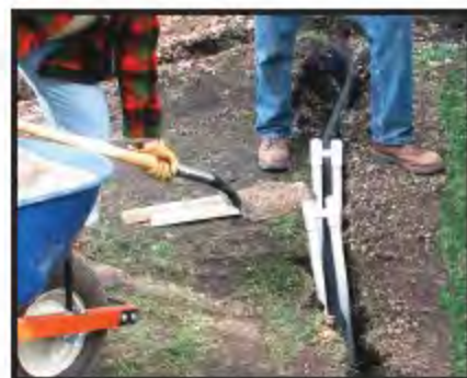
Hold Multi-Flow in the center of the trench while backfilling.
