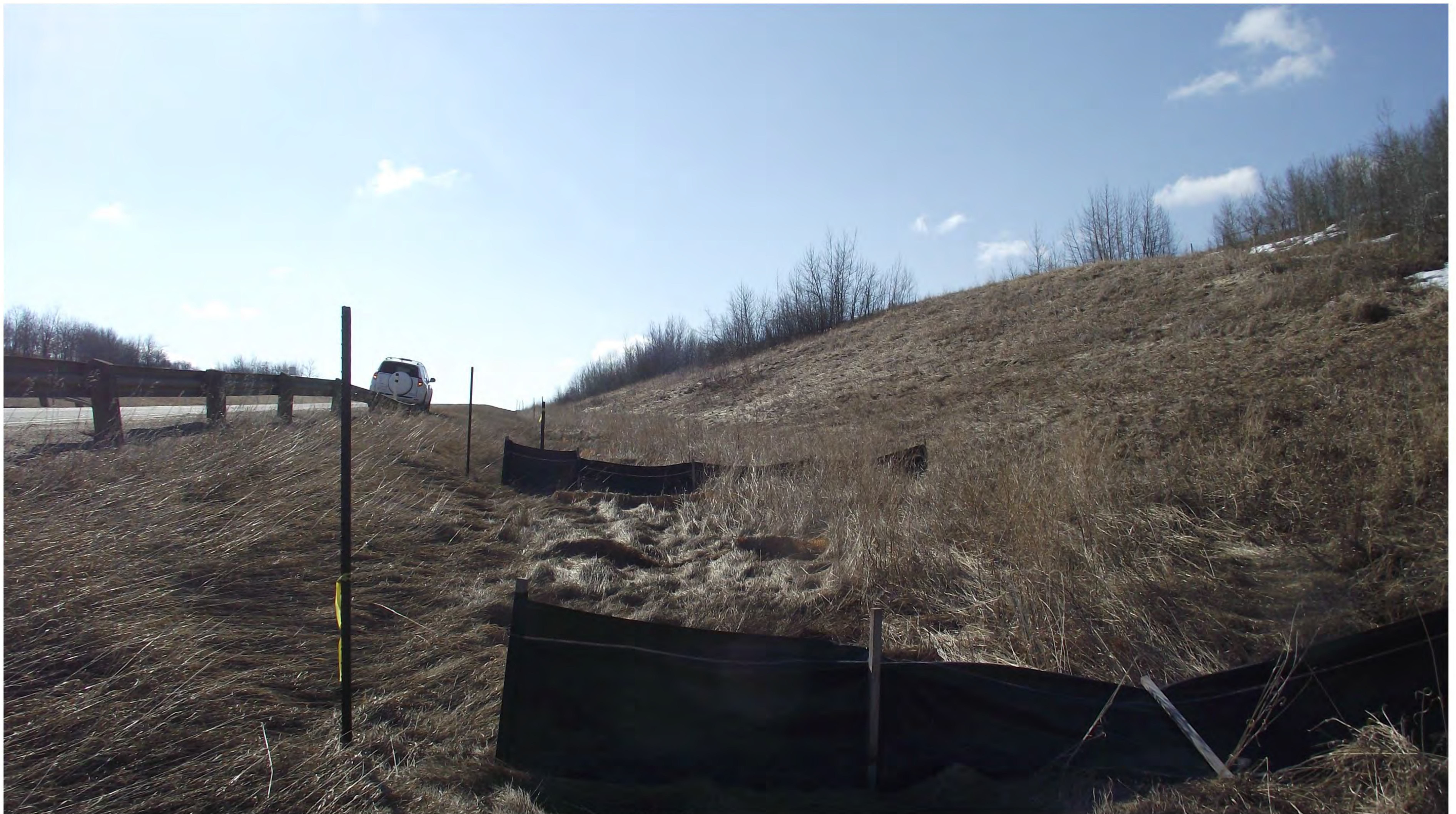
Hwy 14:16 km 48.6 Multiflow Dewatering Project, South Ditch showing growth 1 May 2013
