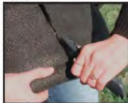
Cut Multi-Flow collector lines to the desired length using a utility knife.
