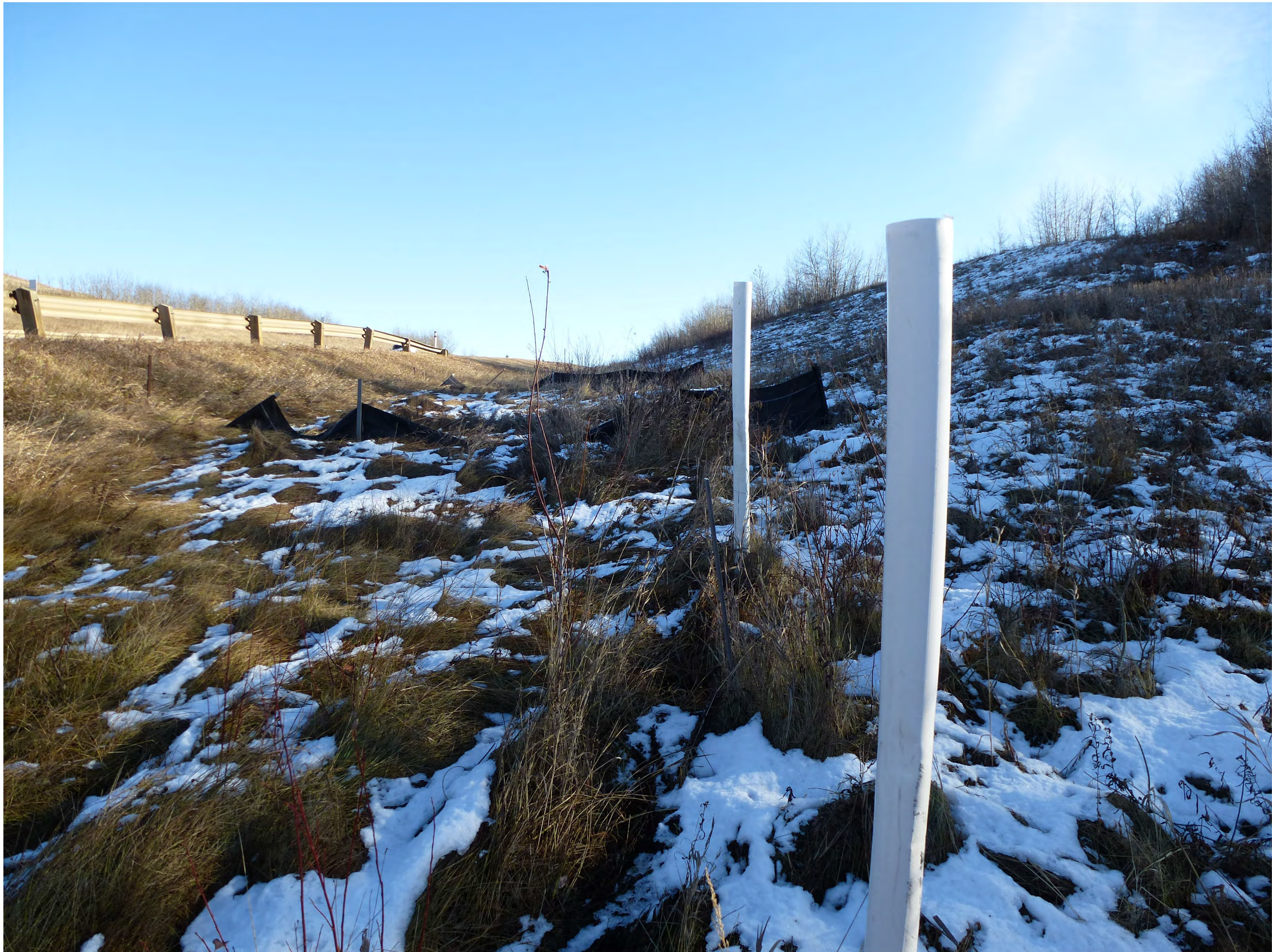
Hwy 14:16, km. 48.6, Multiflow installation inspection south ditch, 5 November, 2014
