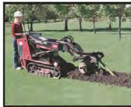
Begin trenching at the lowest point. Always check with utilities before digging.
