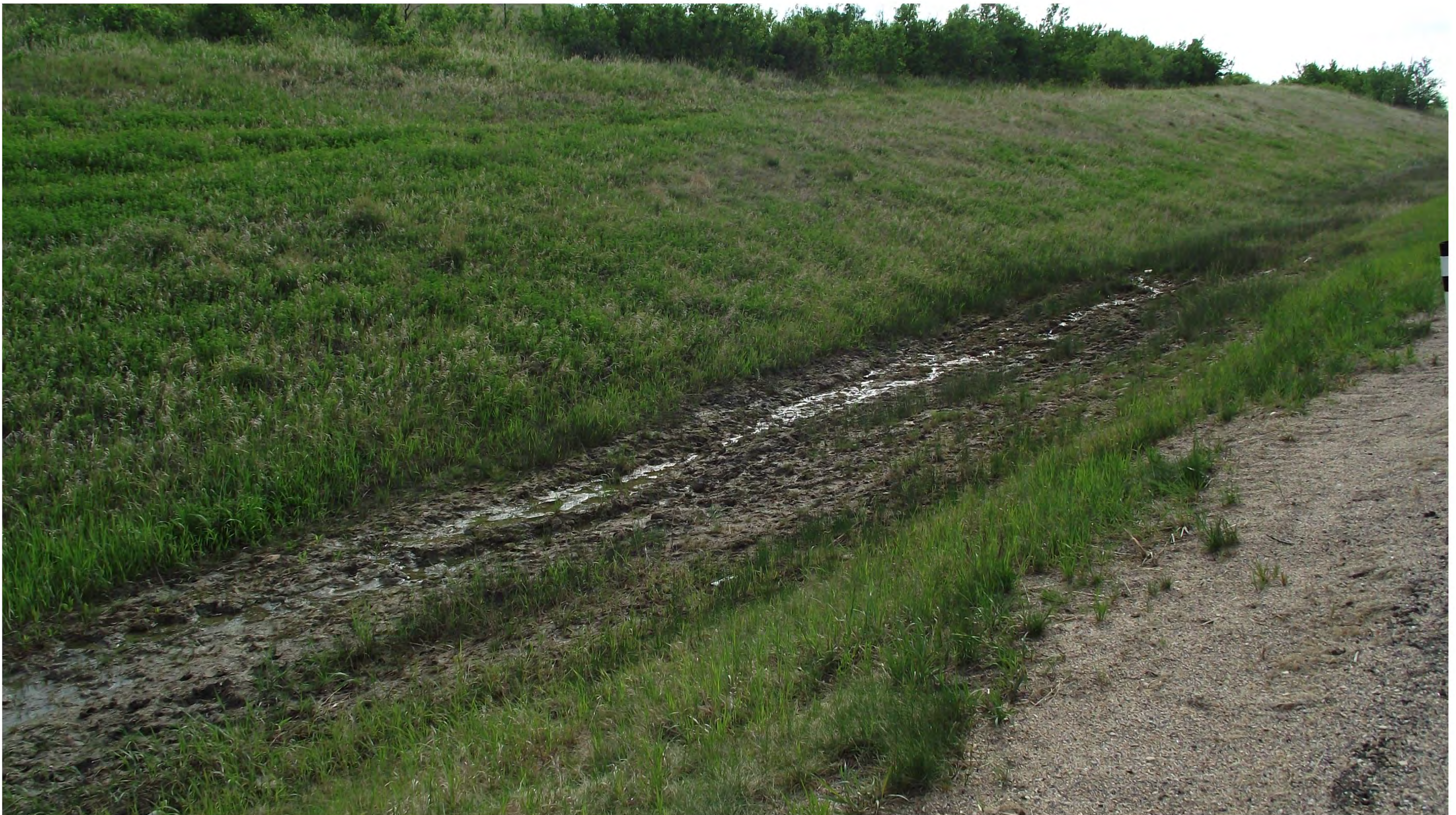
Hwy 14:16, km. 48.6, Multiflow pre-installation north ditch, 9 June, 2011
