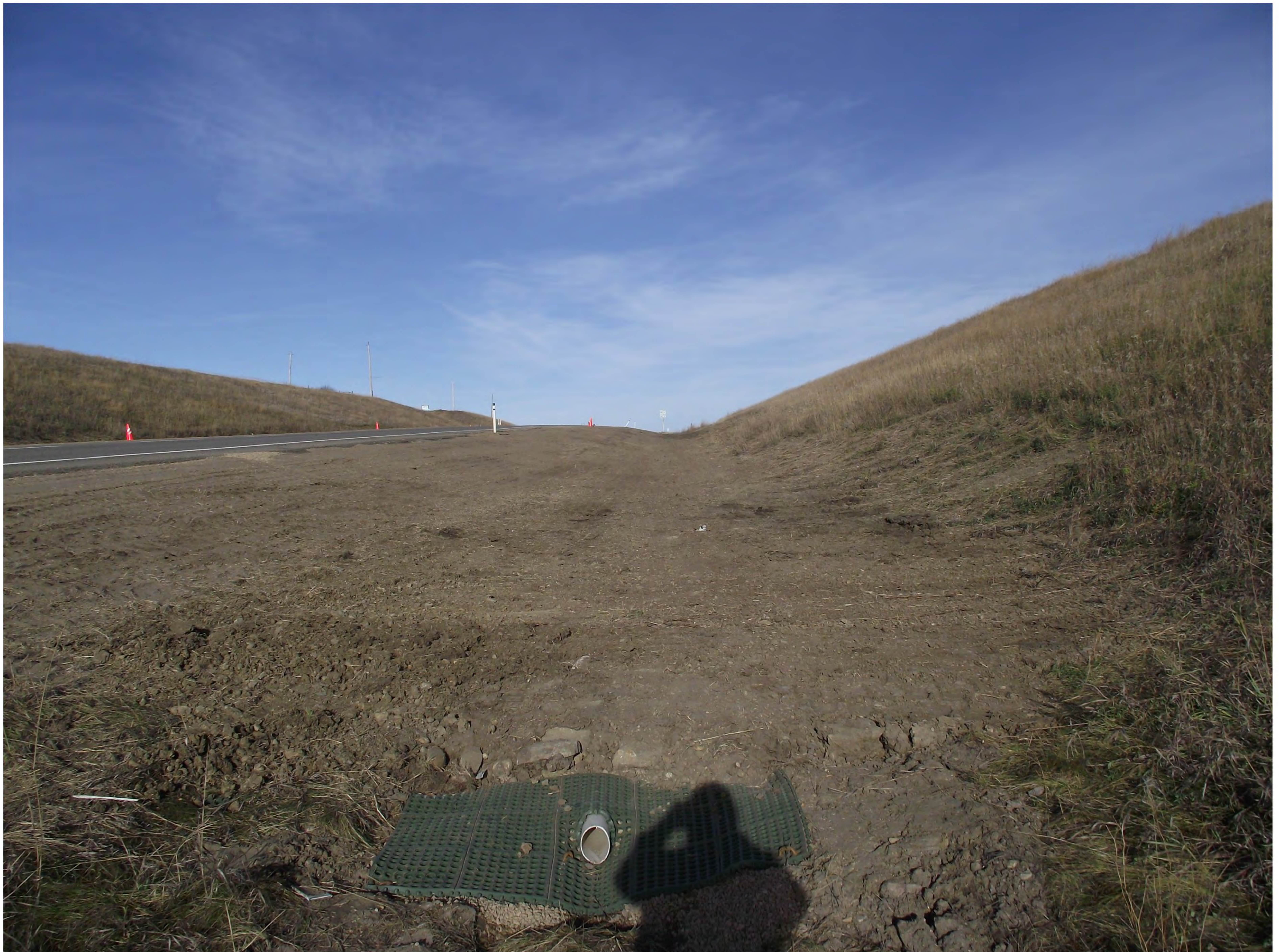
Hwy 41:18 at Hwy 883, Multiflow installed, 100mm outflow pipe on Shoremax, 13 October, 2010
