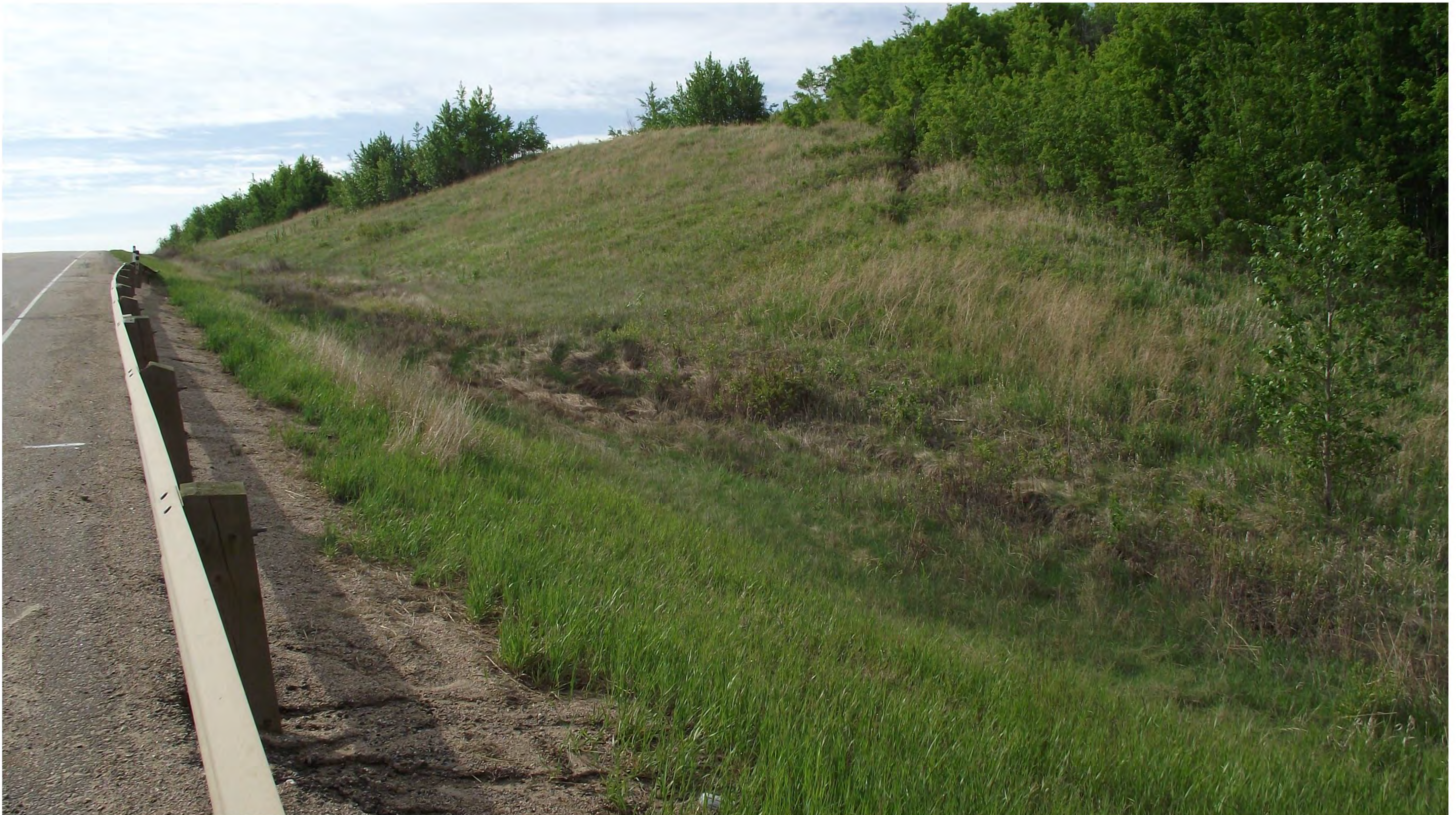
Hwy 14:16, km. 48.6, Multiflow pre-installation south ditch, 9 June, 2011
