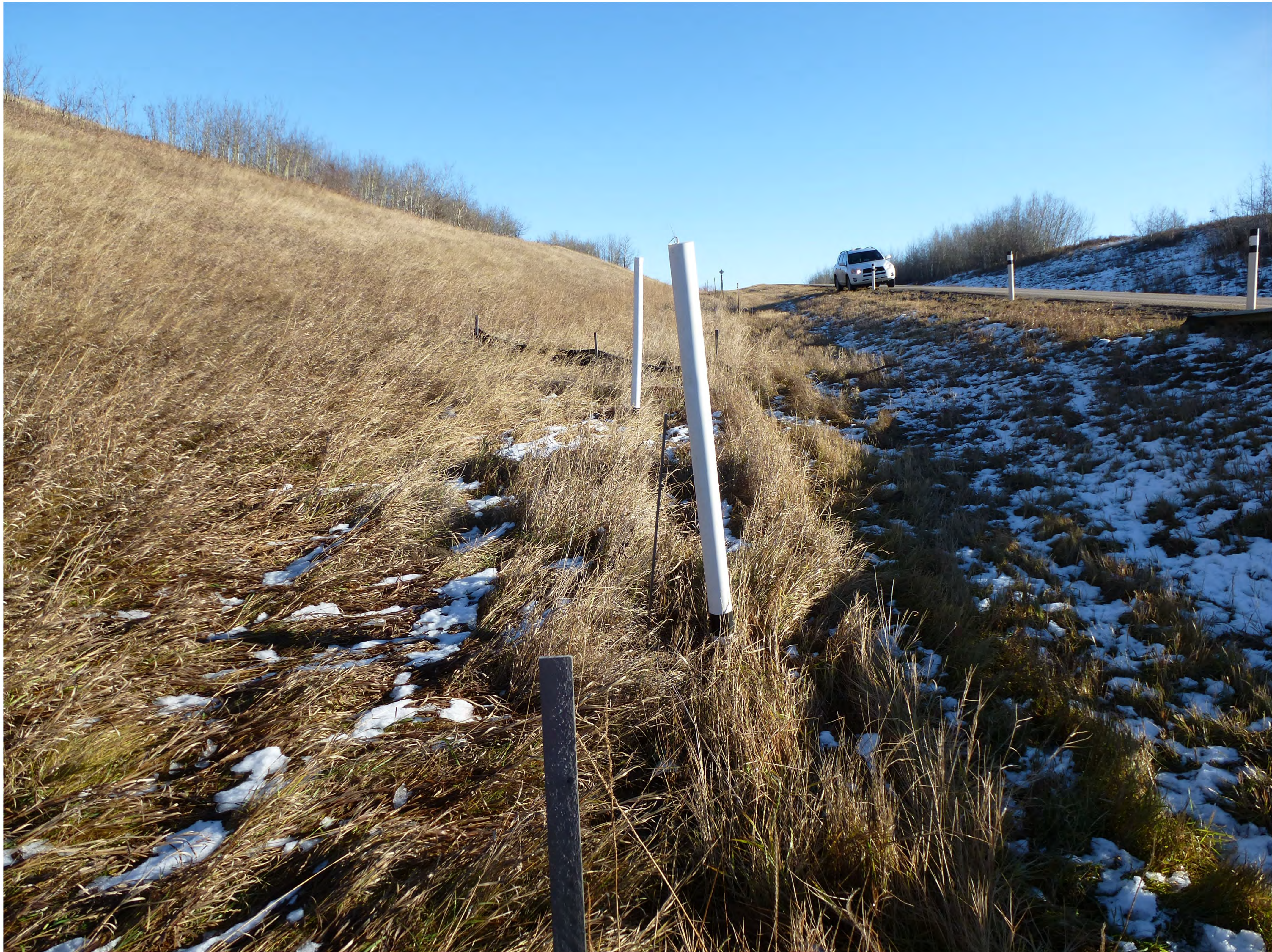
Hwy 14:16, km. 48.6, Multiflow installation inspection north ditch, 5 November, 2014
