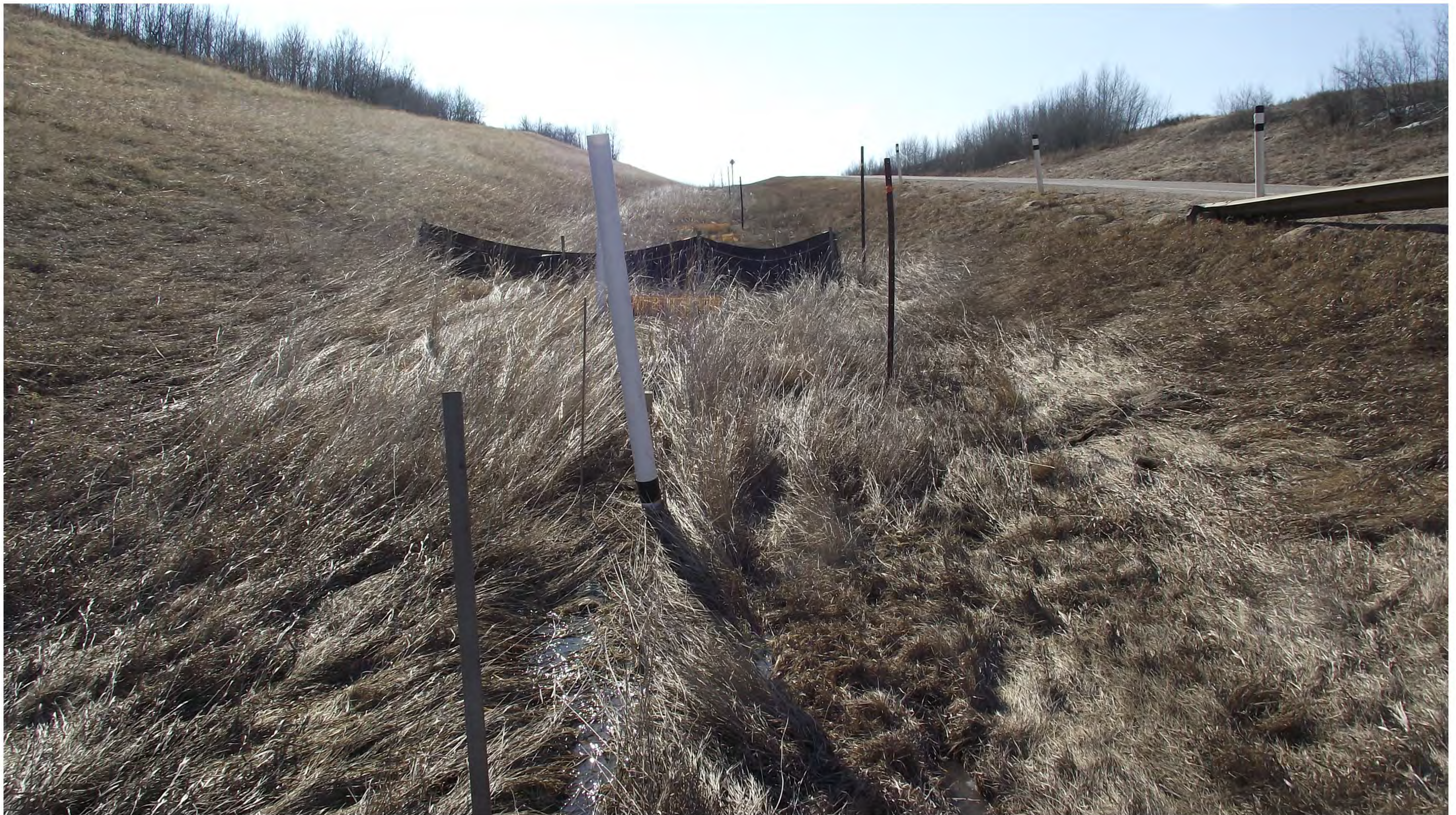
Hwy 14:16 km 48.6 Multiflow Dewatering Project, North Ditch showing growth 1 May 2013
