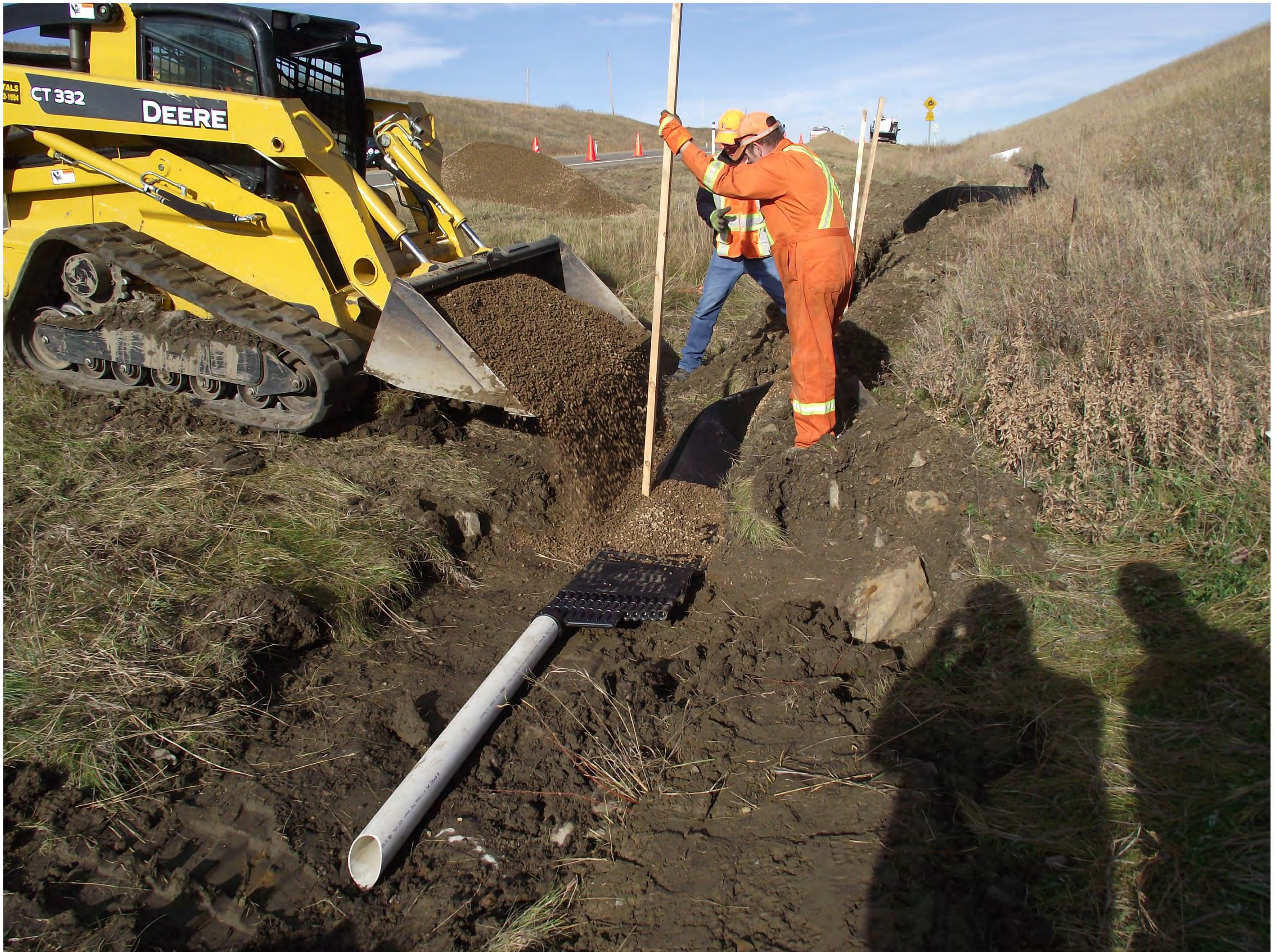
Hwy 41:18 at Hwy 883, Multiflow install and 100mm outflow pipe, 13 October, 2010
