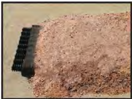
Cover with clean, very coarse sand before bringing in fill.
