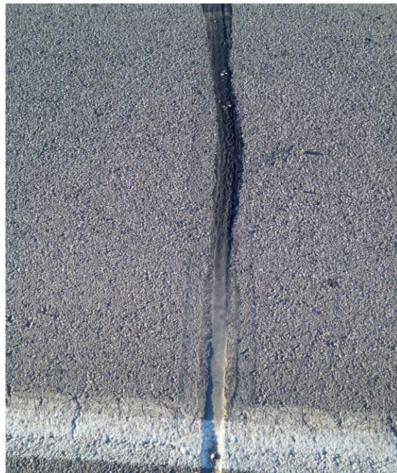
Sealant is performing very well in the transverse cracks, good cohesion and adhesion.
