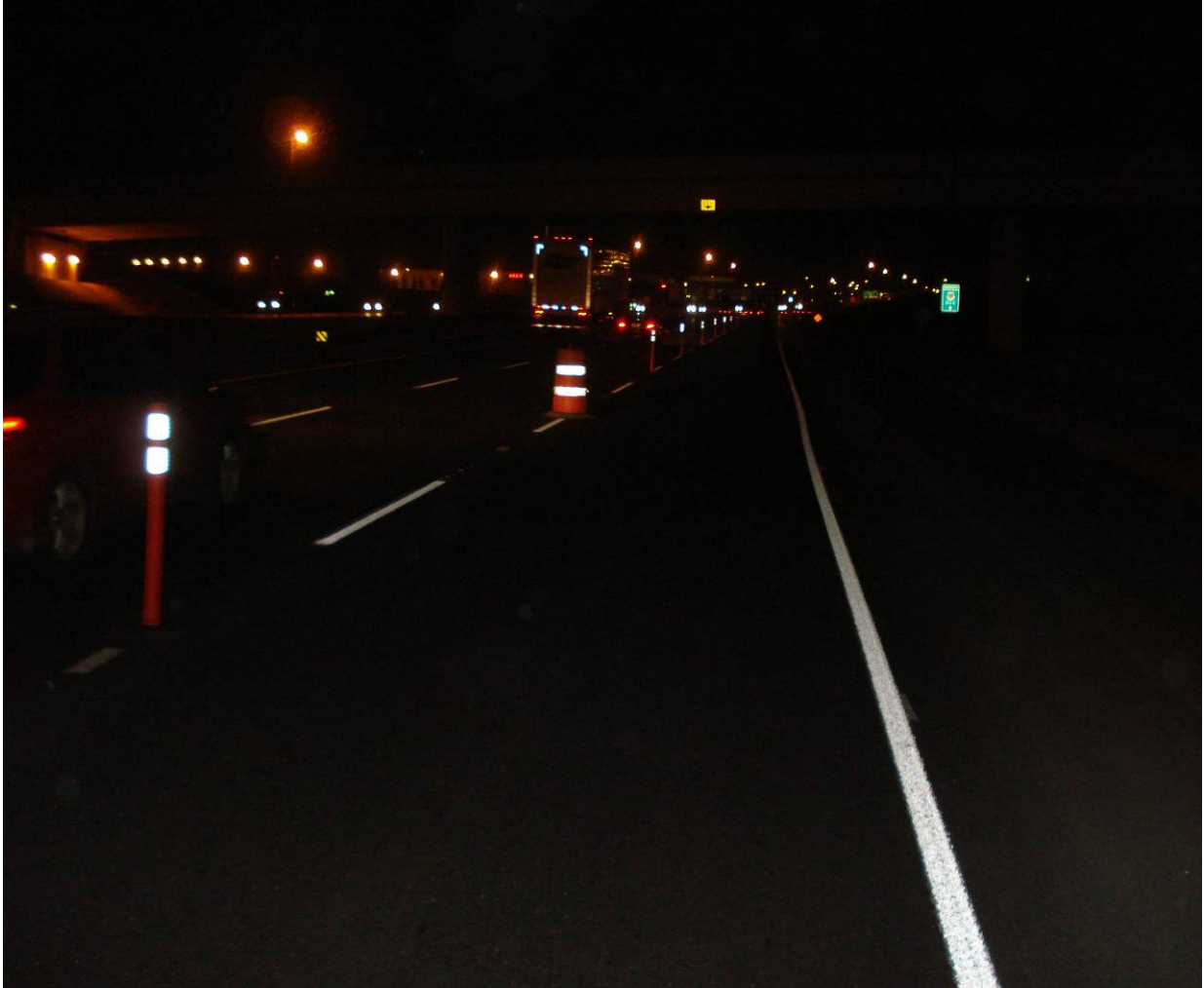
Pathfinder markings are very reflective, providing positive delineation
