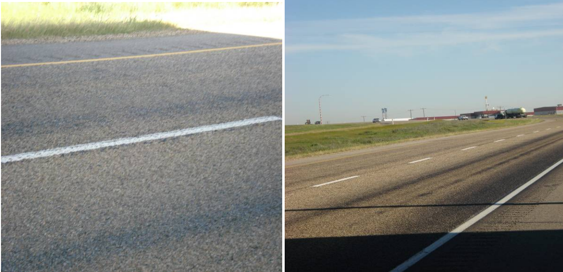
Pathfinder on seal coat (skip lines only)
