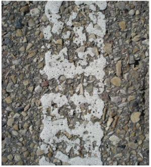
Close-up of the Pathfinder pavement marking, it is estimated that approximately 40% loss of material since 1999.
