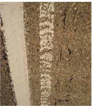
Pathfinder durable wet night marking surface applied adjacent to the west edge line in 1999. Pathfinder is still visible after nine years on this highly travelled roadway.
